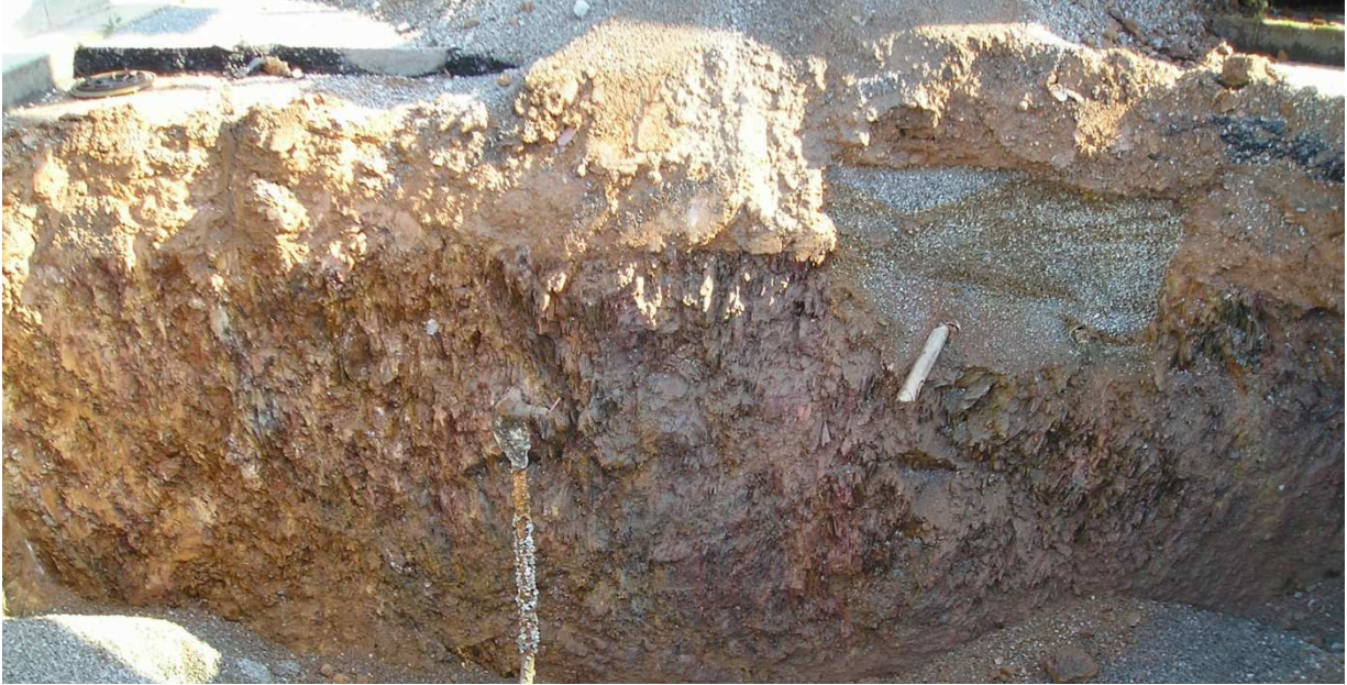
Photograph 1 – Photograph of UST tank field side wall during 2008 removal.
