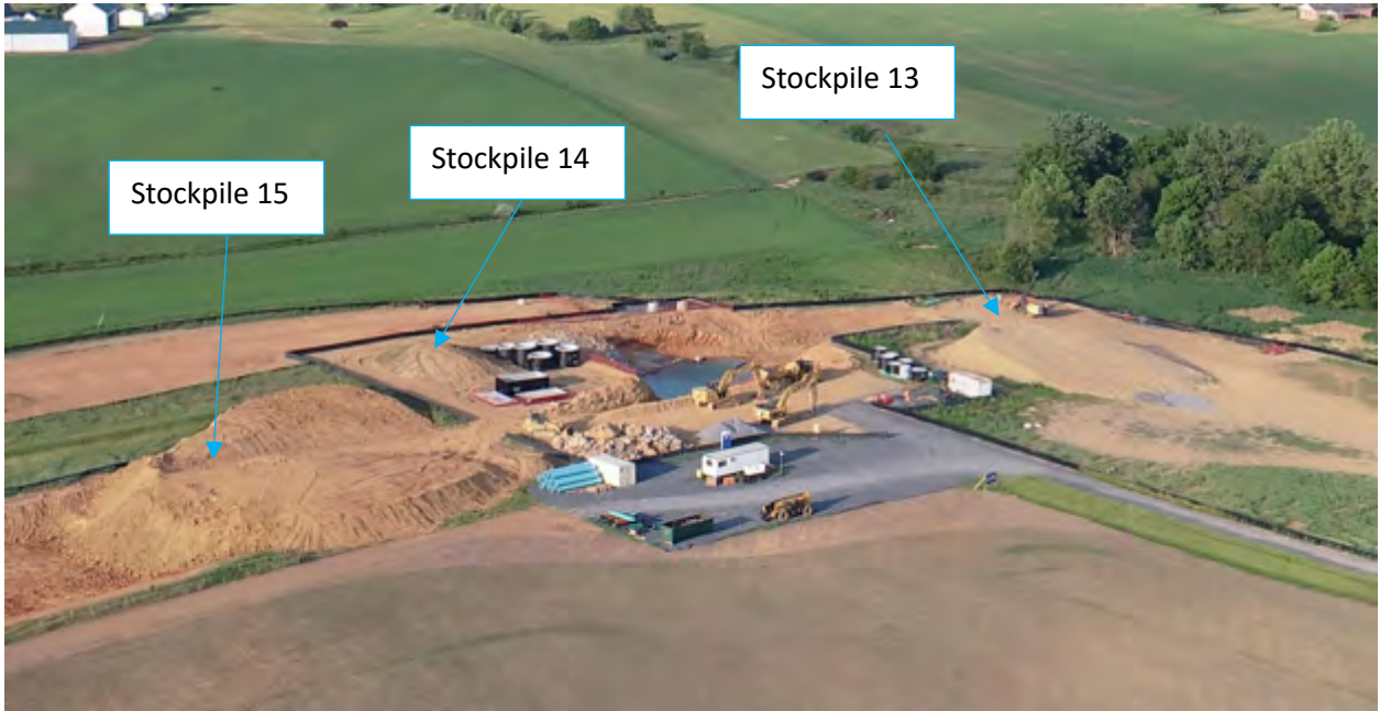
Figure 22: Sewer Pump Station Excavation – 05/30/2023
