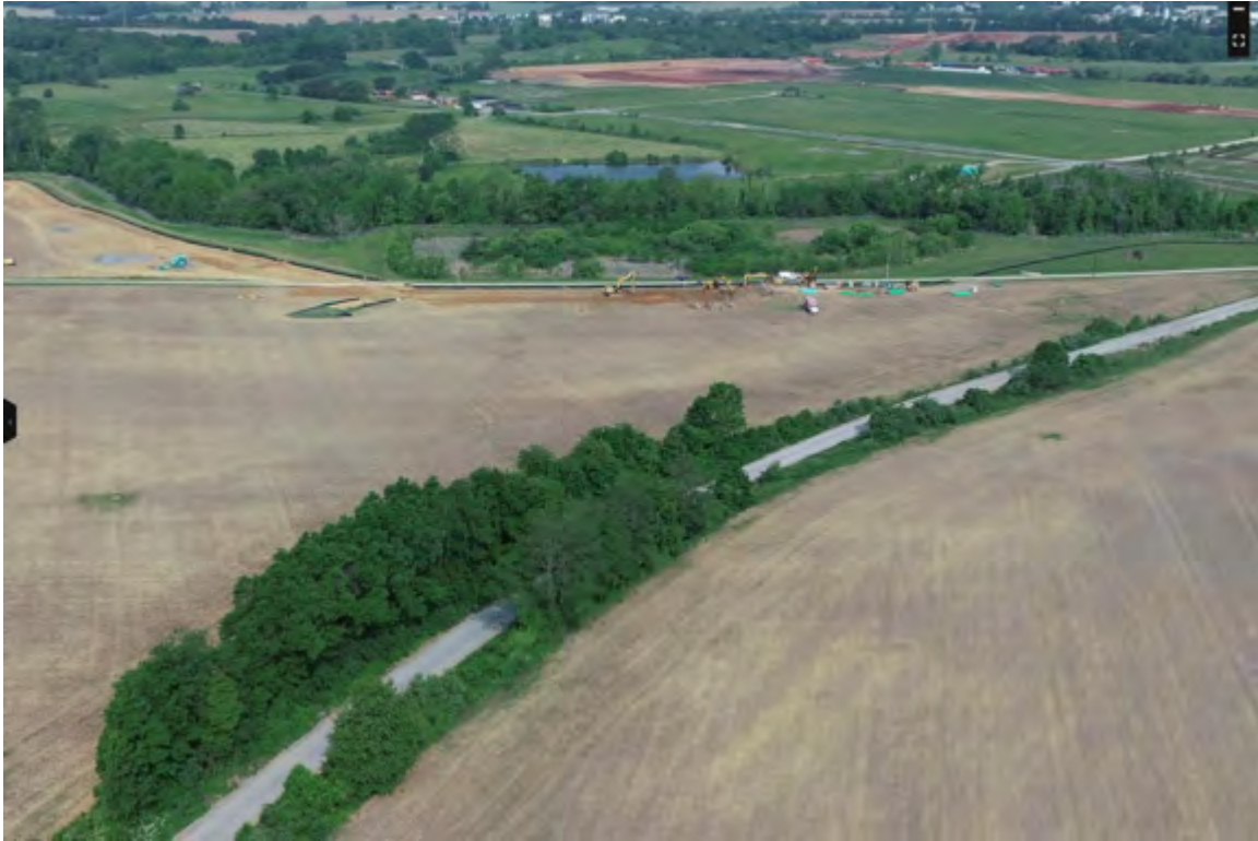
Figure 33: Sewer installation Section A.2 – Week of 05/17/2023
