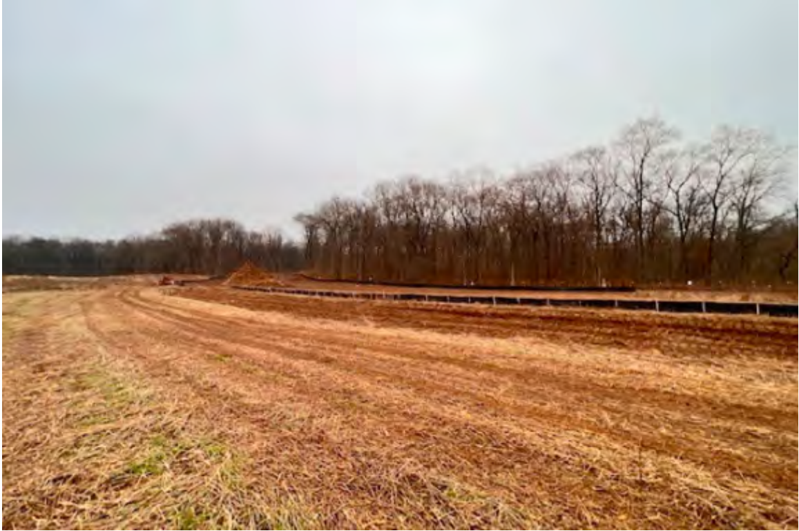
Figure 1: Initial Grading activities along Happy Landing Road from week of 12/09/2022
