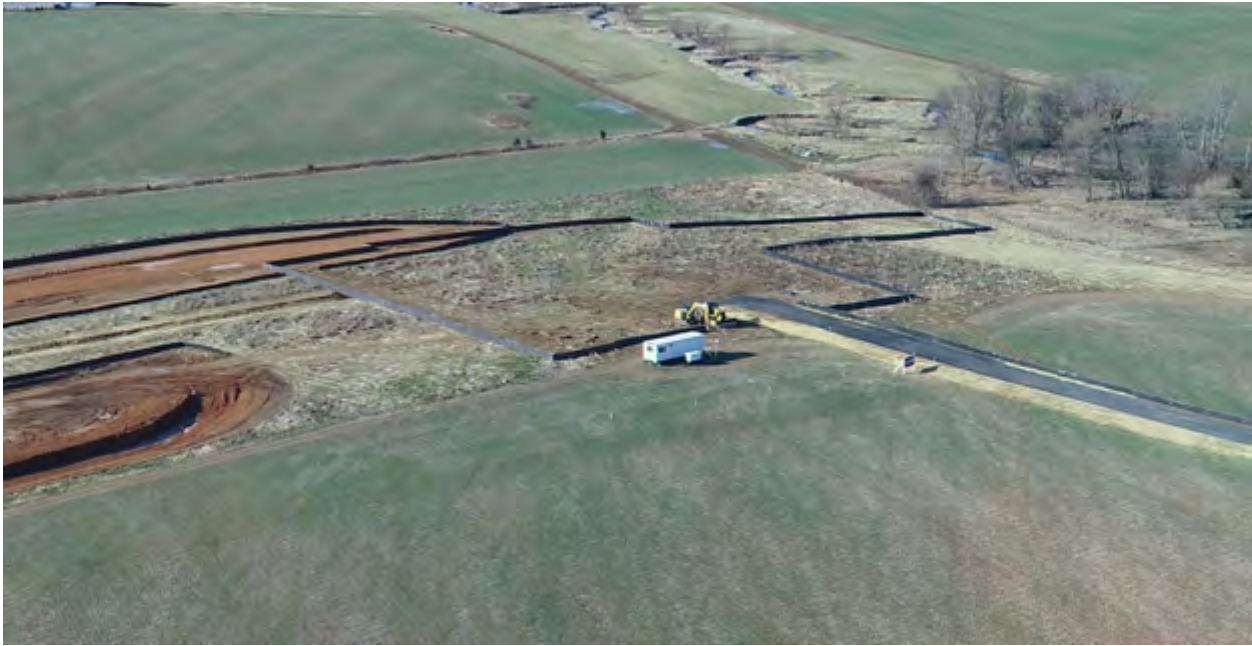
Figure 16: Sewer Pump Station Sediment and Erosion Control Measures – 03/05/2023
