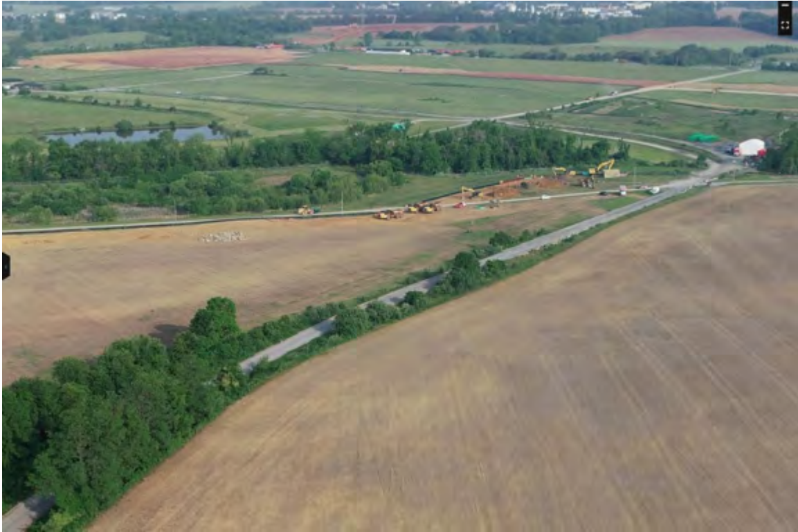
Figure 34: Sewer installation Section A.2 – Week of 05/23/2023
