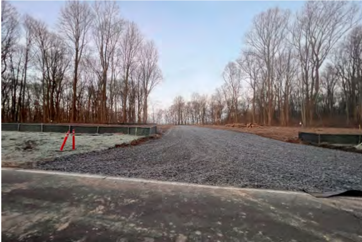
Figure 4: Initial Grading activities along Happy Landing Road from week of 12/23/2022
