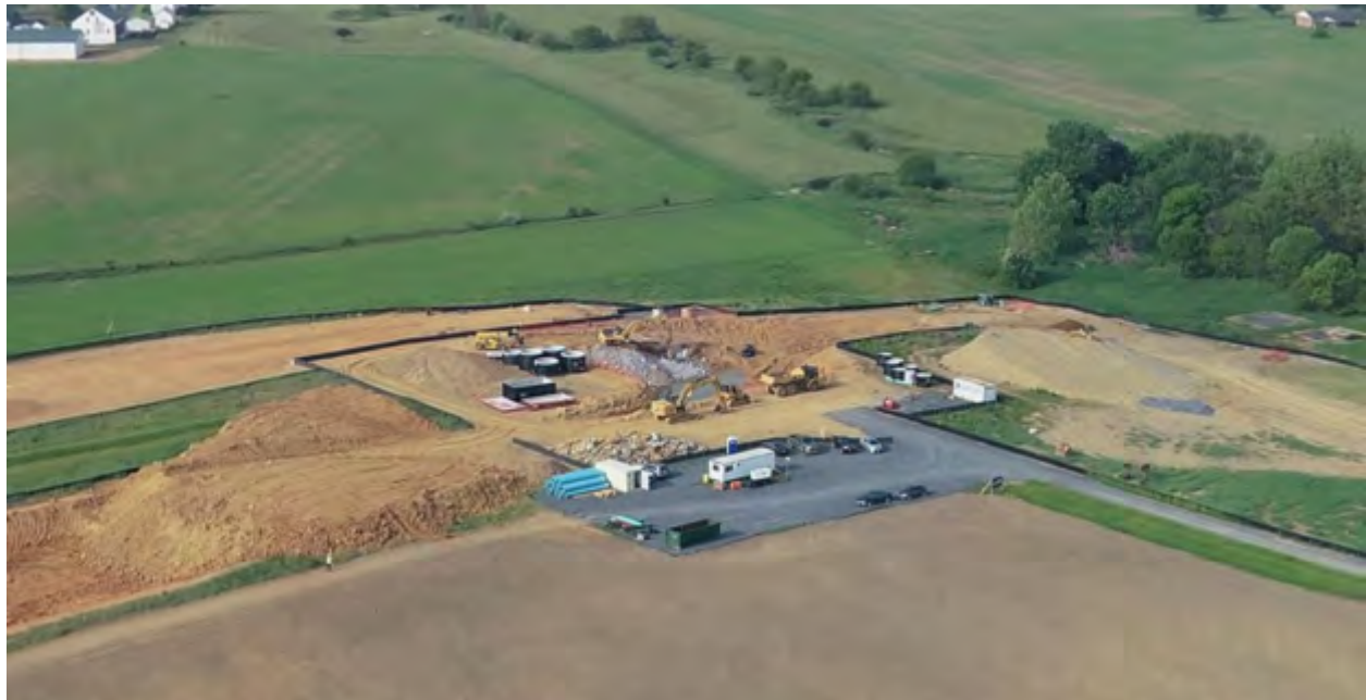
Figure 21: Sewer Pump Station Excavation – 05/23/2023
