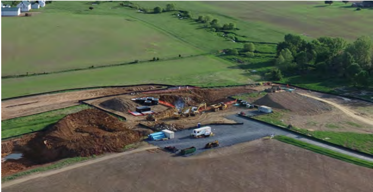
Figure 19: Sewer Pump Station Excavation – 05/10/2023
