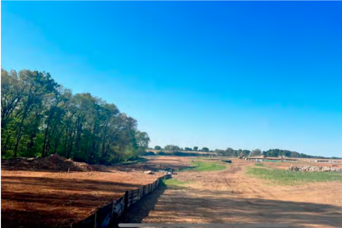
Figure 30: 24" Sewer installation Section A.1 – 04/28/2023
