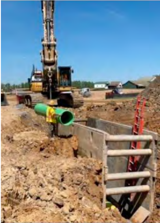
Figure 28: 24" Sewer installation Section A.1 – Week of 04/25/2023
