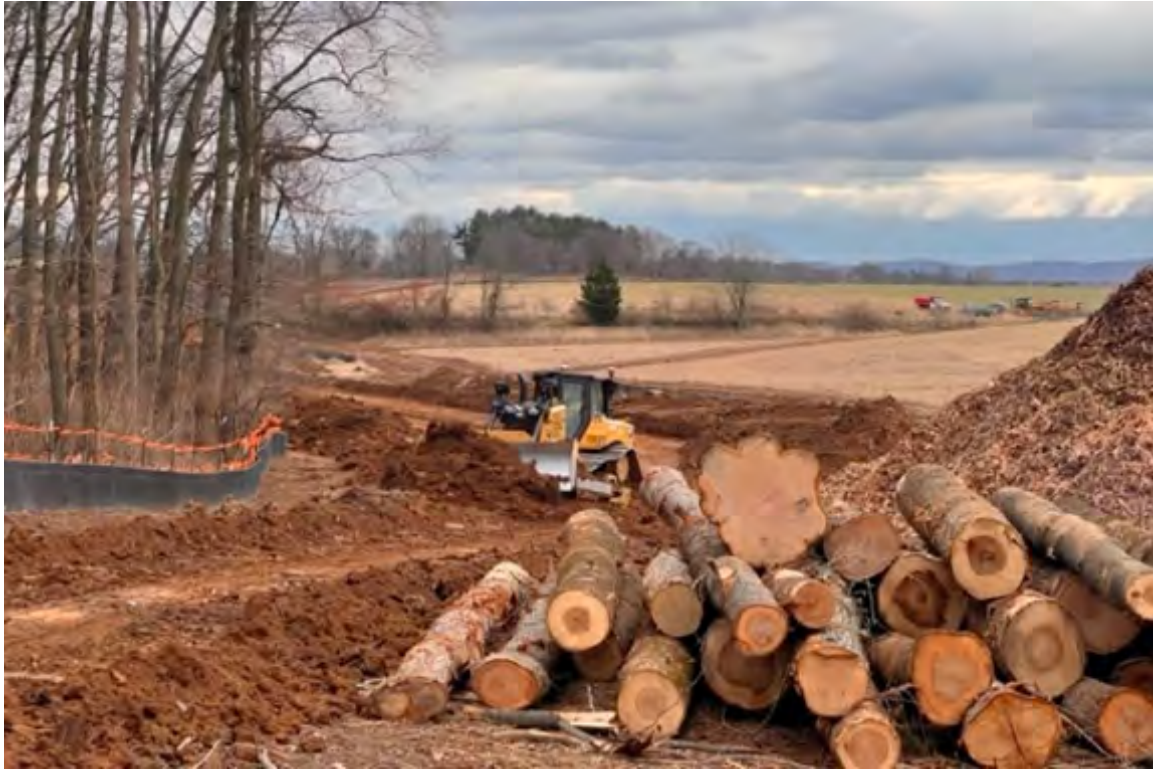
Figure 3: Initial Grading activities along Happy Landing Road from week of 12/16/2022
