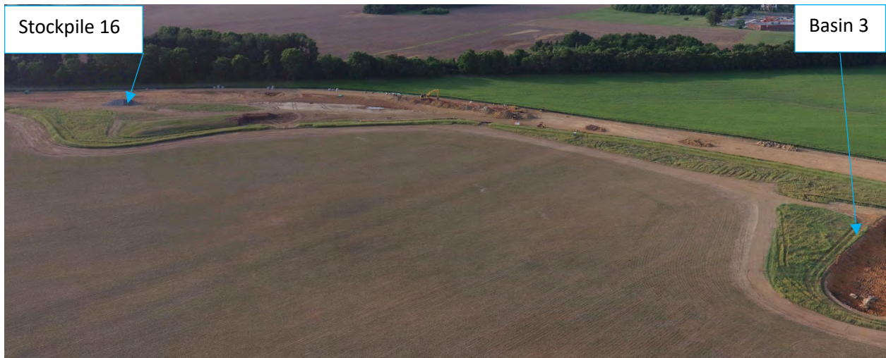
Figure 15: Happy Landing Road - Stockpile 16 - 05/30/2023
