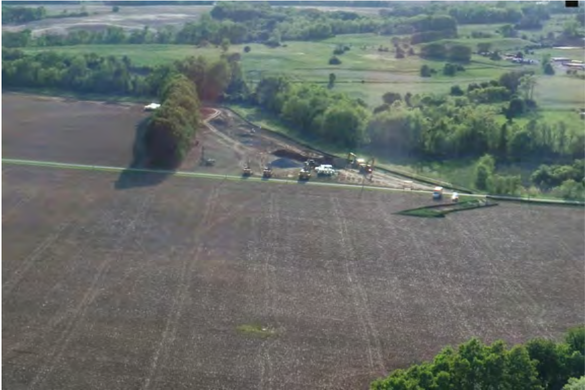
Figure 32: Sewer installation Section A.1 – Week of 05/10/2023
