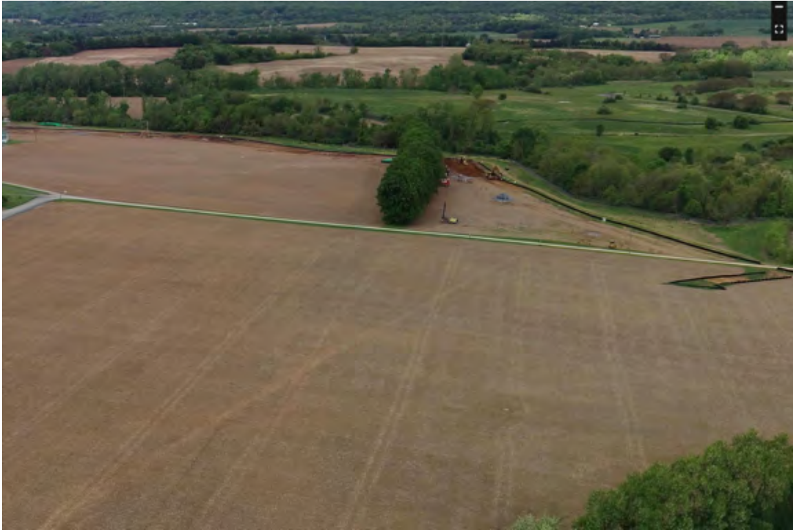
Figure 31: Sewer installation Section A.1 – Week of 05/04/2023
