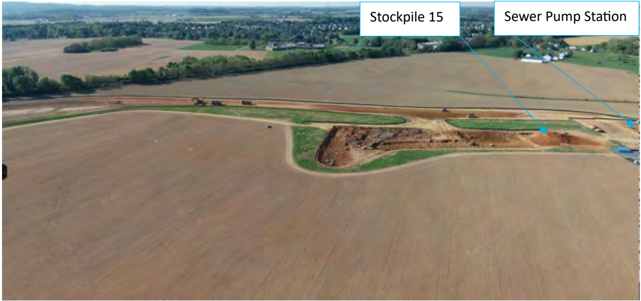
Figure 12: Happy Landing Road – Basin 3 – 04/25/2023
