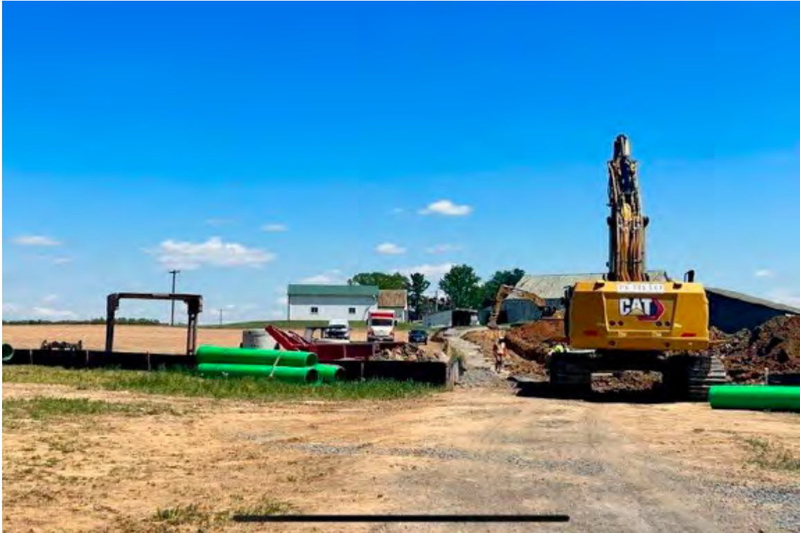
Figure 29: 24" Sewer installation Section A.1 – 04/28/2023
