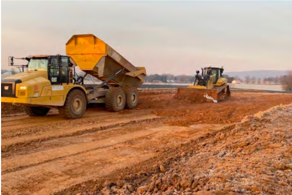
Figure 5: Initial Grading activities along Happy Landing Road from week of 01/13/2023
