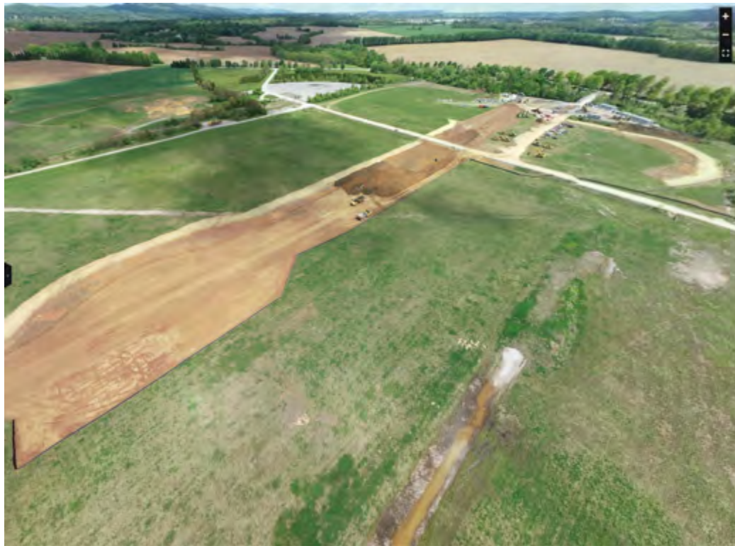
Figure 24: Mass Grading for Quantum Place South – Week of 05/04/2023
