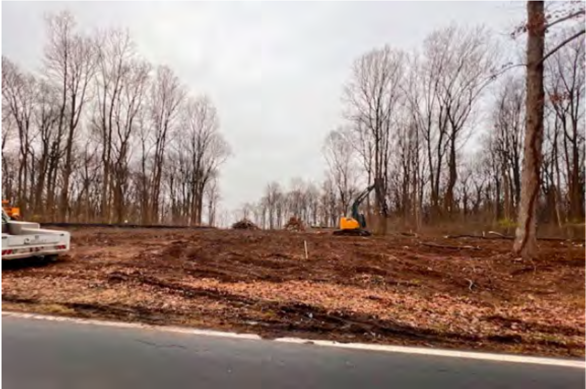
Figure 2: Initial Grading activities along Happy Landing Road from week of 12/16/2022
