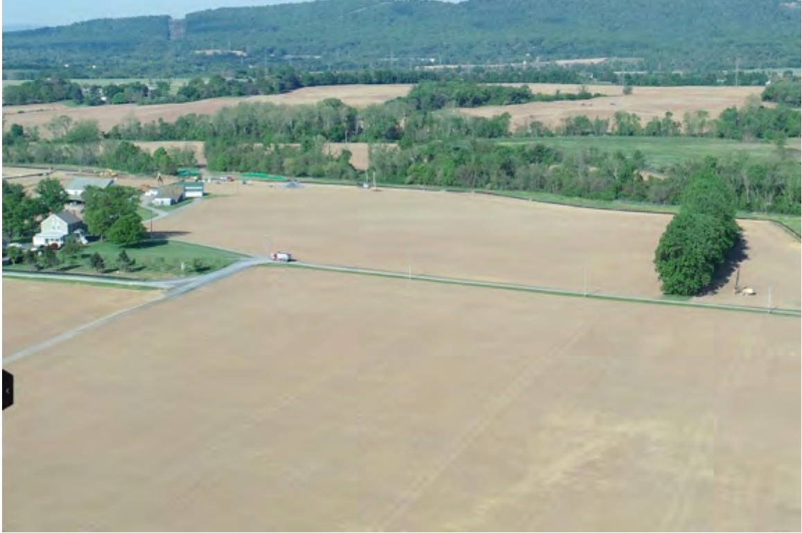
Figure 27: 24" Sewer installation Section A.1 – Week of 04/25/2023
