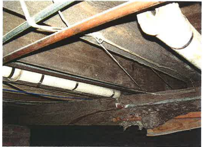
Photo 8. Pipe insulation in crawl space beneath office. The insulation likely contains friable asbestos.
