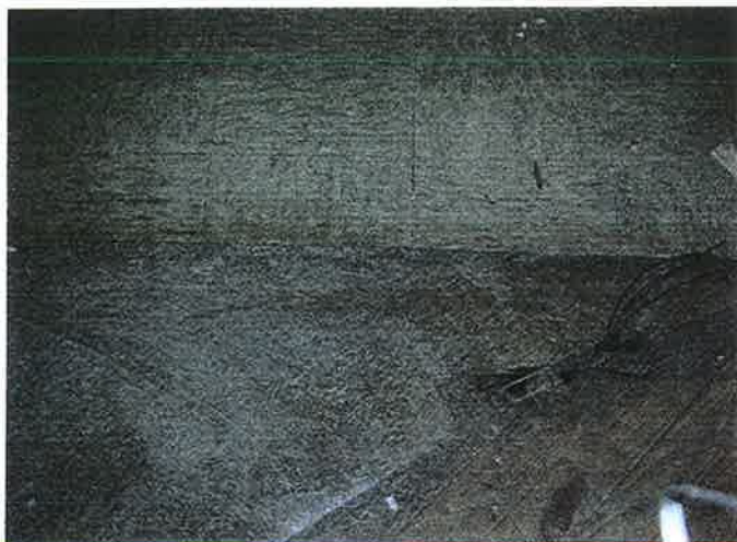
Photo 11. Two layers of floor tiles in office. They may contain asbestos.
