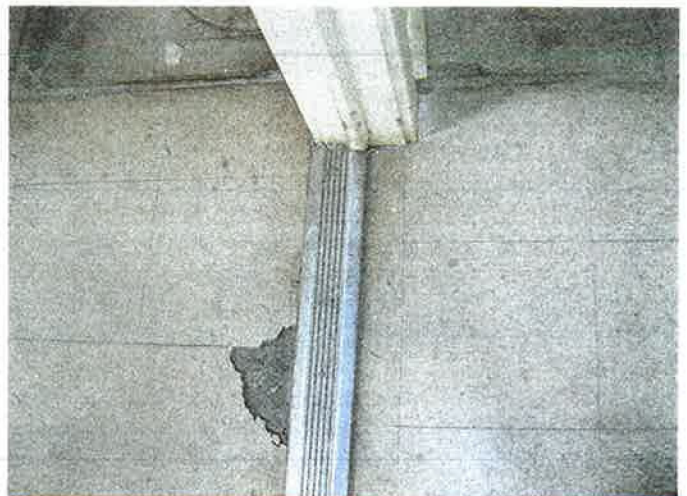
Photo 12. Floor tiles in office building. They may contain asbestos.
