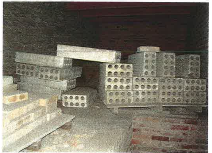
Photo 18. Pyrobar blocks in basement of warehouse. The blocks may contain asbestos.
