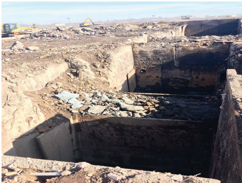
Photograph 4 North and East sides
