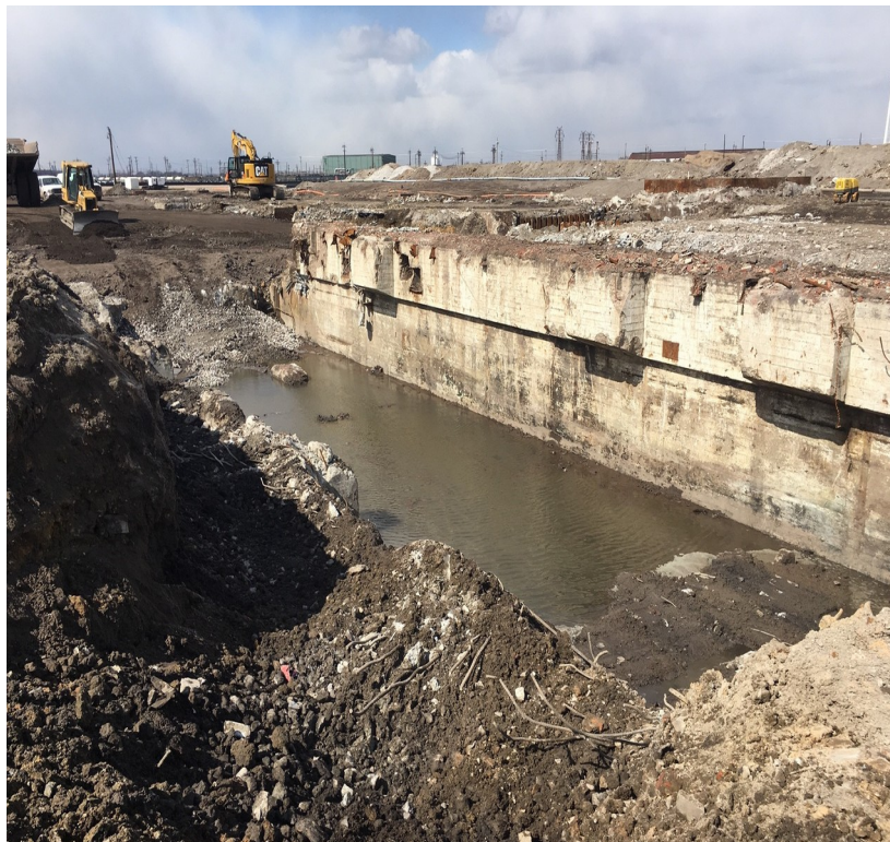
Photograph 2 West & North sides
