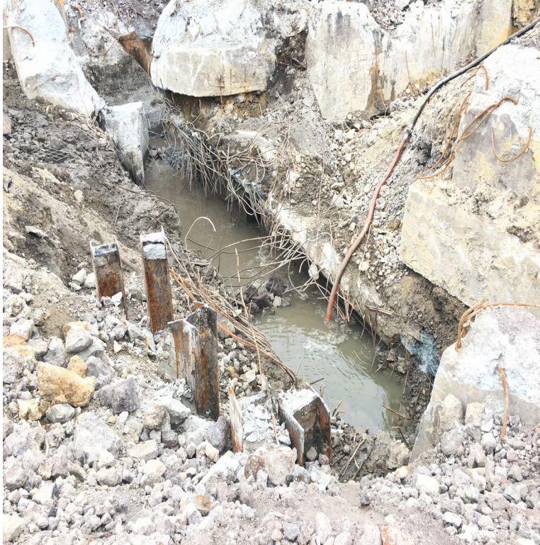
Photograph 3 North arm – North, East, & South sides
