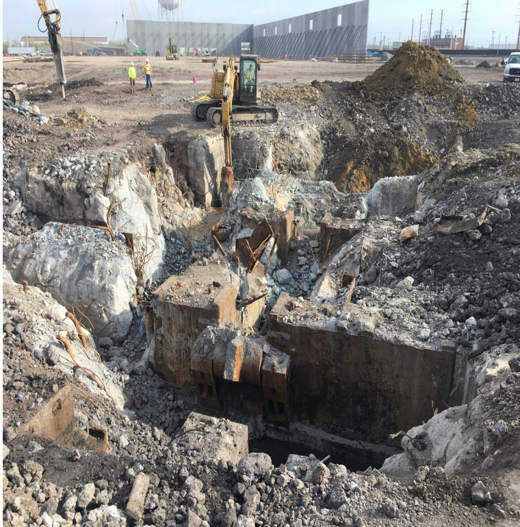
Photograph 1 North & East sides
