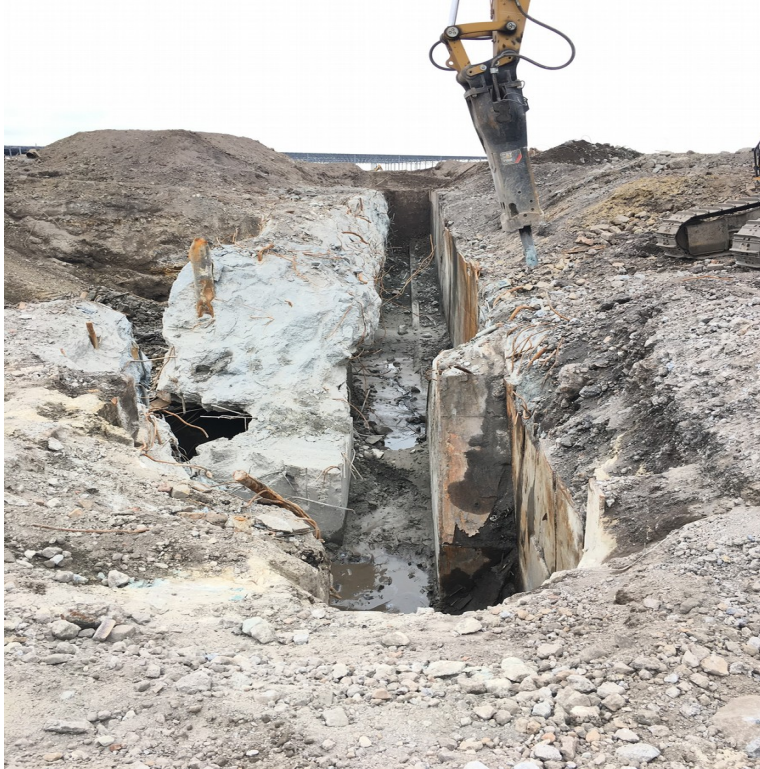
Photograph 1 South arm – North, East, & South sides
