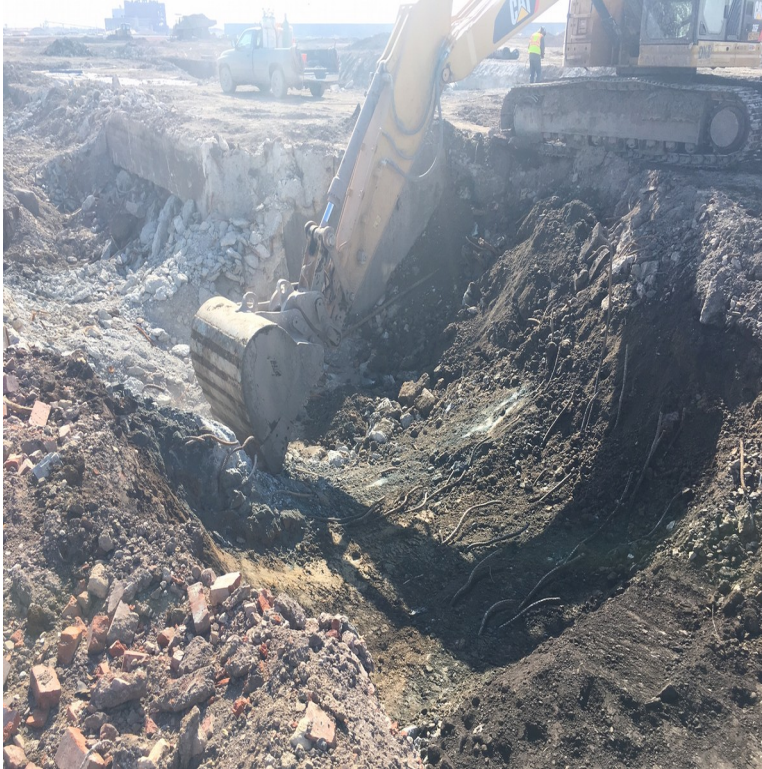
Photograph 1 East & South sides
