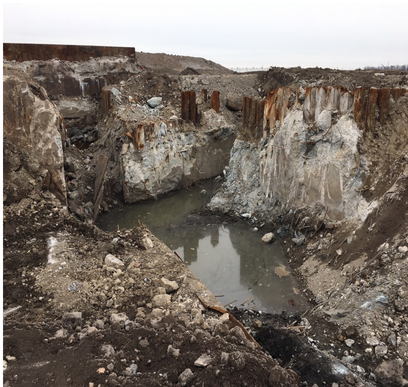
Photograph 2 North & East sides
