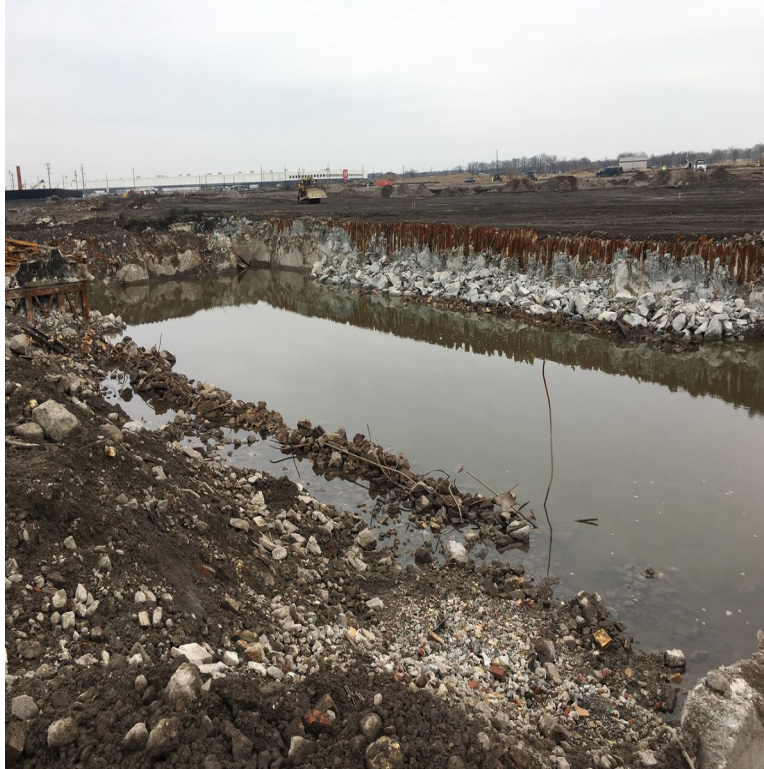
Photograph 4 North & West sides
