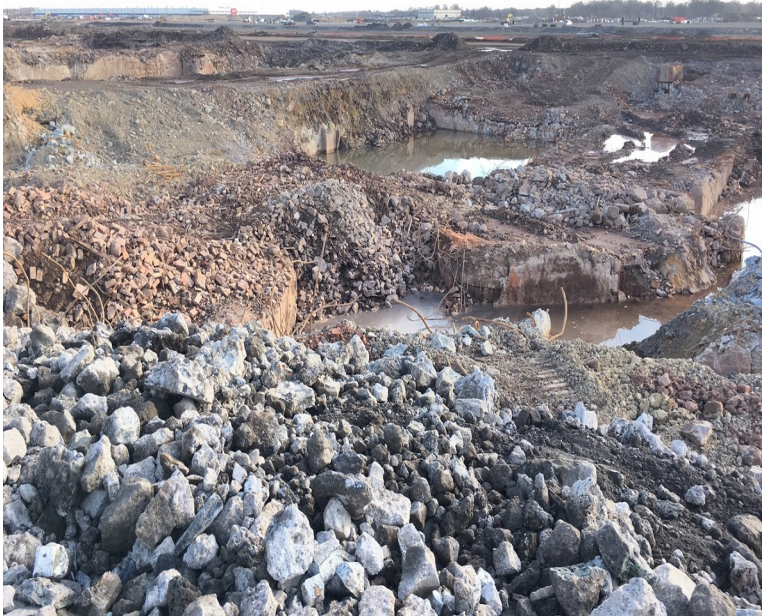
Photograph 5 North & East sides
