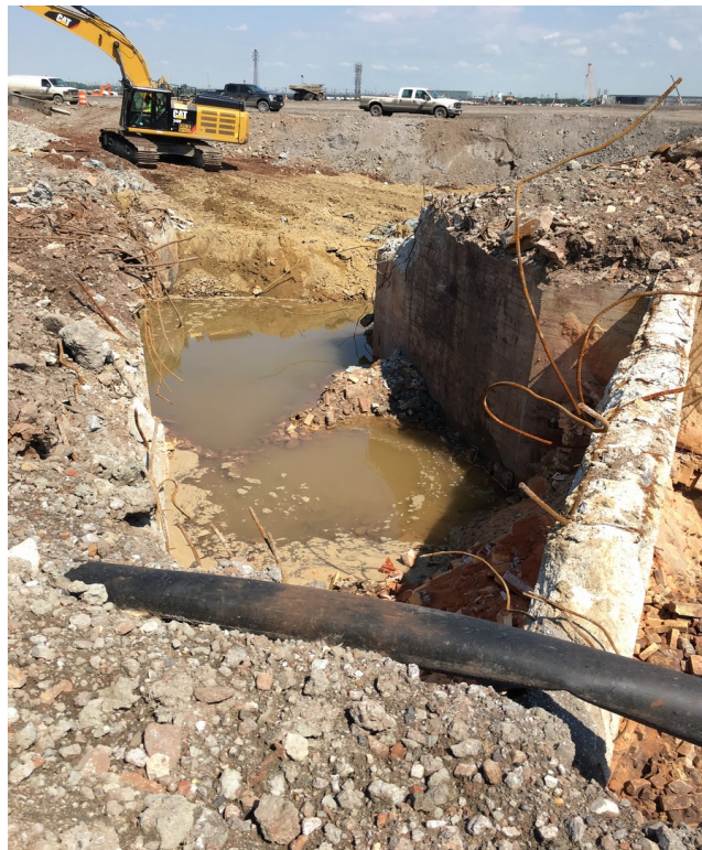
Photograph 4 West side & Middle
