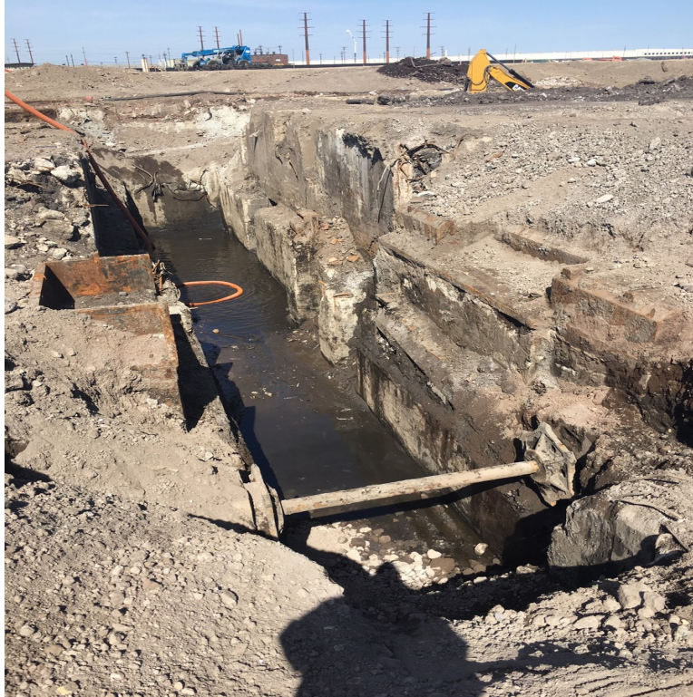
Photograph 3 North & East sides
