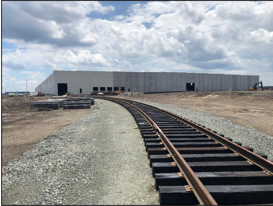
Photo 9: Rail line and building exterior
