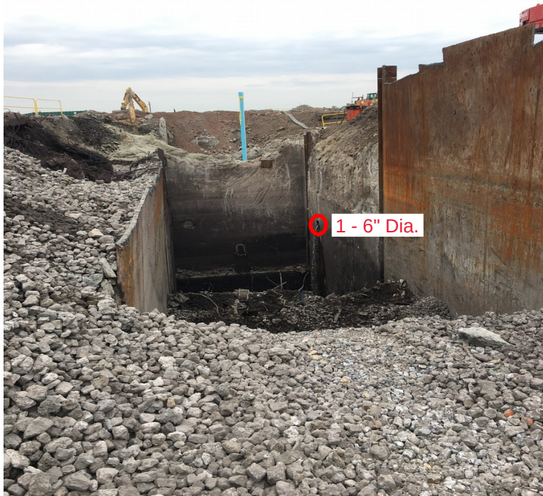
Photograph 1 South, West, & North sides
