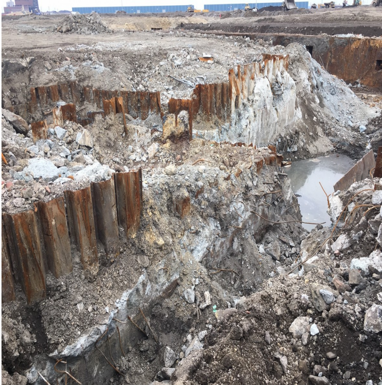
Photograph 1 East & South sides
