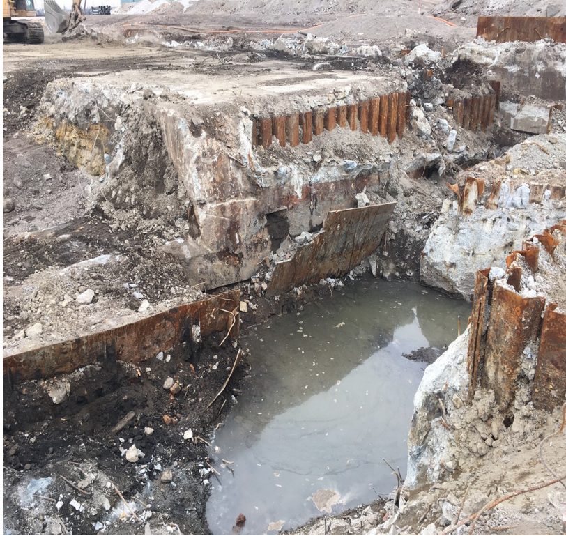
Photograph 3 West & North sides
