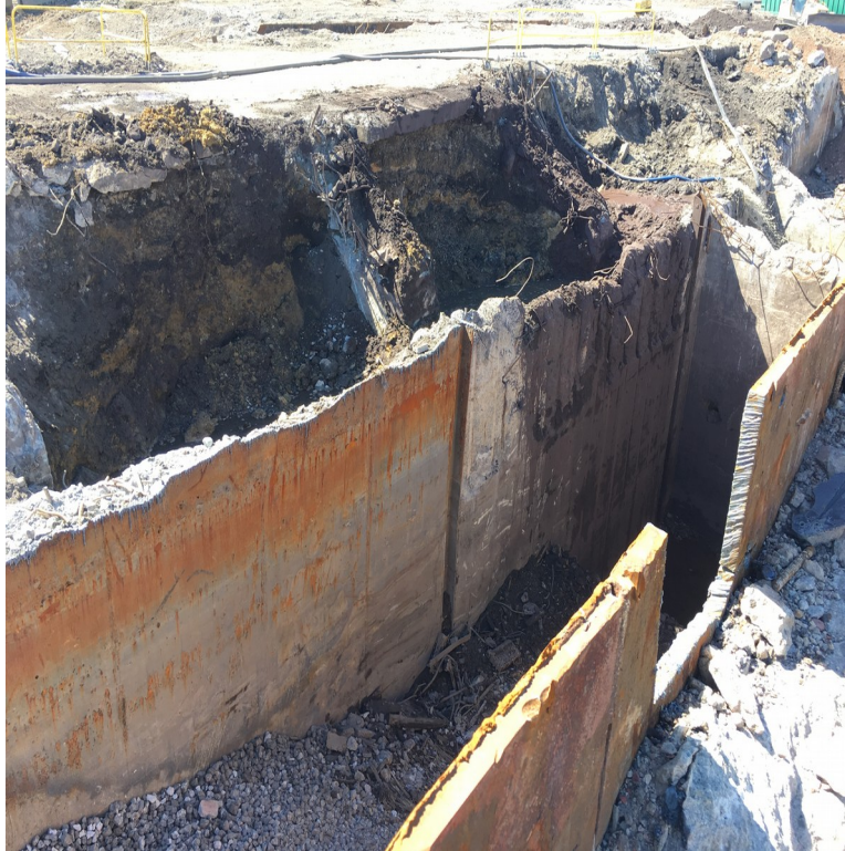
Photograph 3 South & West sides
