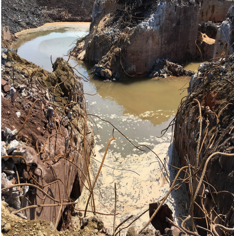
Photograph 5 North side & Middle
