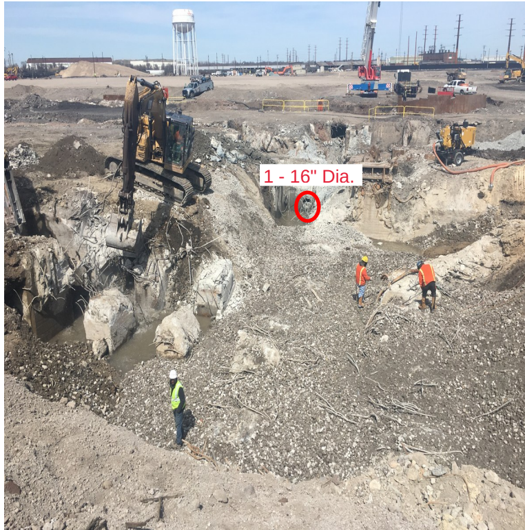
Photograph 1 West & North sides
