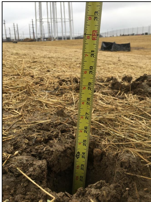
Photo 8: Thickness of clean fill on landscape area
