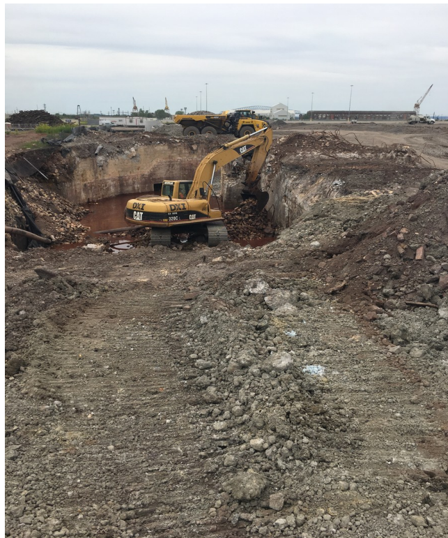
Photograph 6 South & West sides
