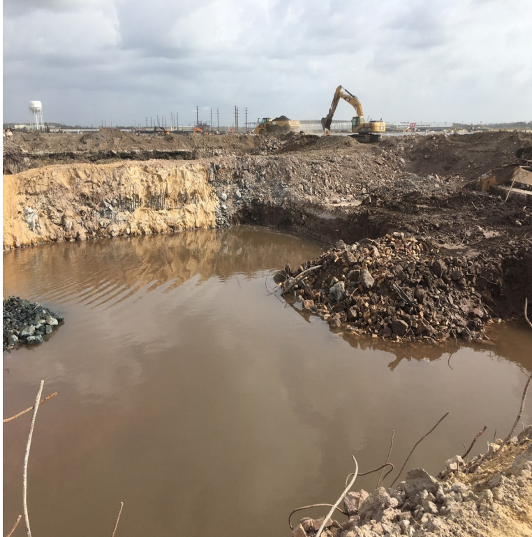
Photograph 5 North & East sides
