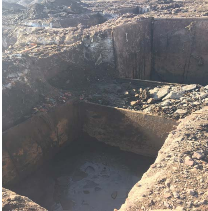
Photograph 5 South and West sides
