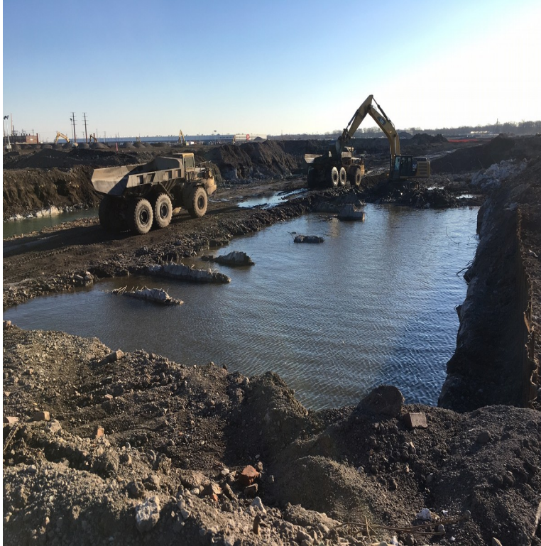
Photograph 3 North & East sides
