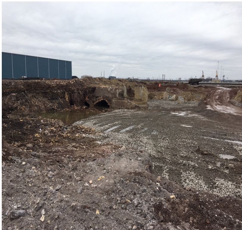
Photograph 2 South & West sides
