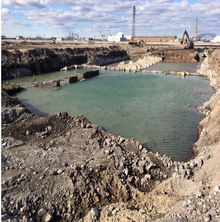
Photograph 1 South & West sides
