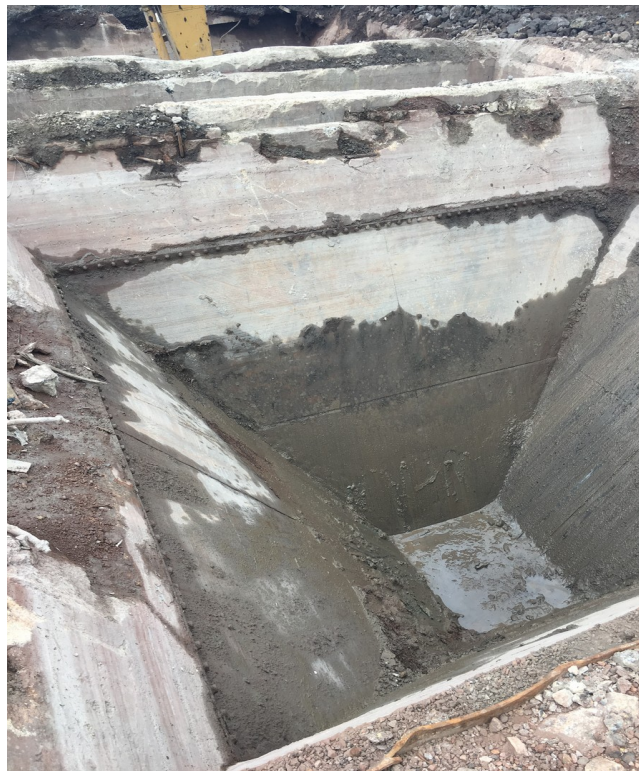
Photograph 2 Inside of East chute
