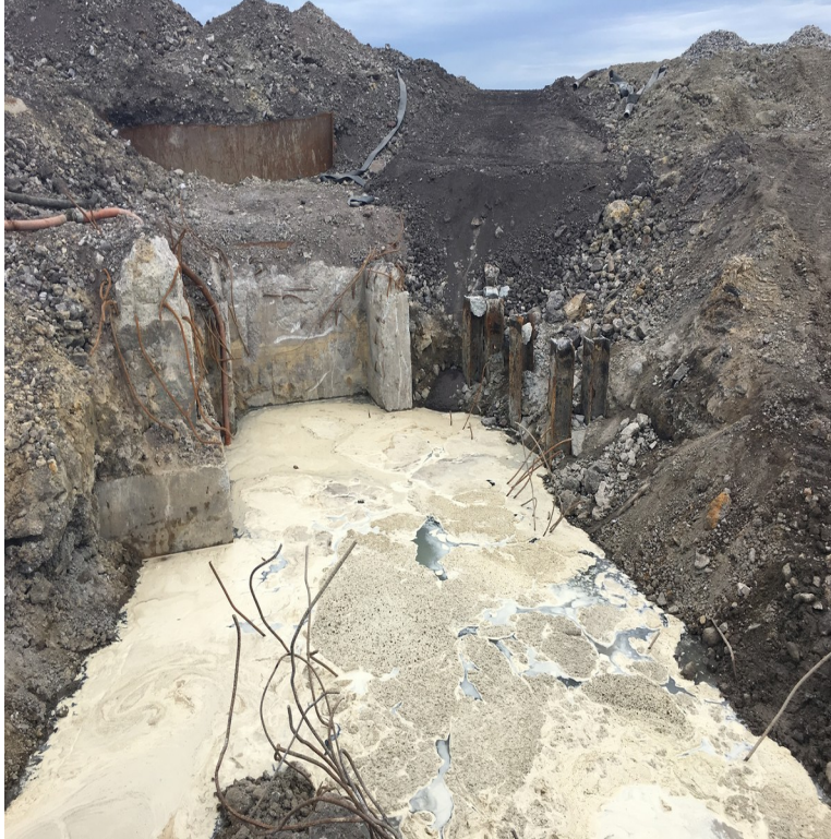
Photograph 5 North arm – West & North sides
