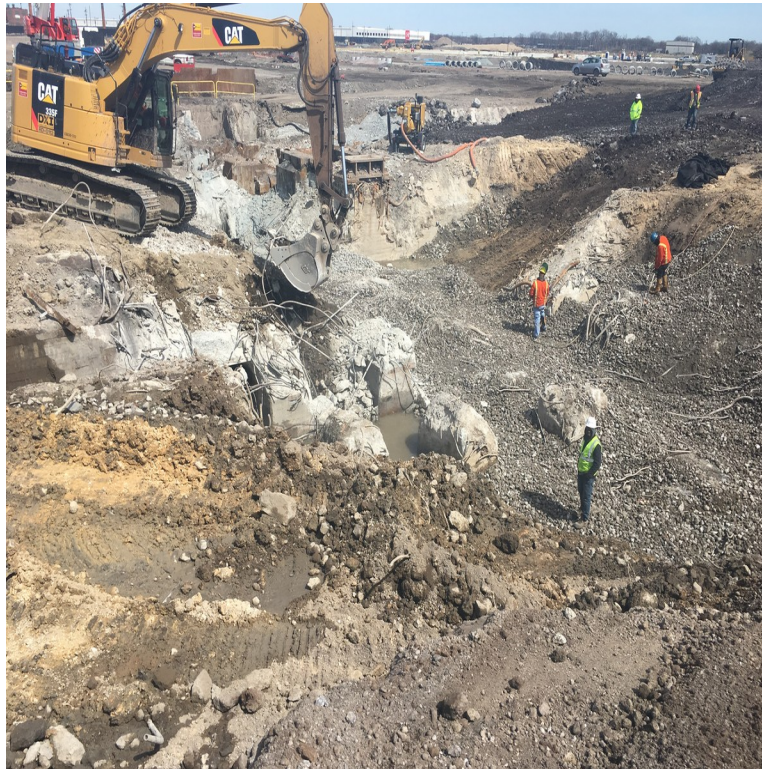
Photograph 2 North & East sides
