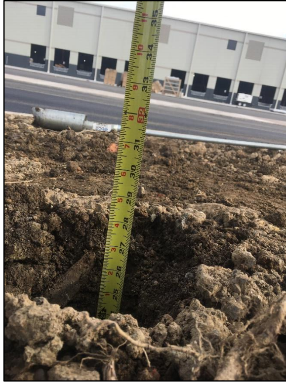
Photo 7: Thickness of clean fill on landscape area
