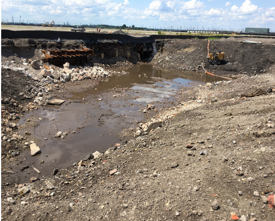
Photograph 1 West & North sides
