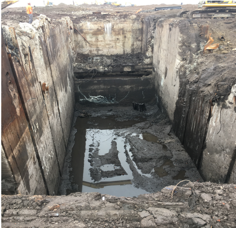
Photograph 3 South, West, & North sides
