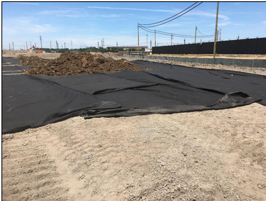
Photo 6: Placement of fabric and clean fill in basin
