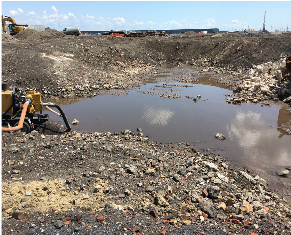
Photograph 2 East & South sides
