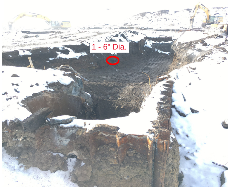
Photograph 1 East & South sides
