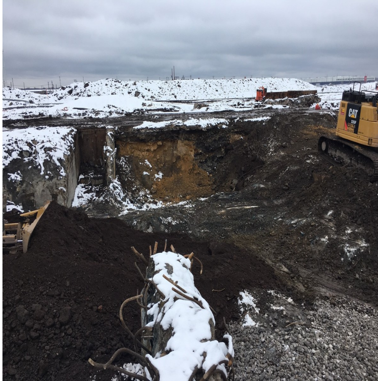
Photograph 1 North & East sides
