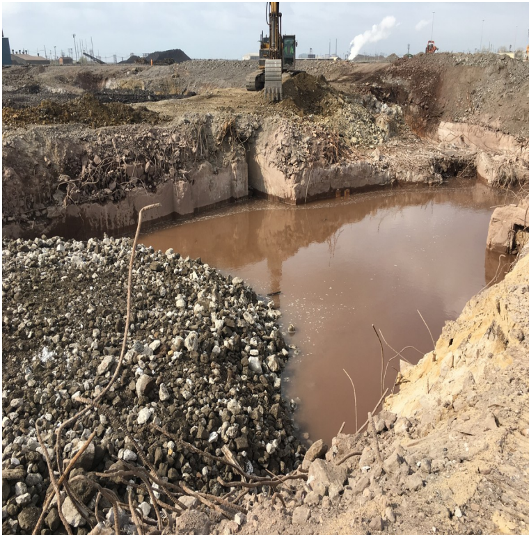
Photograph 2 South & West sides
