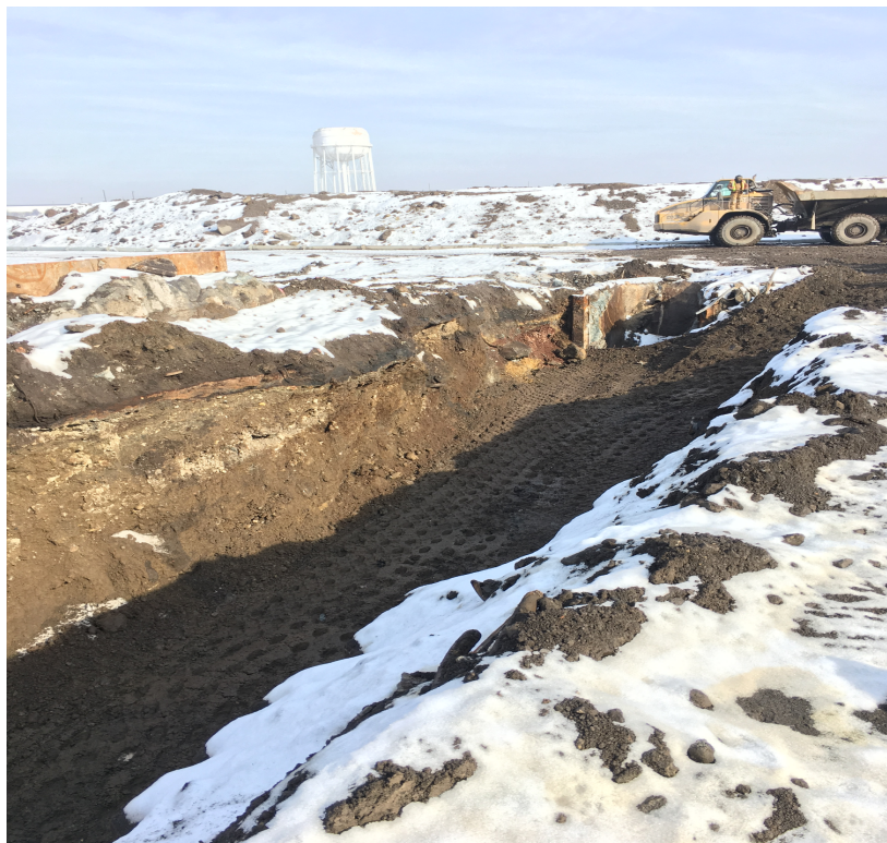
Photograph 2 West & North sides
