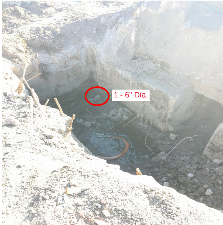
Photograph 1 North & East sides
