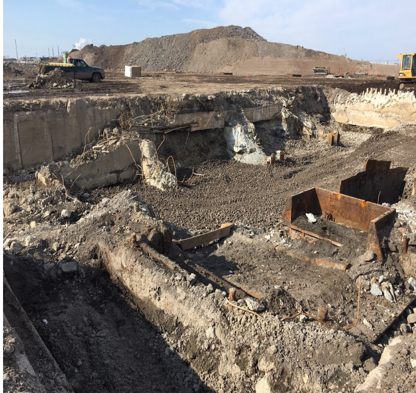
Photograph 3 South & West sides
