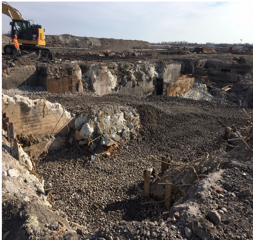
Photograph 2 North & East sides
