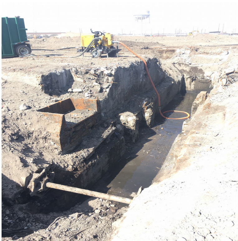
Photograph 4 West & North sides
