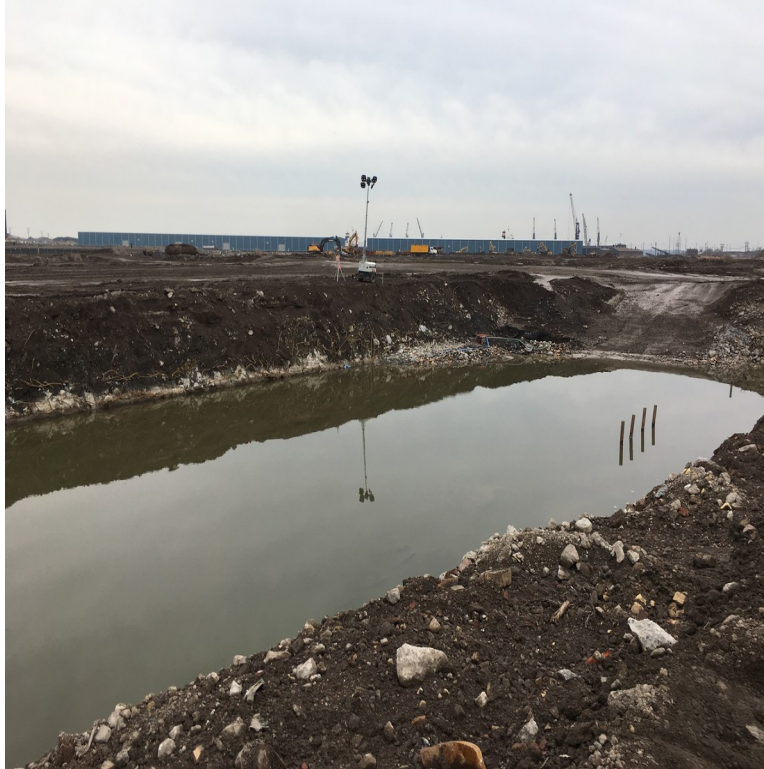
Photograph 3 East & South sides
