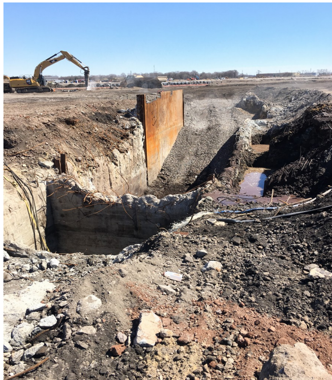
Photograph 2 North & East sides
