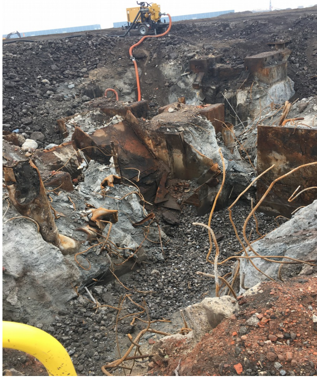
Photograph 3 East & South sides
