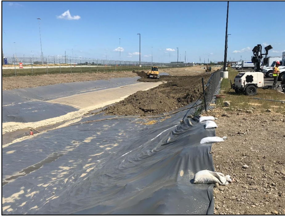
Photo 5: Placement of fabric and clean fill in basin
