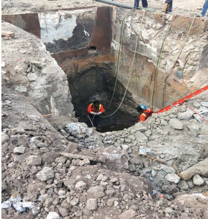
Photograph 7 West and North sides
