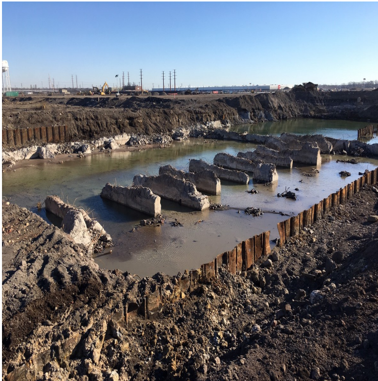
Photograph 2 North & East sides
