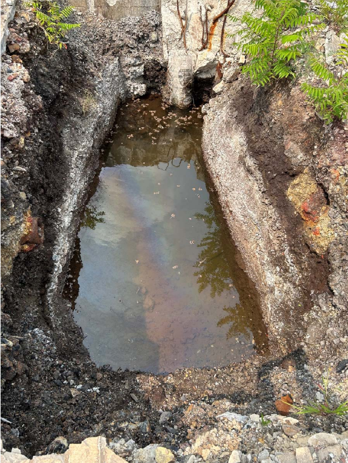
TP-D (former SW-026D-MWS): Top view of test pit interior.
