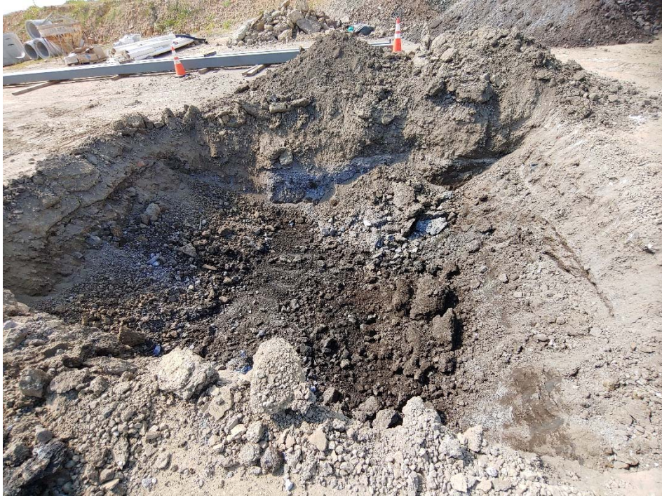
Photo 6: Excavation Area A11-024V-SB
