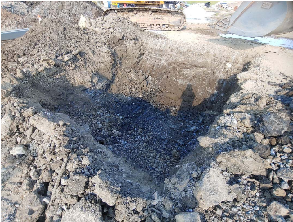
Photo 5: Excavation Area A11-024V-SB
