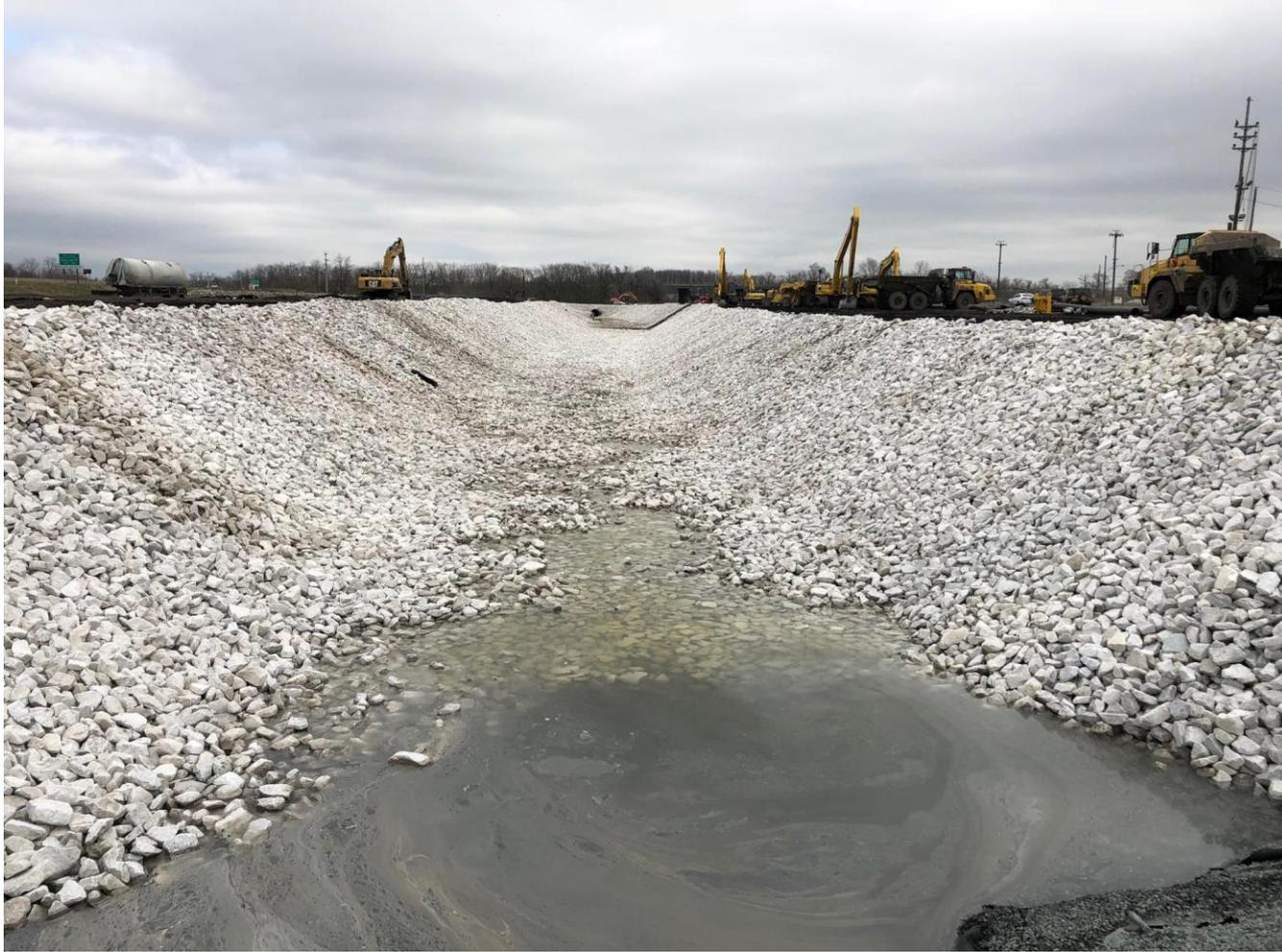
Sections #1 and #2 of Tin Mill Canal Following Placement of Rip- Rap
