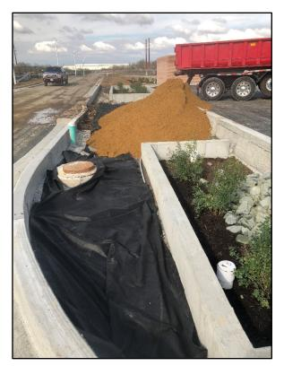
Photo 10: Placement of marker fabric and clean fill
