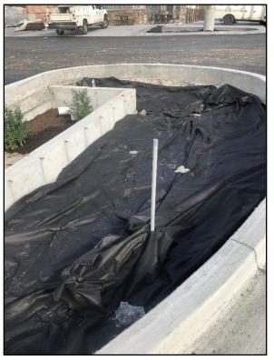
Photo 7: Placement of marker fabric
