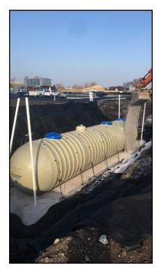
Photo 5: Underground Storage Tank (UST) installation
