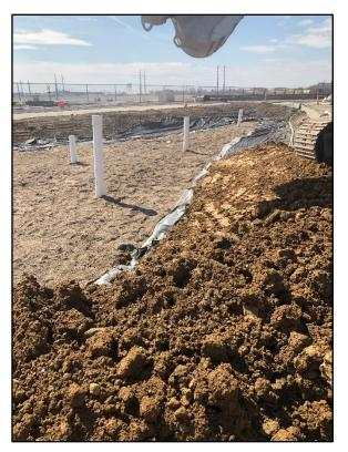
Photo 8: Placement of marker fabric and clean fill
