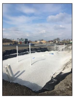
Photo 6: UST excavation backfilling
