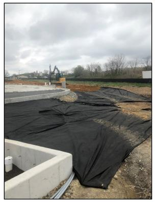
Photo 9: Placement of marker fabric and clean fill
