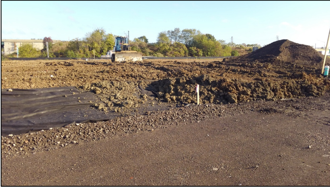
Photo 1: Placement of clean fill and marker fabric
