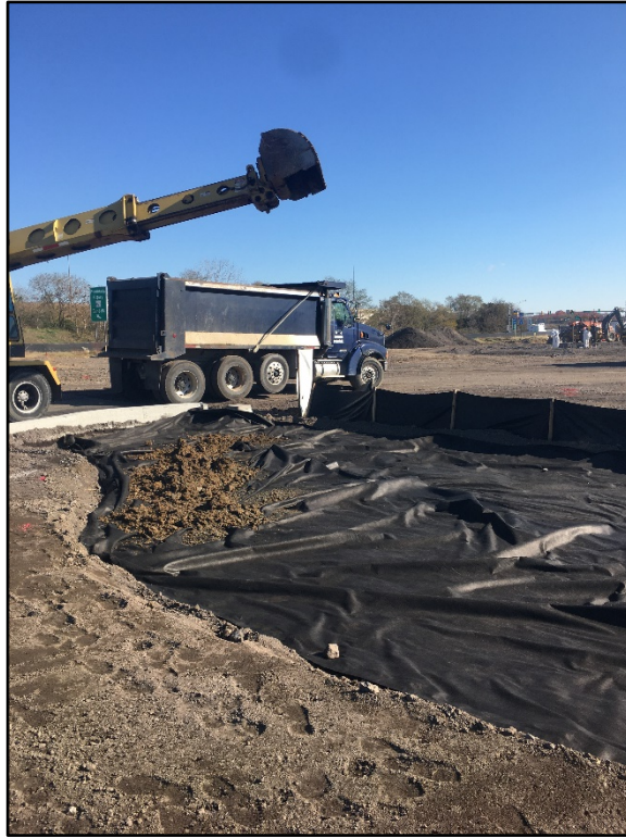
Photo 3: Placement of marker fabric and clean fill
