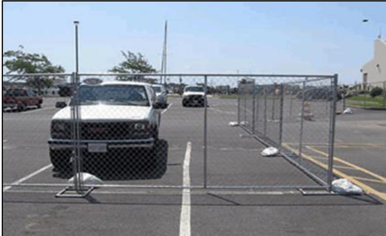
**Non-Ground Intrusive Chain Link Temporary Storm Fencing**
