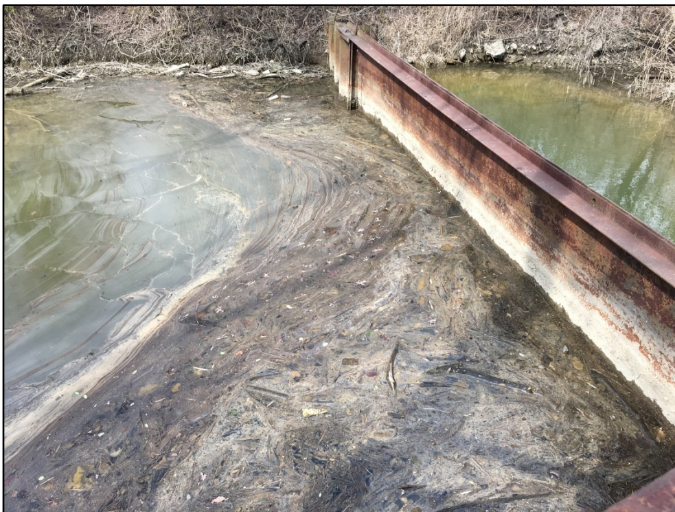
031518-8: View of potential petroleum impacts located at the oil skimming weir.
