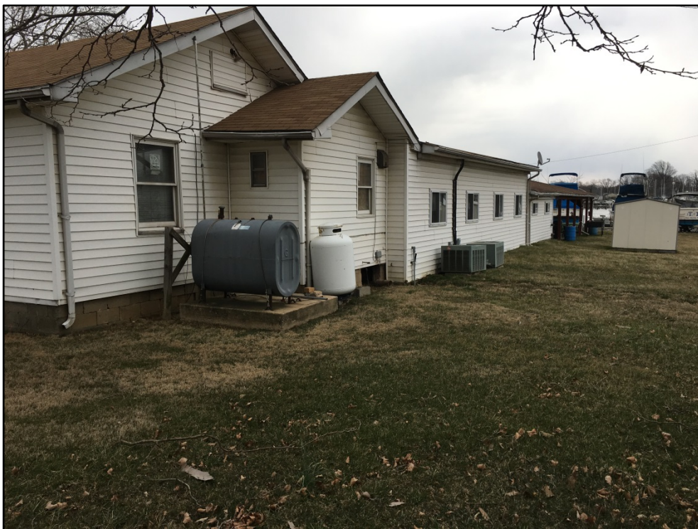
031518-2: View of a heating oil AST located along the southwest corner of the main building.
