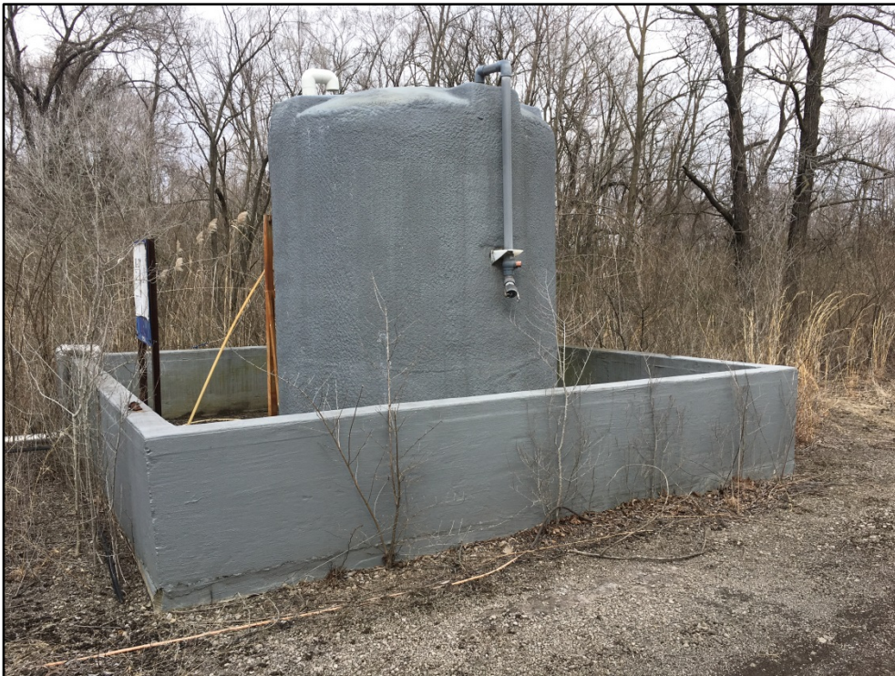
031518-6: View of a sodium bisulfate AST located within secondary containment.
