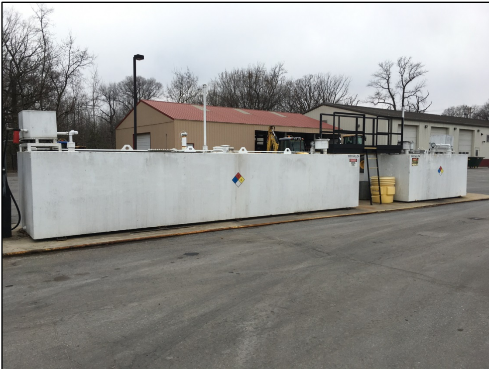
031518-16: View of one 5,000 gallon diesel AST and one 2,000 gallon gasoline AST located along the southern portion of the facility.
