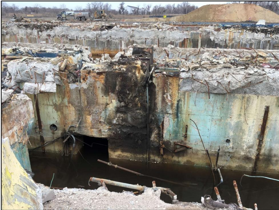
020118-7: Acid staining observed on the concrete in the eastern Halogen Line (No. 1) located on the northern portion of the parcel. Halogen Line No. 2 can be seen in the background.
