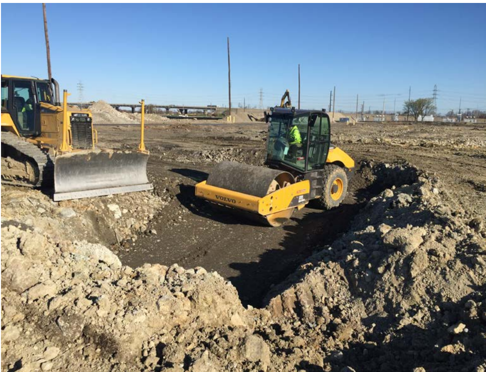
Photo 12: View of backfill compaction activities.
