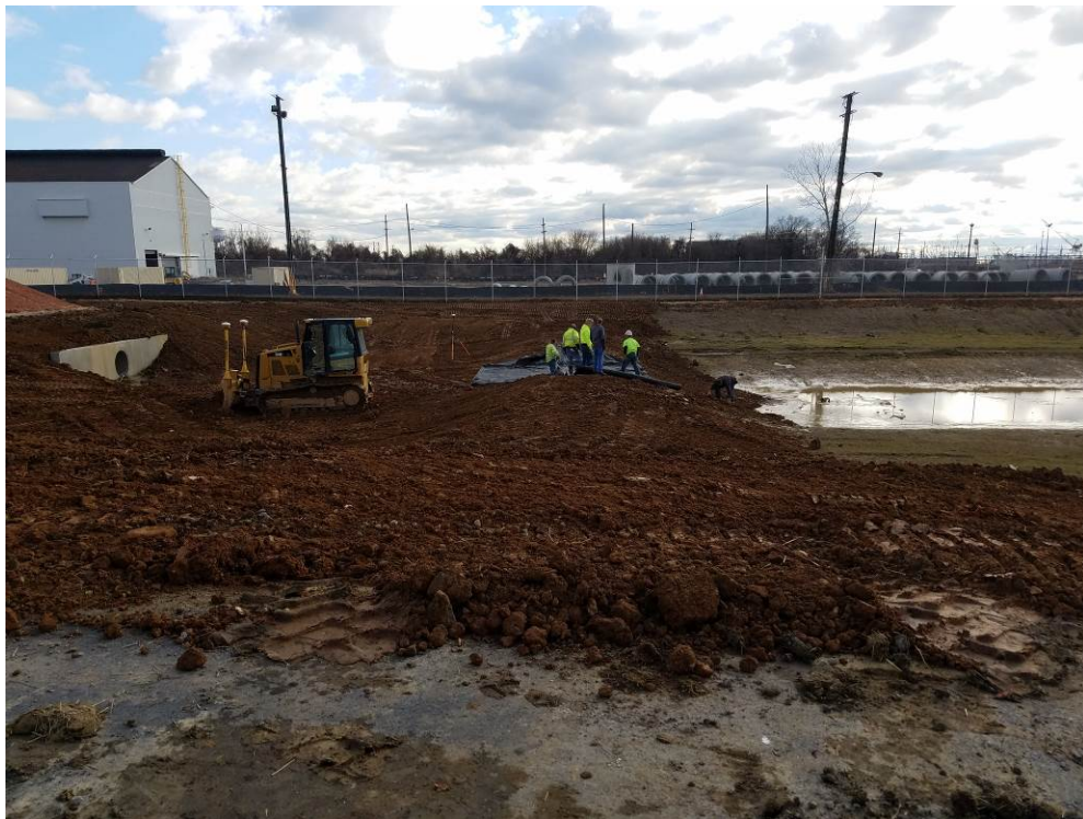
Photo 46: View of workers laying geotextile fabric for SWM facility No. 1.
