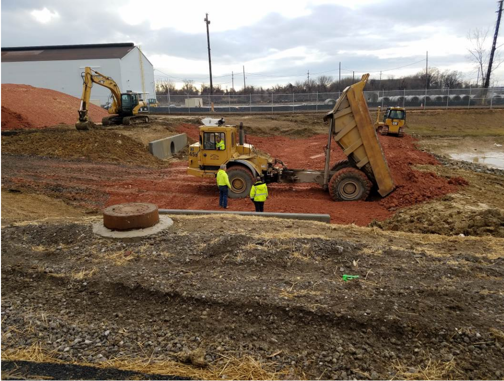
Photo 45: View of construction of storm water management (SWM) facility No. 1.
