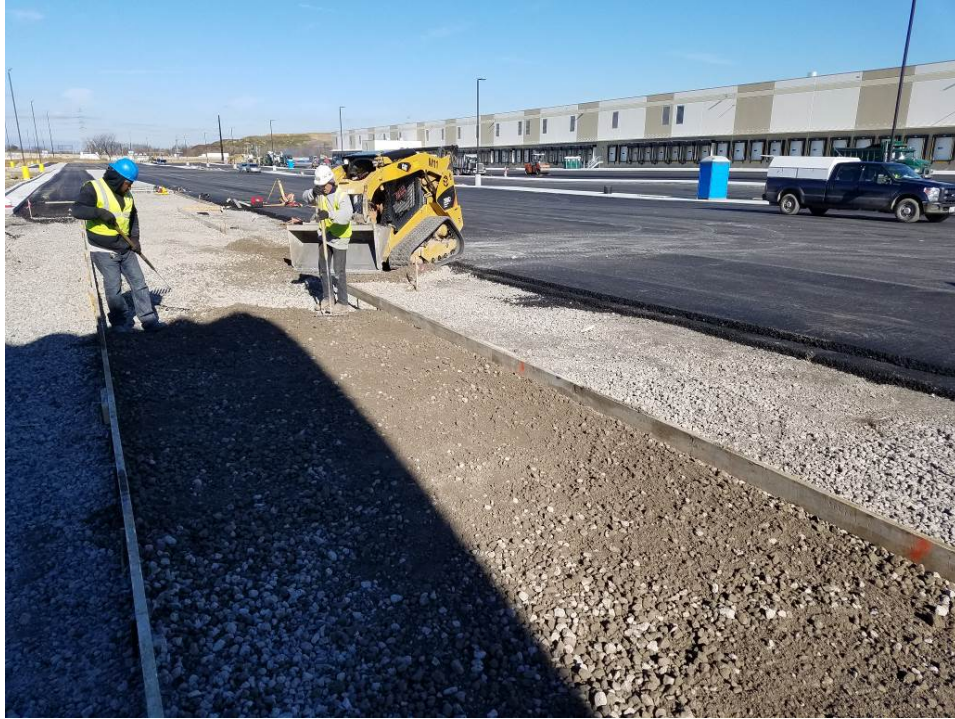
Photo 39: View of road base and asphalt in a hardscape area.
