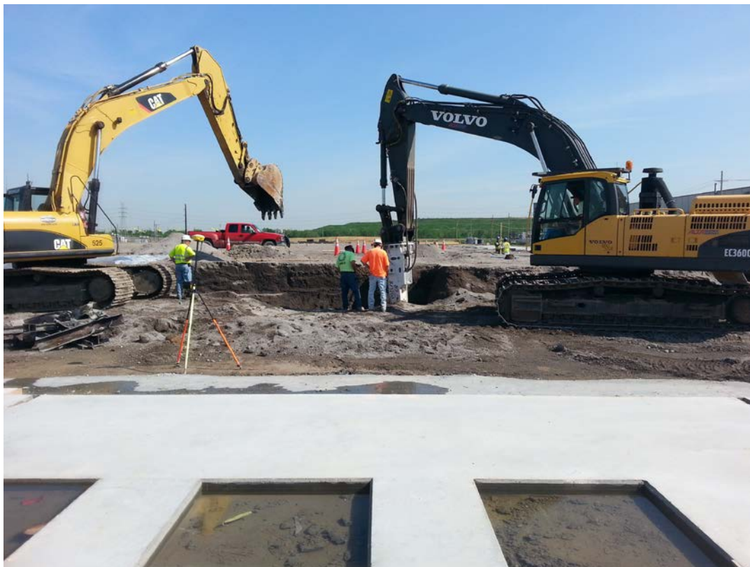
Photo 20: View of excavation activities for main building footers.
