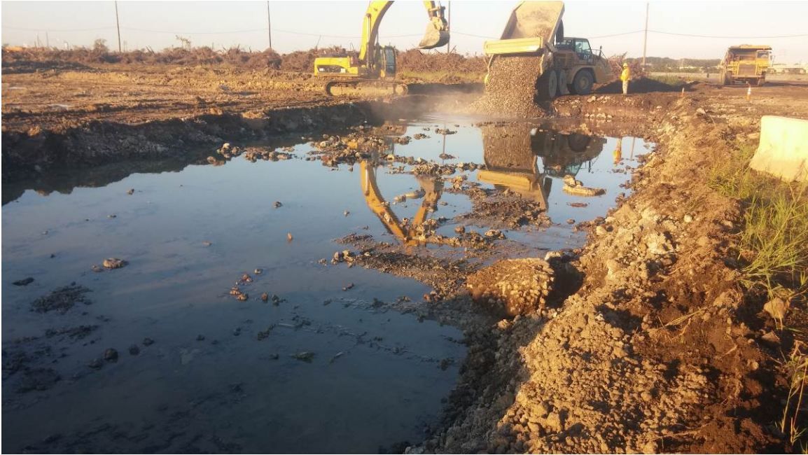
Photo 15: View of backfilling activities for the SP-4 excavation.
