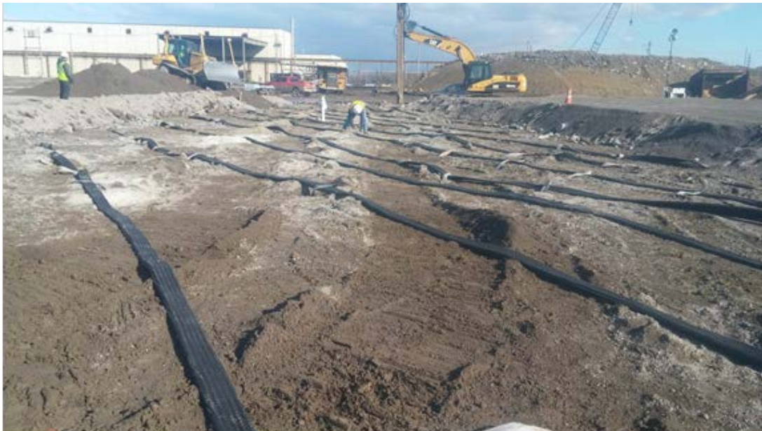
Photo 18: View of the wick drain installation.
