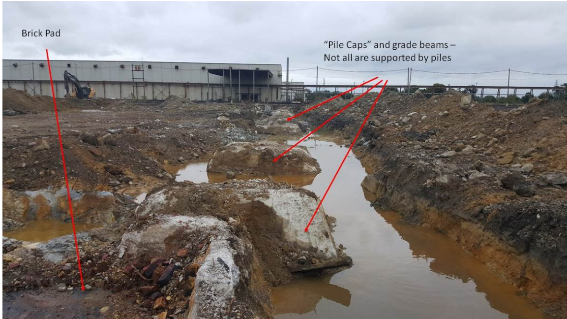
Photo 3: View of concrete pile caps and brick pad.
