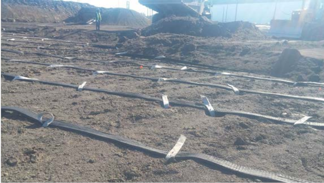
Photo 19: Alternate view of the wick drain installation.
