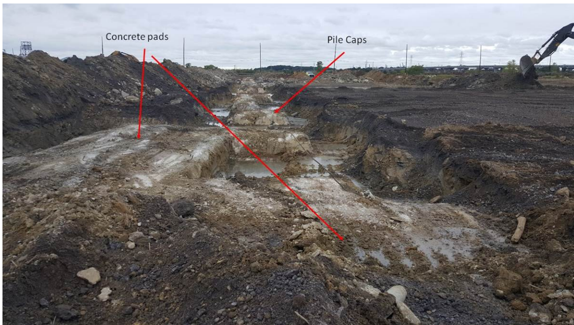
Photo 2: View of former building slabs and concrete pile caps.
