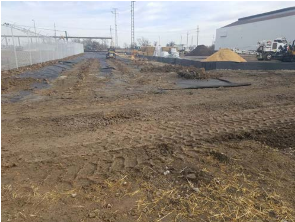
Photo 34: View of geotextile fabric laid in future landscape area.
