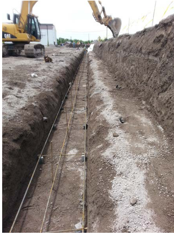
Photo 21: View of excavation activities for main building footers.
