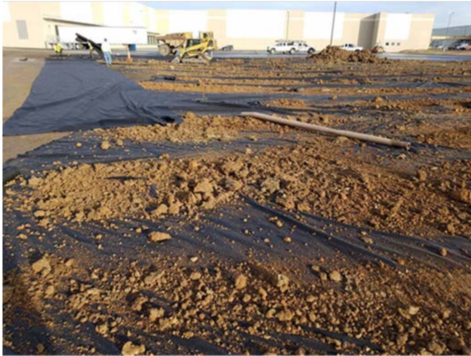
Photo 35: Alternate view of the geotextile fabric in future landscape area.
