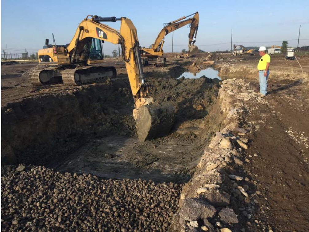
Photo 9: View of excavation for removal of subsurface obstructions.
