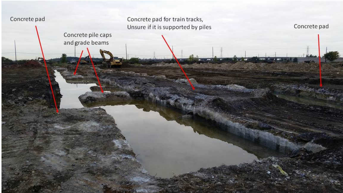
Photo 1: View of former building slabs and concrete pile caps.
