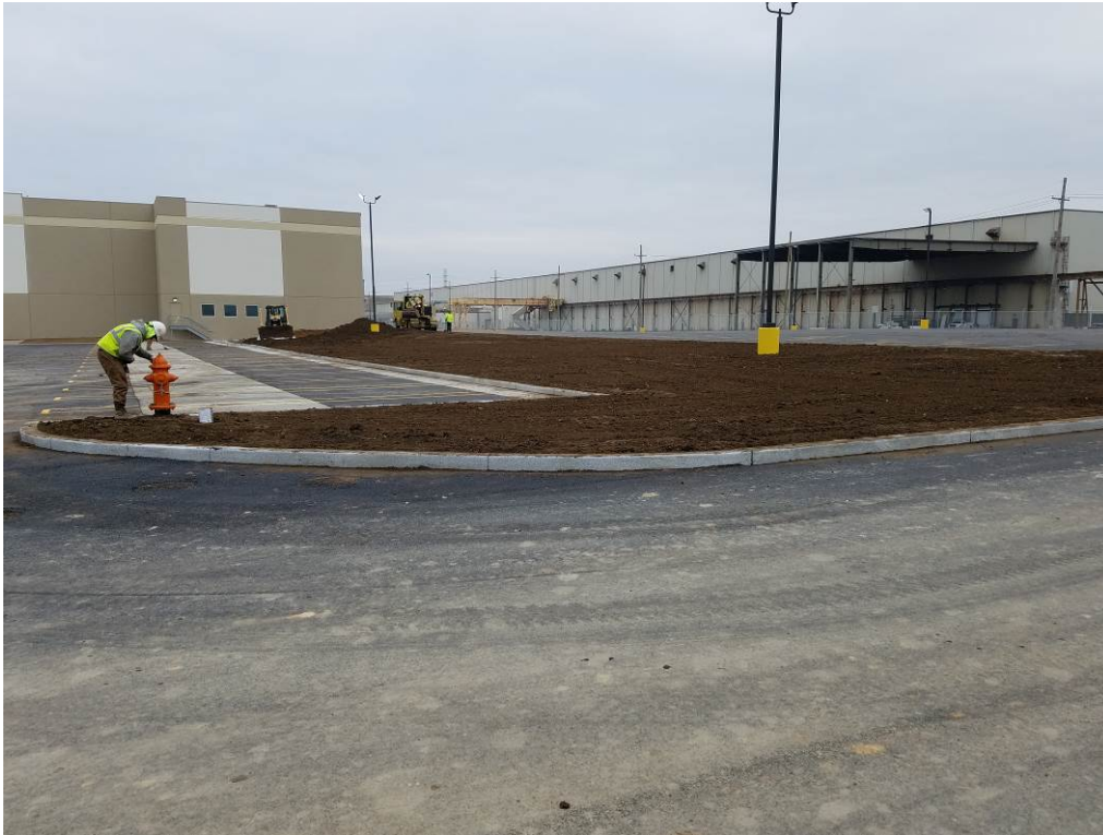
Photo 37: View of completed placement of clean fill cap in landscape area.
