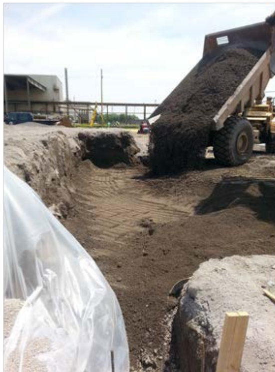
Photo 24: View of backfilling with clean fill material in footer area.
