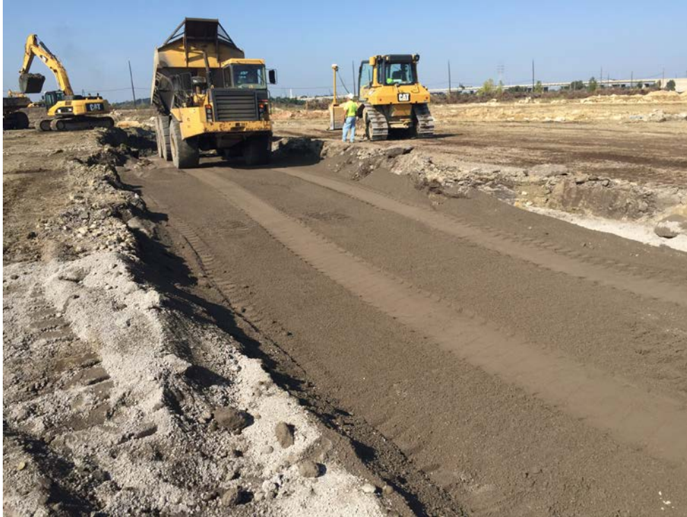
Photo 11: View of trench backfilling with clean structural fill.
