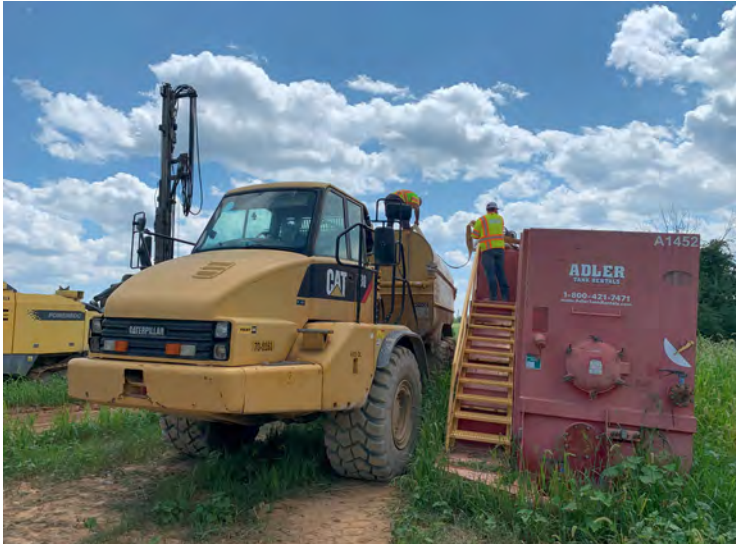
Photo 177: Pumping water from Tank 1 into the water truck for relocation into Tank 2. (August 18, 2023)
