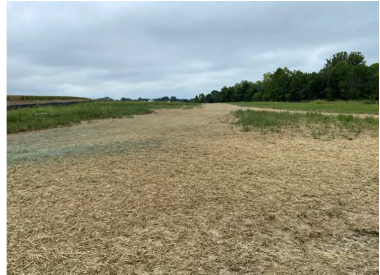
Photo 212: Former construction access road adjacent east of MH-7 following seed/fertilizer mixture and straw application. (August 29, 2023)
