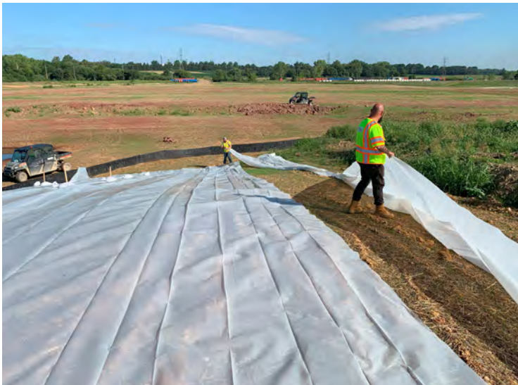
Photo 167: Placing 10 mil plastic sheeting across stockpile east of DA-11. (August 17, 2023)
