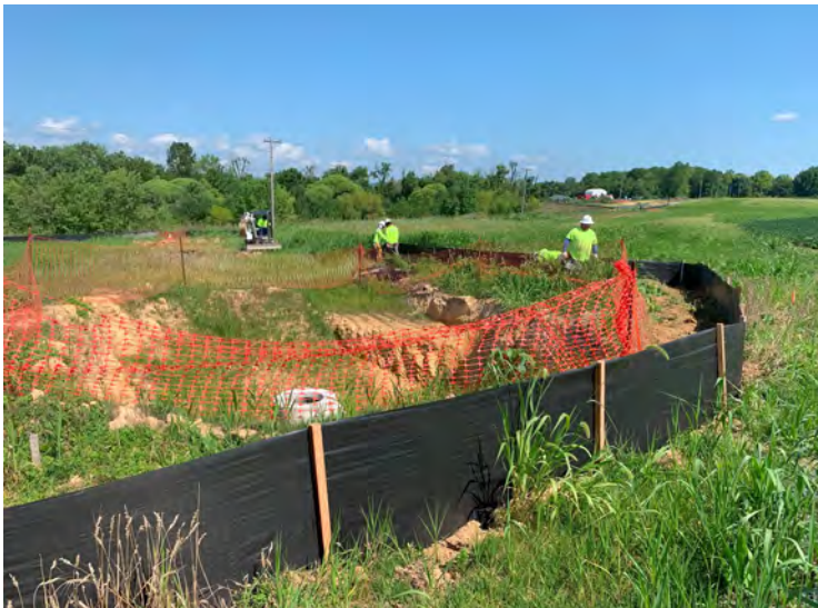
Photo 87: Repairing silt fence surrounding MH-85. (July 31, 2023)
