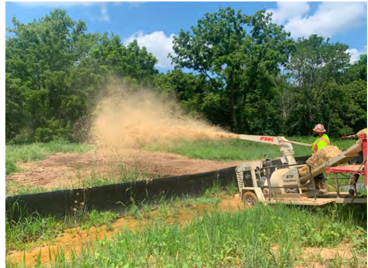
Photo 26: Re-stabilizing floodplain area west of MH-3 with hay following removal of gravel and hay. (July 19, 2023)
