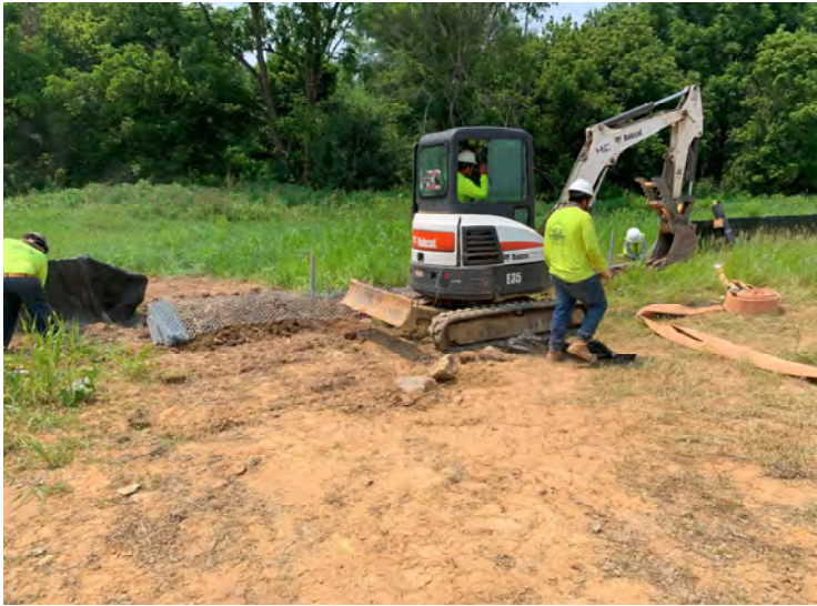
Photo 21: Silt fence installation to repair super silt fence near MH-4. (July 18, 2023)
