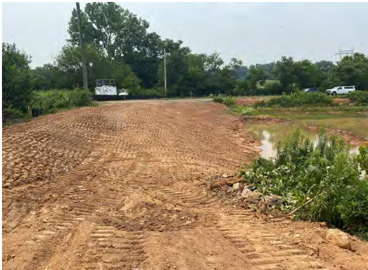
Photo 7: Southeast corner of Basin DA-11 following smoothing operations. (July 17, 2023)
