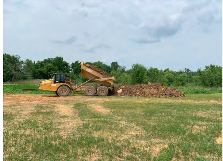
Photo 42: Placing soil from Stockpile 10 into relocation Stockpile A. (July 20, 2023)
