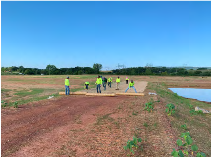
Photo 169: Placing straw matting along Quantum Place South. (August 17, 2023)
