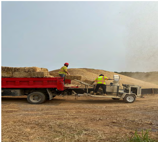
Photo 95: Covering Stockpile D with straw for stabilization. (August 1, 2023)
