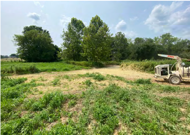
Photo 109: Shooting straw across disturbed areas associated with the floodplain straw bale and filter bag removal south of MH-3. (August 2, 2023)
