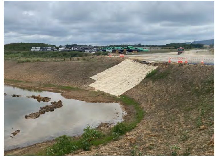
Photo 214: View of curlex straw matting applied to an approximately 12-foot wide section of the western slope of Basin DA-2. (August 29, 2023)
