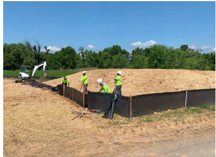
Photo 88: Installation of silt fence around Stockpile A. (July 31, 2023)
