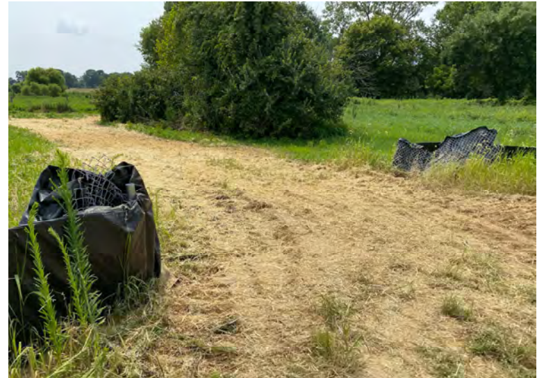
Photo 110: Stabilization using seed and hay across disturbed areas during floodplain straw bale and filter bag removal. (August 2, 2023)
