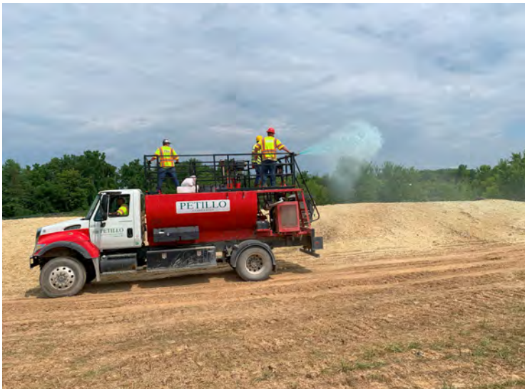
Photo 59: Hydroseeding Stockpile A (July 25, 2023).
