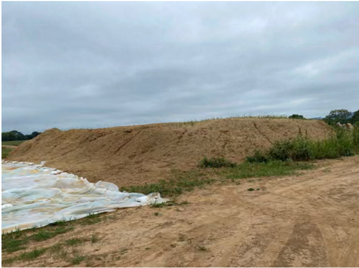
Photo 209: Stockpile 15 following seed/fertilizer mixture and straw application. (August 29, 2023)
