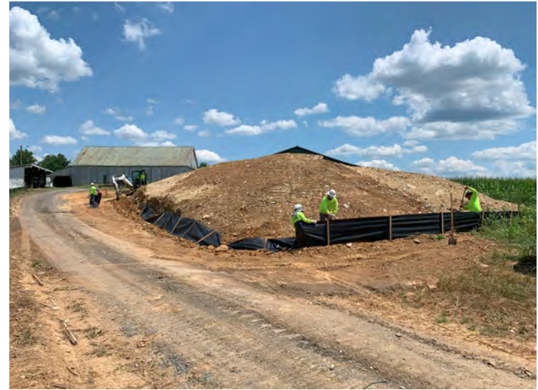
Photo 90: Cutting back northern sidewall of Stockpile B to complete buffer between stockpile and farmers access road. (July 31, 2023)
