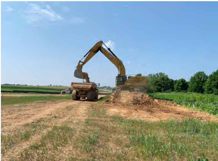
Photo 39: Loading tri-axle end dump with soil from Stockpile 11 for relocation to Stockpile B. (July 20, 2023)
