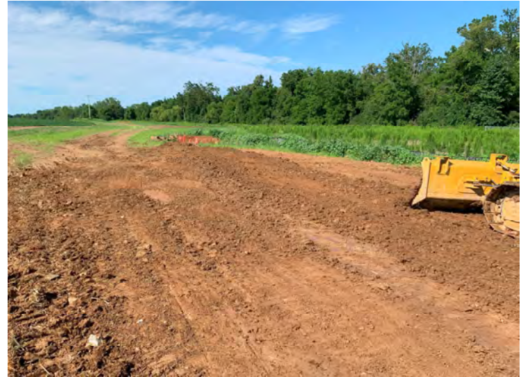
Photo 46: Bulldozer stabilizing sub-grade from relocation of Stockpile 9. (July 21, 2023)
