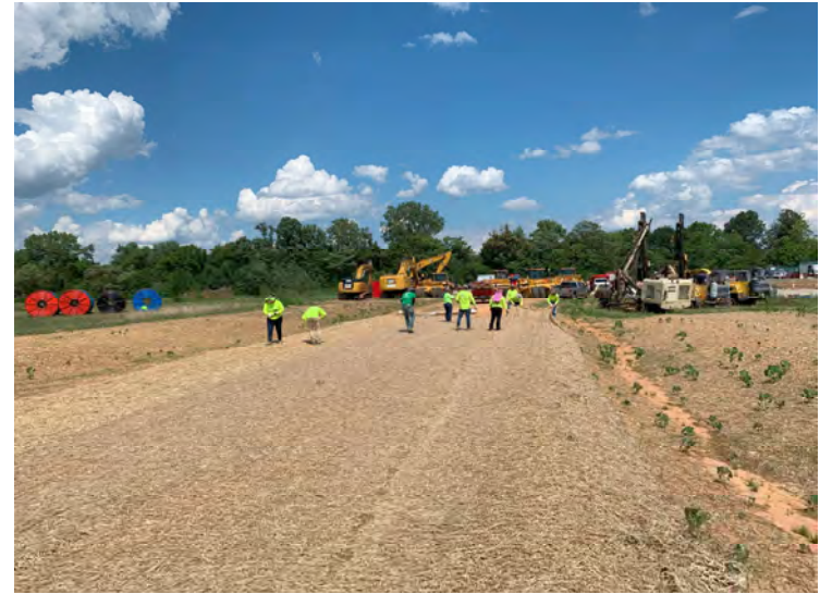
Photo 170: Placing straw matting along Quantum Place South. (August 17, 2023)
