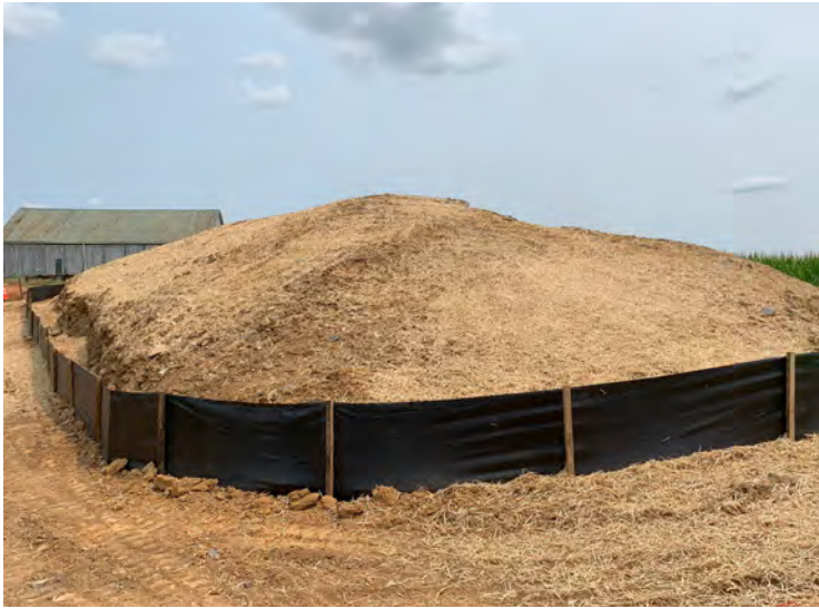
Photo 97: Straw placed atop Stockpile B. (August 1, 2023)
