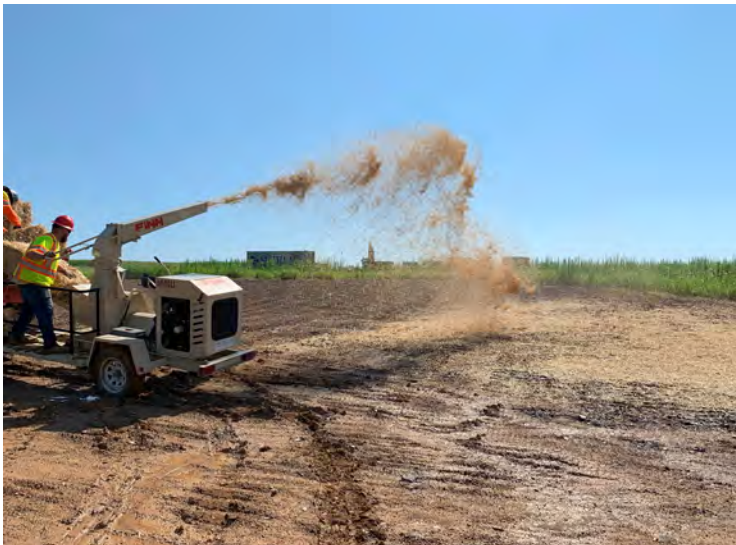
Photo 47: Shooting straw across disturbed areas from relocation of Stockpile 13. (July 21, 2023)
