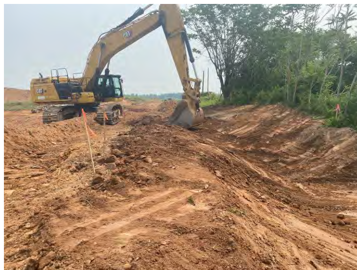
Photo 4: South boundary of Basin DA-11. Previously excavated soils were relocated to re-establish a swale. (July 17, 2023)
