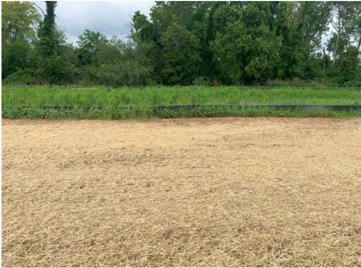
Photo 53: Straw covering disturbed area from relocation of Stockpile 9. (July 24, 2023)
