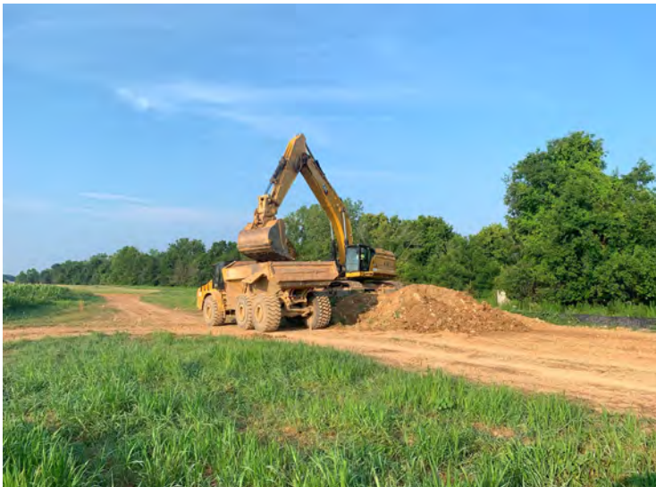
Photo 35: Loading tri-axle end dump with soil from Stockpile 12 for relocation to Stockpile B. (July 20, 2023)
