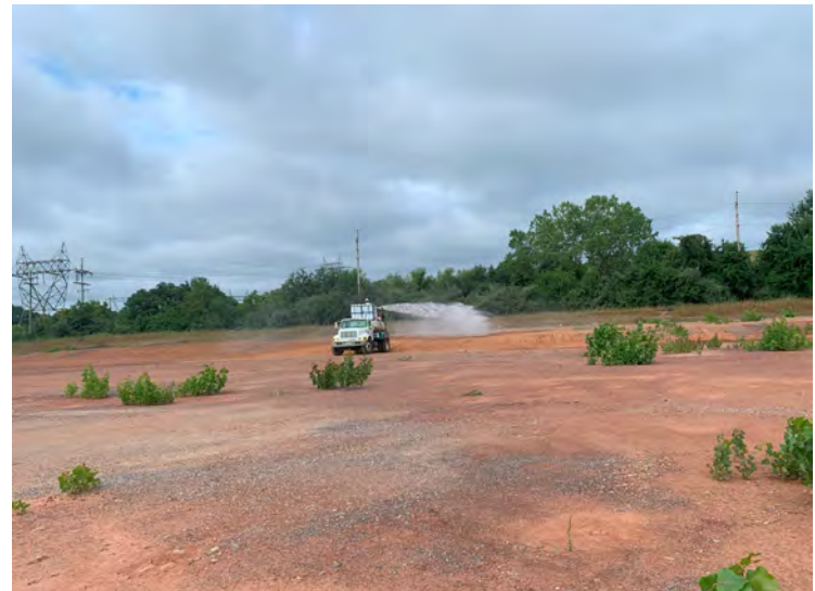
Photo 128: Coating the northeastern portion of the substation pad with seed-fertilizer mixture. (August 7, 2023)
