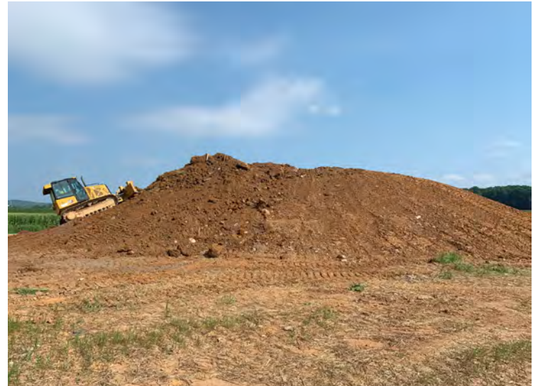
Photo 80: Grading soil placed into Stockpile D with a bulldozer. (July 28, 2023)
