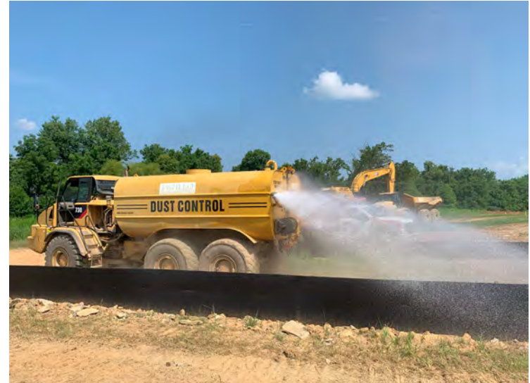
Photo 38: Hydrating haul road to prevent dust generation. (July 20, 2023)
