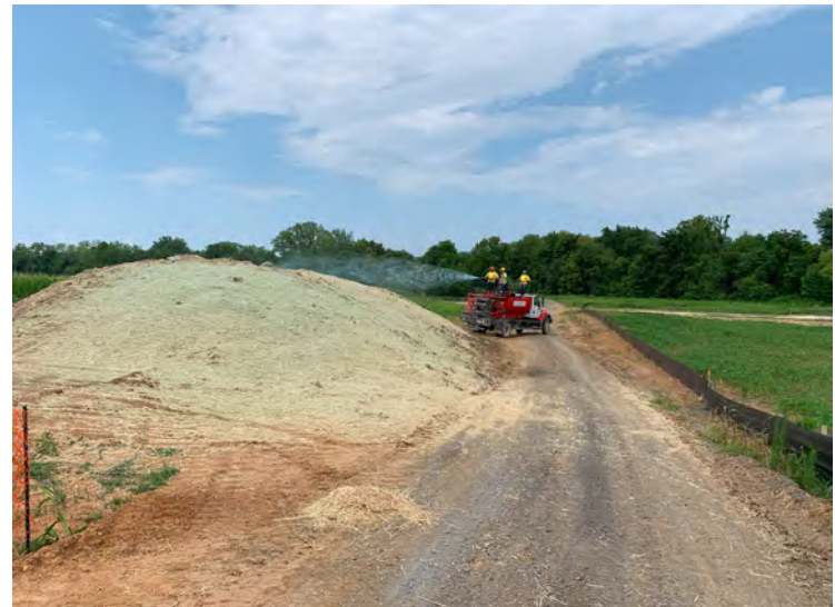
Photo 60: Hydroseeding Stockpile B (July 25, 2023).
