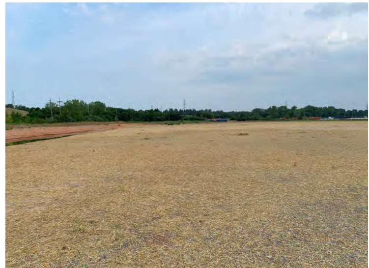
Photo 116: Stabilization with straw and seed across the substation pad. (August 2, 2023)
