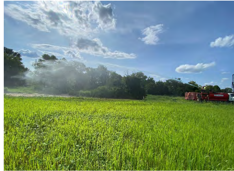
Photo 34: Hydroseeding area following removal of hay bales south of MH-3. (July 19, 2023)
