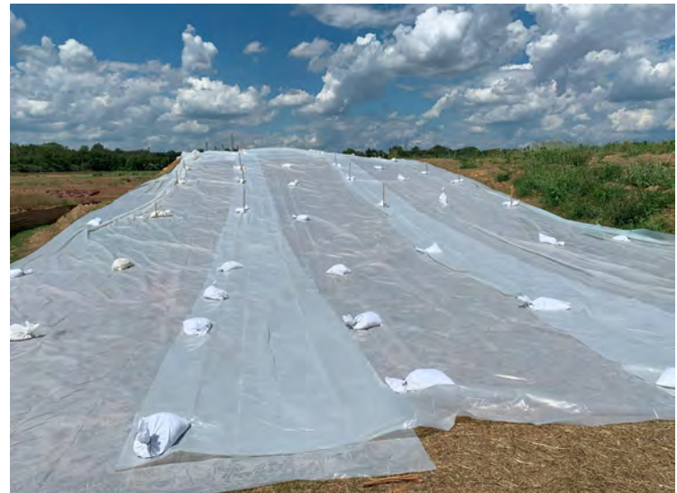
Photo 168: Sandbags and wooden stakes used to anchor plastic sheeting. (August 17, 2023)
