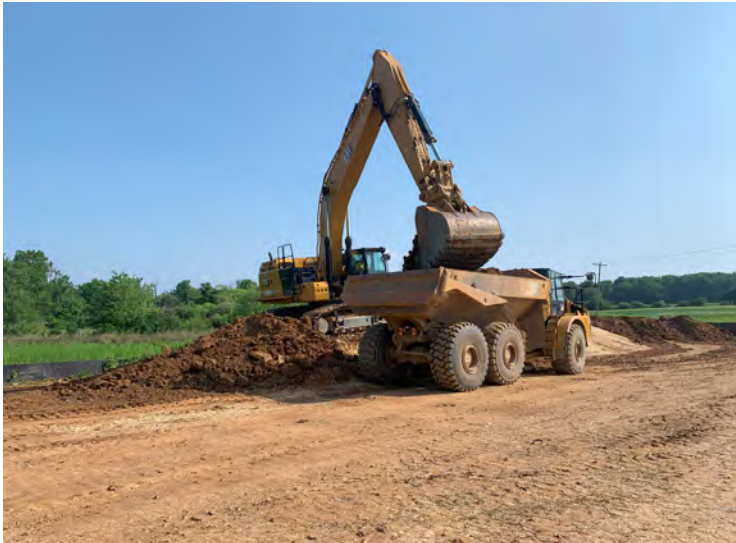
Photo 79: Loading soil from Stockpile A into dump truck for relocation into Stockpile D. (July 28, 2023)
