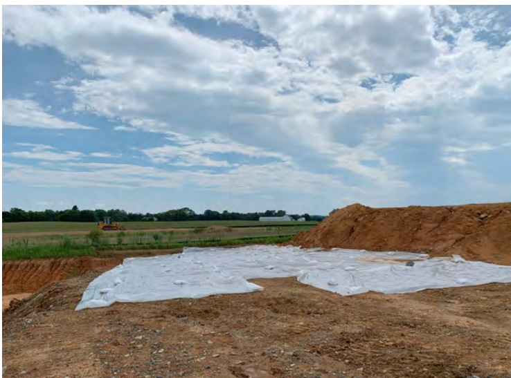
Photo 135: Progress of 10 mil plastic sheeting placed across Stockpile C. (August 8, 2023)
