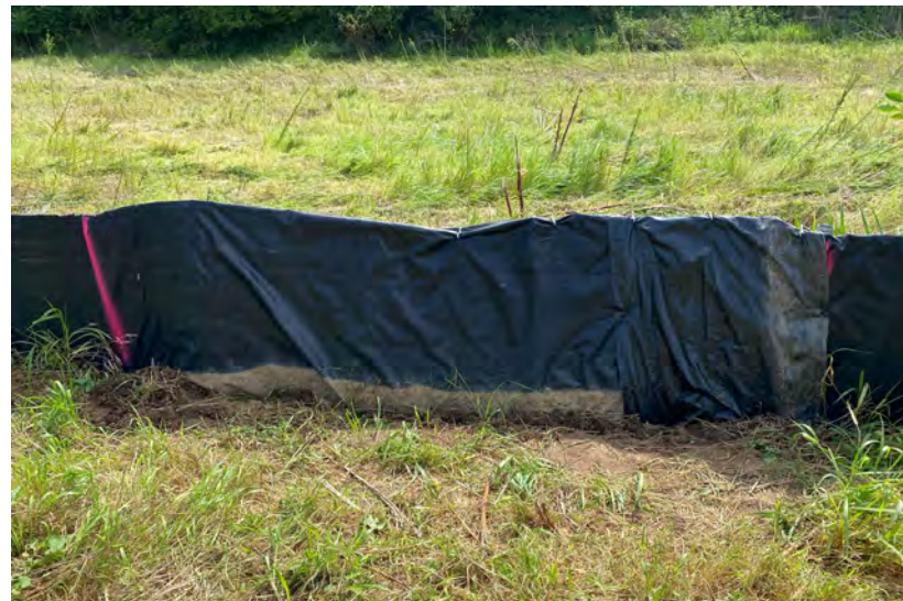
Photo 154: Repaired silt fence.
