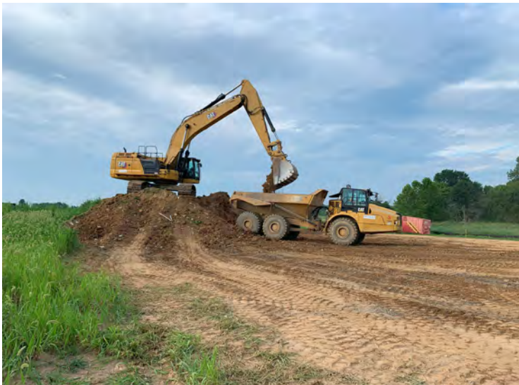
Photo 23: Loading tri-axle dump truck with soil from Stockpile 13 for relocation into Basin 3. (July 19, 2023)
