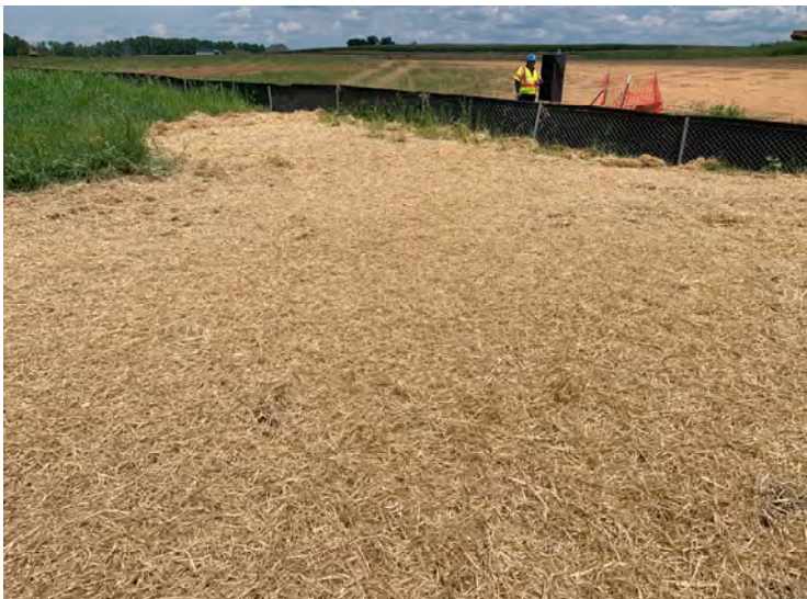
Photo 27: Hay spread across floodplain area west of MH-3. (July 19, 2023)
