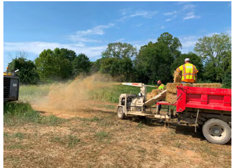
Photo 200: Shooting straw atop seed/fertilizer mixture to stabilize disturbed sub-grade. (August 23, 2023)
