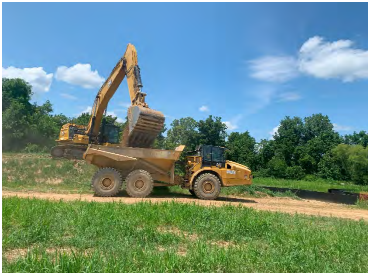
Photo 31: Loading tri-axle dump truck with soil from Stockpile 12 for relocation. (July 17, 2023)
