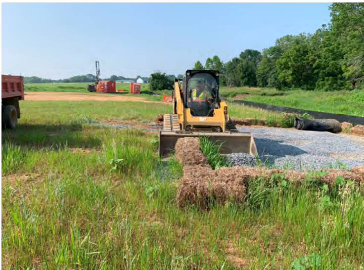
Photo 19: Removing hay bales and gravel from floodplain area located between MH-4 and MH-5. (July 18, 2023)
