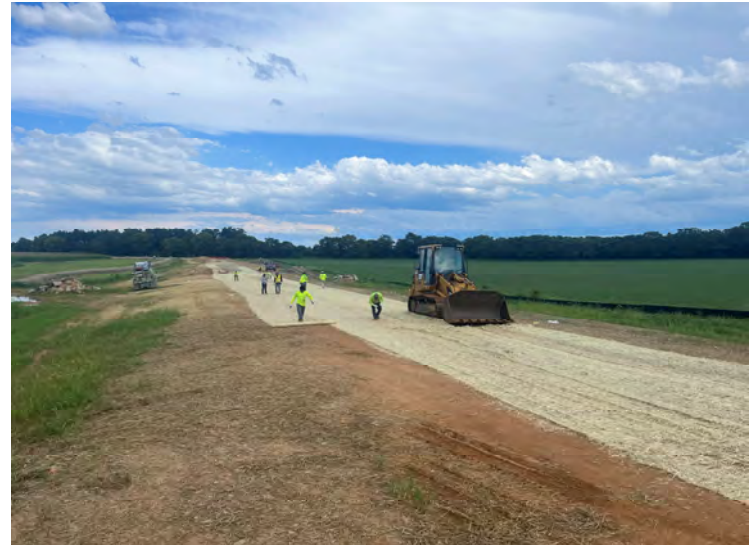
Photo 162: Placing the final straw matting along the southern portion of Happy Landing Road. (August 15, 2023)
