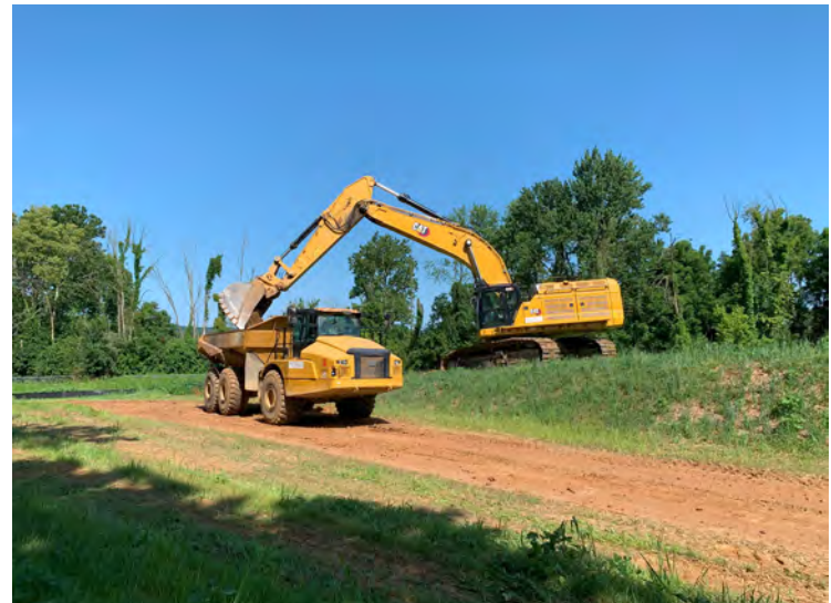
Photo 48: Loading tri-axle end dump with soil from Stockpile 7 for relocation to Stockpile A. (July 21, 2023)
