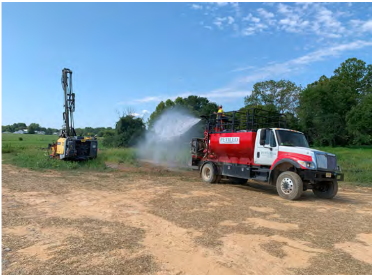
Photo 199: Spraying seed/fertilizer mixture across disturbed sub-grade from the former frac tank location. (August 23, 2023)
