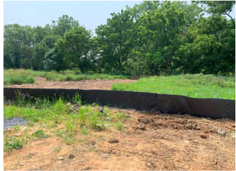
Photo 22: Completed super silt fence repair. (July 18, 2023)
