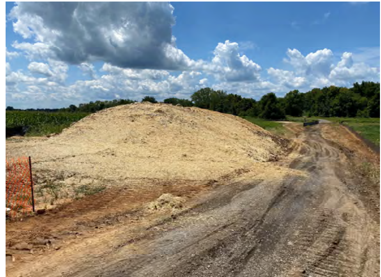
Photo 50: Straw placed atop Stockpile B for stabilization. (July 21, 2023)
