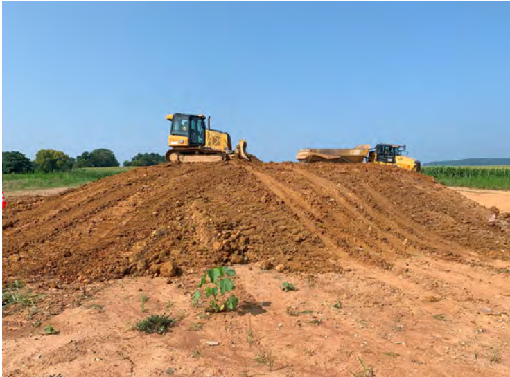
Photo 63: Bulldozer grading soil into Stockpile D. (July 26, 2023)
