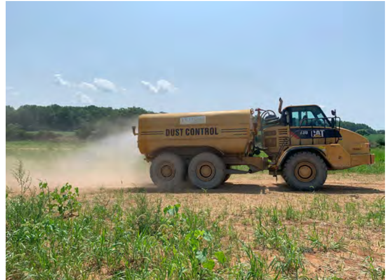
Photo 64: Water suppression for dust control along haul road leading from stockpile locations. (July 26, 2023)
