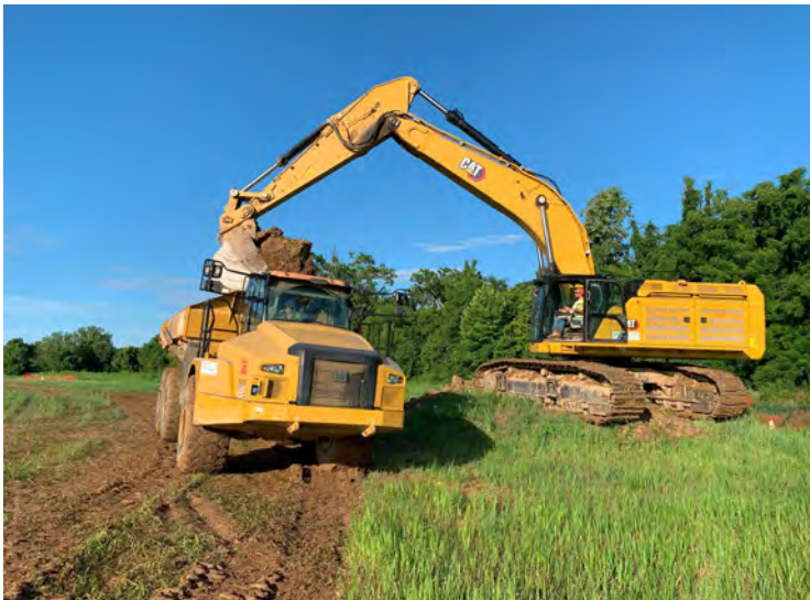
Photo 43: Loading tri-axle end dump with soil from Stockpile 10 for relocation to Stockpile A. (July 21, 2023)
