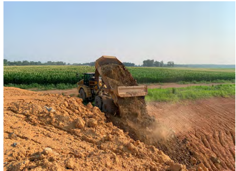
Photo 16: Placing soil from Stockpile 13 into Basin 3. (July 18, 2023)
