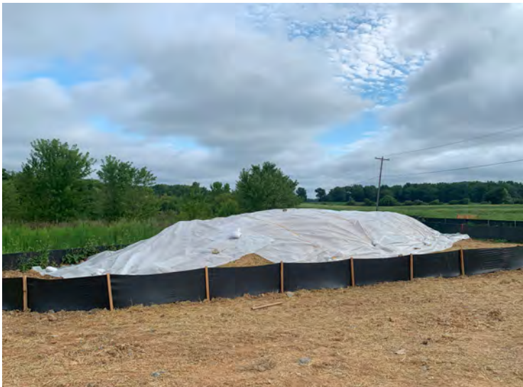
Photo 127: Stockpile A covered with plastic sheeting. (August 7, 2023)
