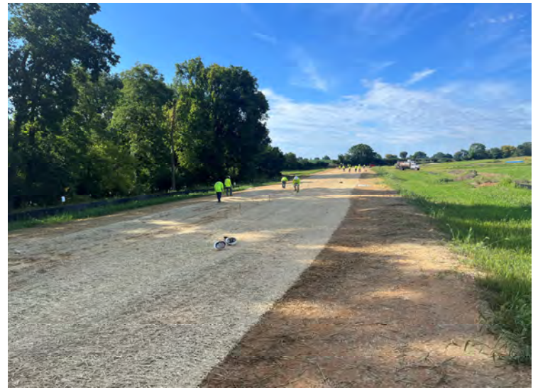
Photo 160: HEC continuing south on Happy Landing Road, placing additional straw matting to cover the future roadway area. (August 15, 2023)
