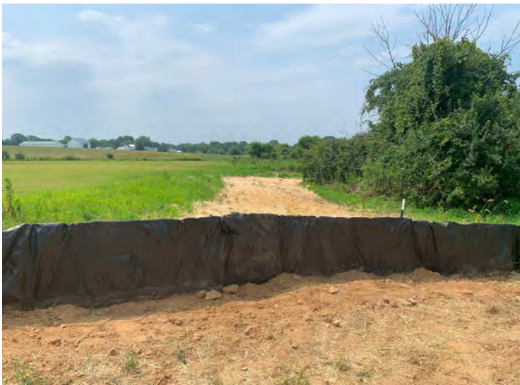
Photo 115: Repaired silt fence south of MH-3. (August 2, 2023)
