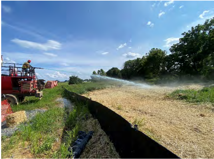
Photo 33: Hydroseeding area following removal of hay bales and gravel west of MH-4. (July 19, 2023)
