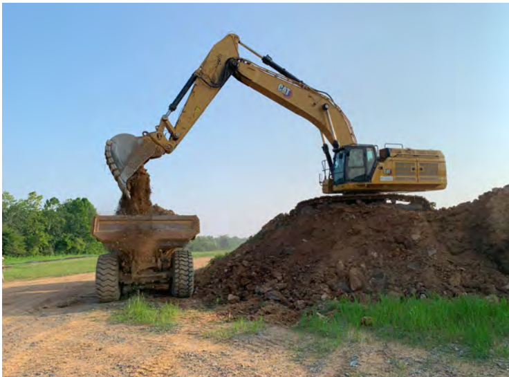
Photo 15: Loading tri-axle dump truck with soil from Stockpile 13 for relocation into Basin 3. (July 18, 2023)
