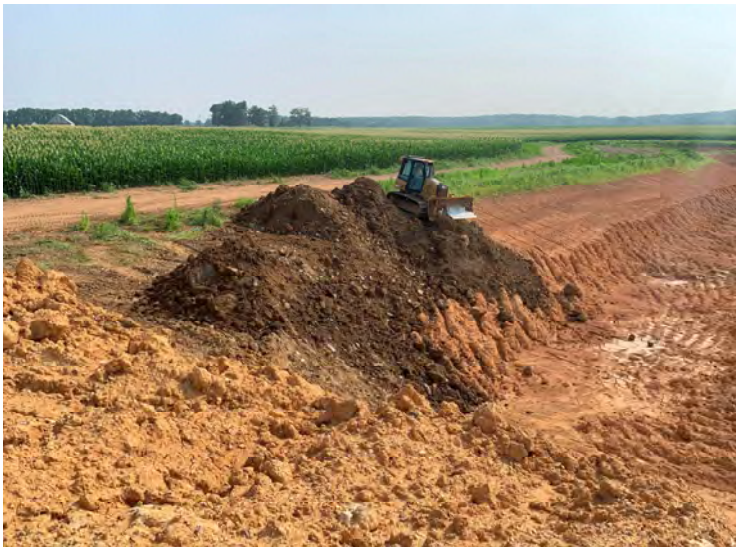
Photo 17: Using a bulldozer to push soils into Basin 3. (July 18, 2023)
