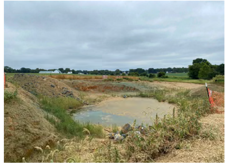
Photo 210: Pump station excavation following seed/fertilizer mixture and straw application. (August 29, 2023)
