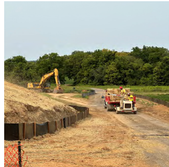
Photo 96: Covering Stockpile B with straw for stabilization. (August 1, 2023)
