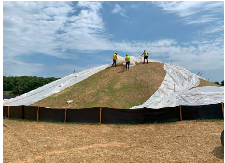
Photo 202: Re-securing plastic sheeting atop Stockpile D. (August 23, 2023)
