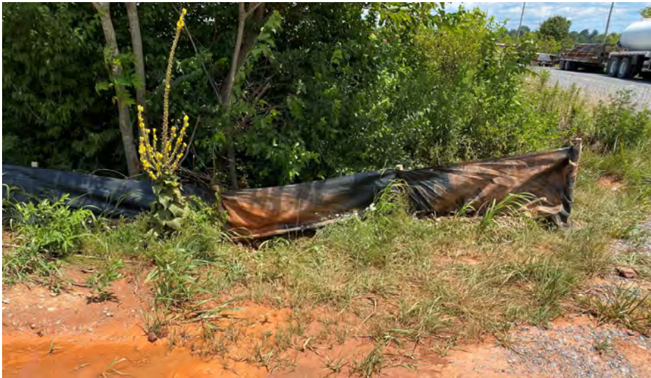
Photo 49: Reestablished silt fence along access road to the borrow pit. (July 21, 2023)
