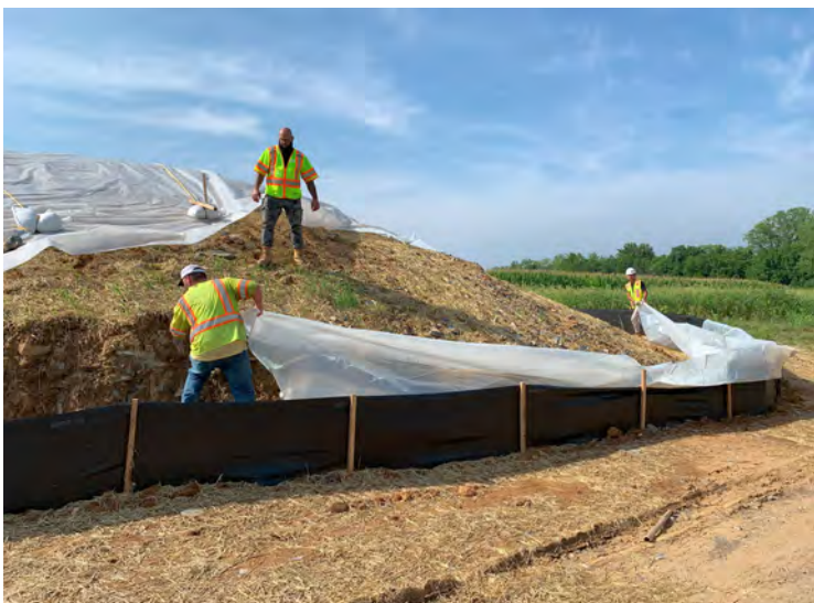
Photo 151: Placing 10 mil plastic sheeting across Stockpile D. (August 11, 2023)
