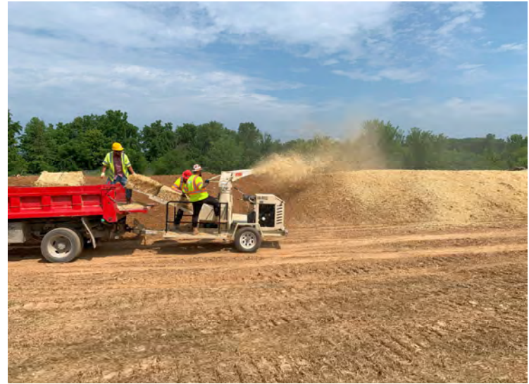
Photo 58: Placing straw atop Stockpile A. (July 25, 2023)
