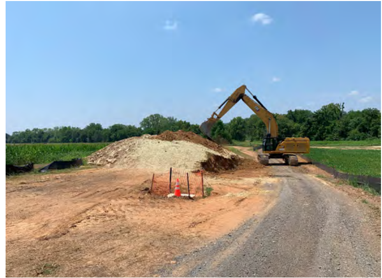
Photo 82: Cutting back northern sidewall of Stockpile B to complete buffer between stockpile and farmers access road. (July 28, 2023)
