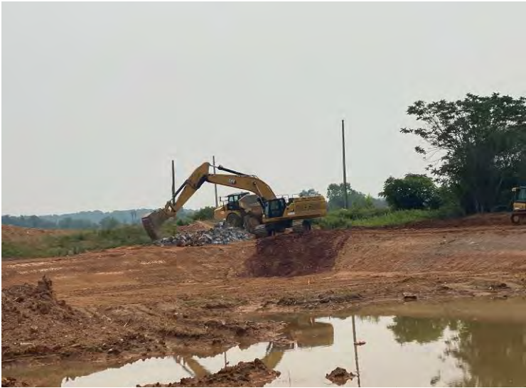
Photo 9: Crushed concrete loaded onto end dump with excavator. (July 17, 2023)
