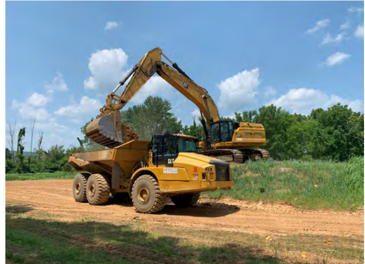
Photo 66: Placing soil into dump truck from Stockpile 7 for relocation to Stockpile D. (July 26, 2023)
