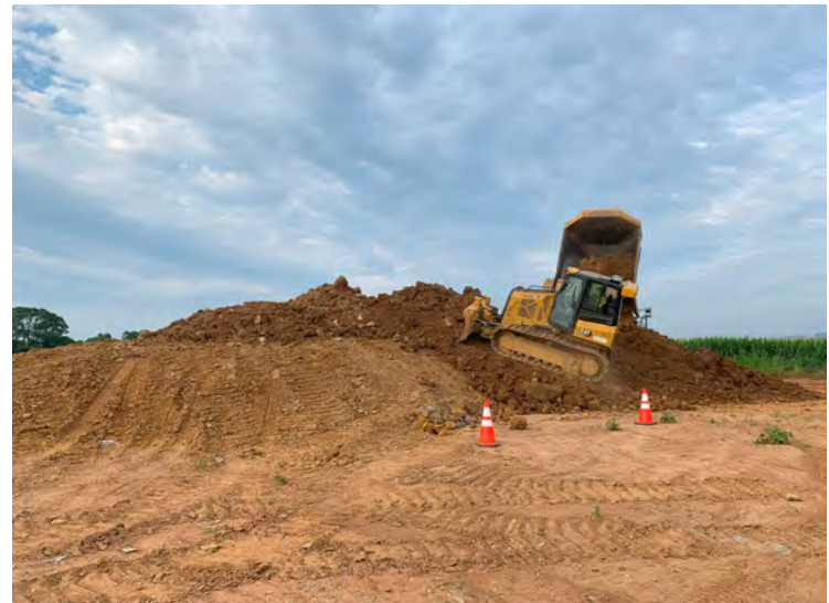
Photo 72: Grading soil placed into Stockpile D with a bulldozer. (July 27, 2023)
