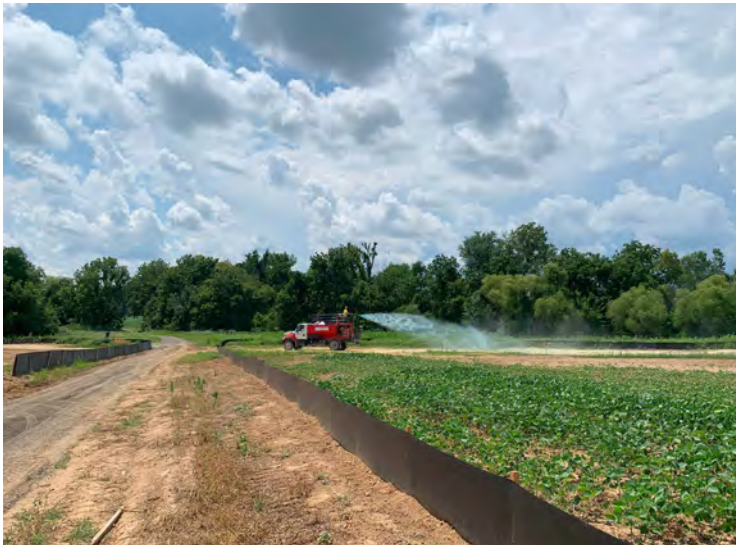
Photo 55: Hydroseeding disturbed area associated with former Stockpile 11. (July 24, 2023)
