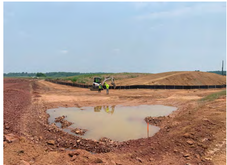
Photo 20: Silt fence installation around stockpile areas located east of DA-11. (July 18, 2023)
