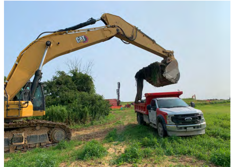
Photo 104: Loading straw and filter bag into a dump truck for disposal into designated relocation stockpile near Happy Landing Road. (August 2, 2023)
