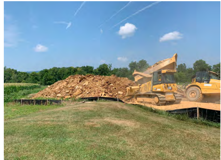
Photo 40: Bulldozer grading deposited soils into Stockpile B. (July 20, 2023)
