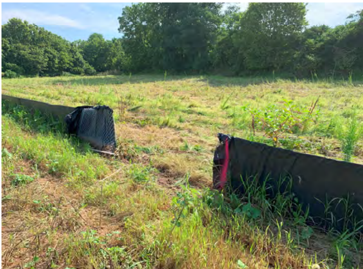
Photo 153: Temporarily removed silt fence opened to allow landscaping equipment entry.
