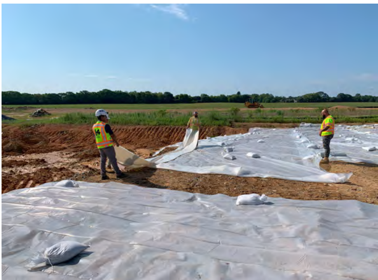
Photo 143: Placing 10 mil plastic sheeting across Stockpile C. (August 8, 2023)
