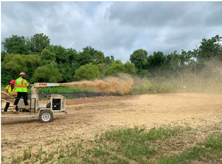
Photo 51: Shooting straw across disturbed area from relocation of Stockpile 10. (July 24, 2023)
