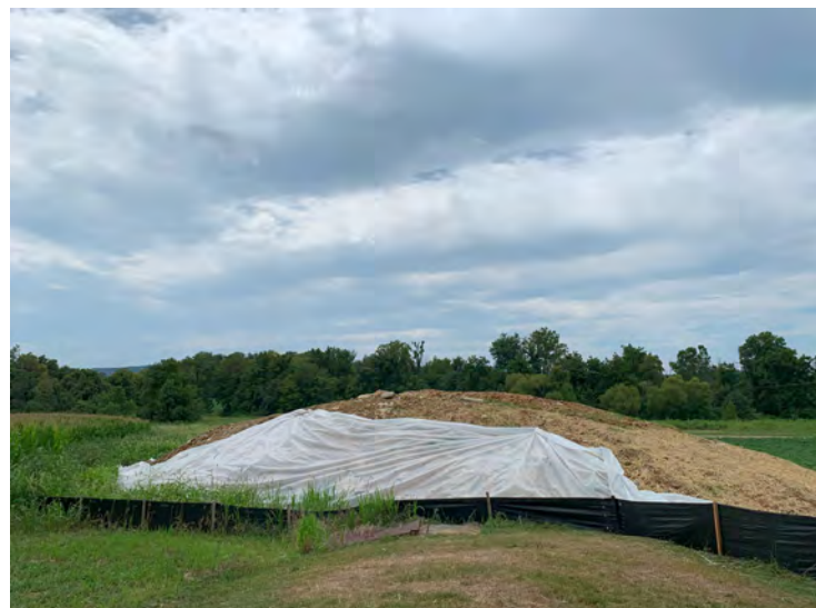
Photo 136: Progress of 10 mil plastic sheeting placed across Stockpile B. (August 8, 2023)
