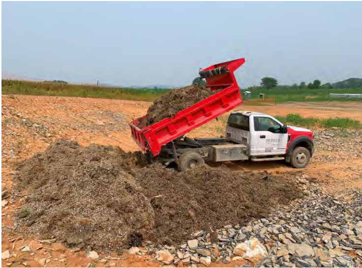
Photo 13: Placing gravel and hay into temporary stockpile location adjacent to Happy Landing Road. (July 17, 2023)
