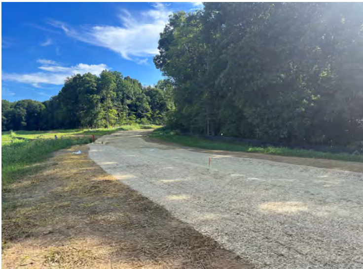
Photo 159: Extent of straw matting placed on Happy Landing Road on the previous day. (August 15, 2023)
