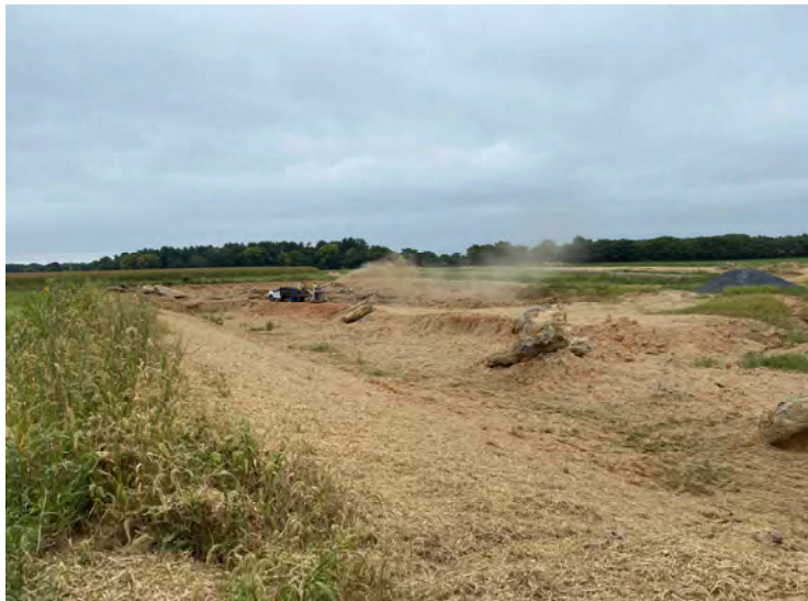
Photo 207: Shooting straw atop seed/fertilizer mixture at Basin 3. (August 29, 2023)
