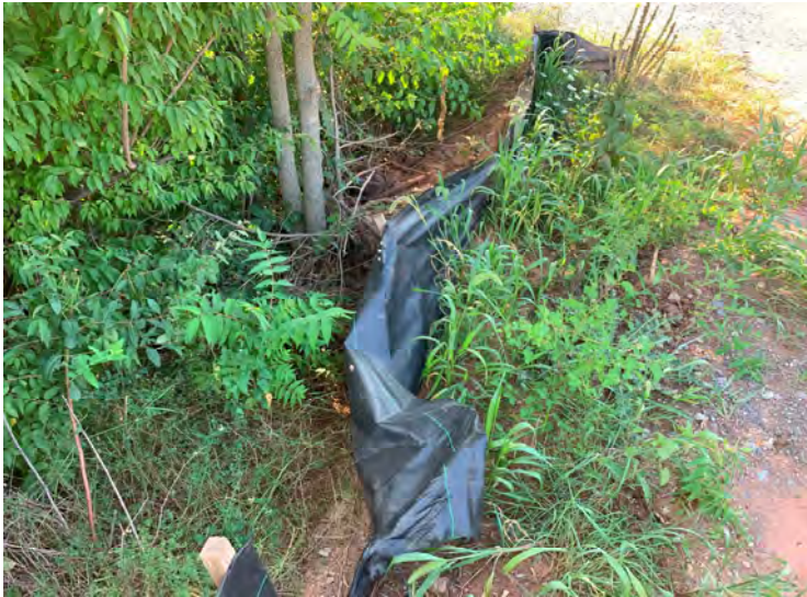
Photo 91: Impaired silt fence near borrow pit entrance. (July 31, 2023)
