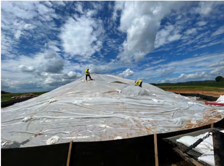
Photo 161: Replacing plastic sheeting on Stockpile D. (August 15, 2023)
