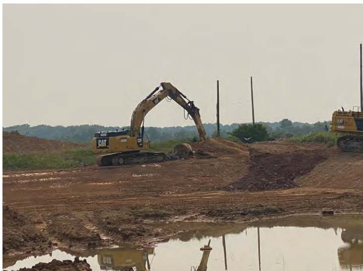
Photo 1: Previously excavated concrete crushed by a hoe ram. (July 17, 2023)
