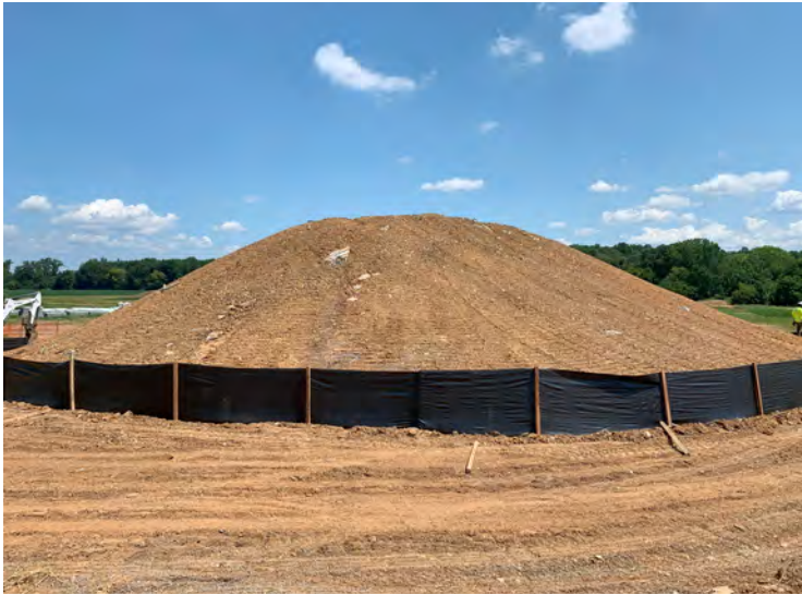
Photo 89: Silt fence installed around Stockpile C. (July 31, 2023)
