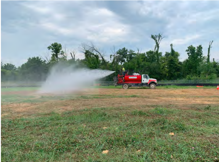
Photo 73: Covering disturbed surface area from stockpile relocation activities with seed. (July 27, 2023)
