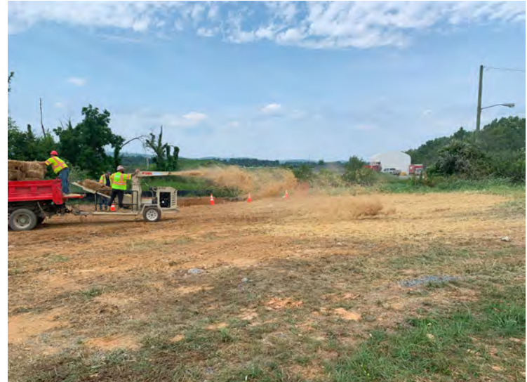
Photo 74: Spreading straw across disturbed areas following stockpile relocation. (July 27, 2023)
