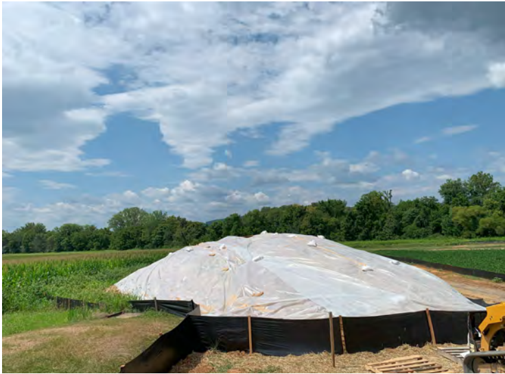
Photo 145: Plastic sheeting completely covering Stockpile B. (August 8, 2023)
