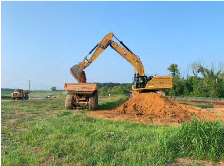
Photo 61: Loading soil from Stockpile 4 into a dump truck for relocation into Stockpile D. (July 26, 2023)
