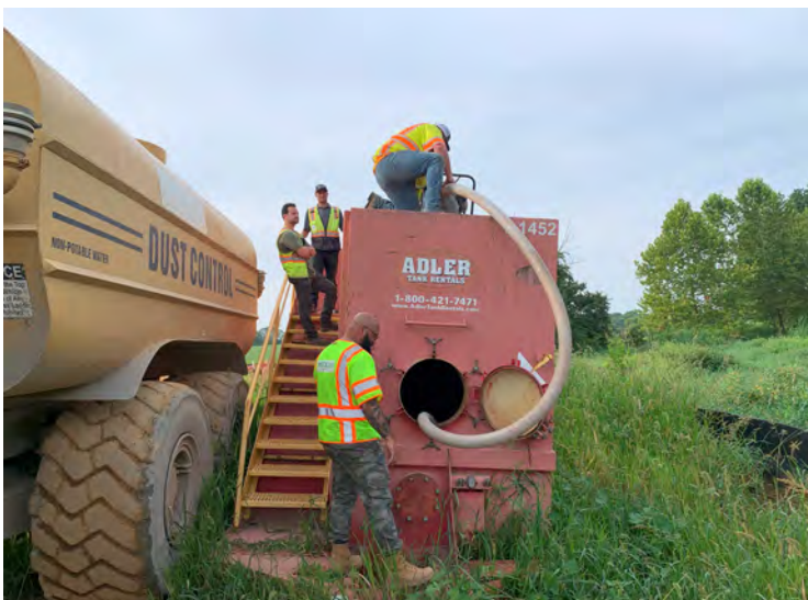
Photo 183: Pumping water from Tank 1 into water truck for relocation into Tank 2. (August 21, 2023)
