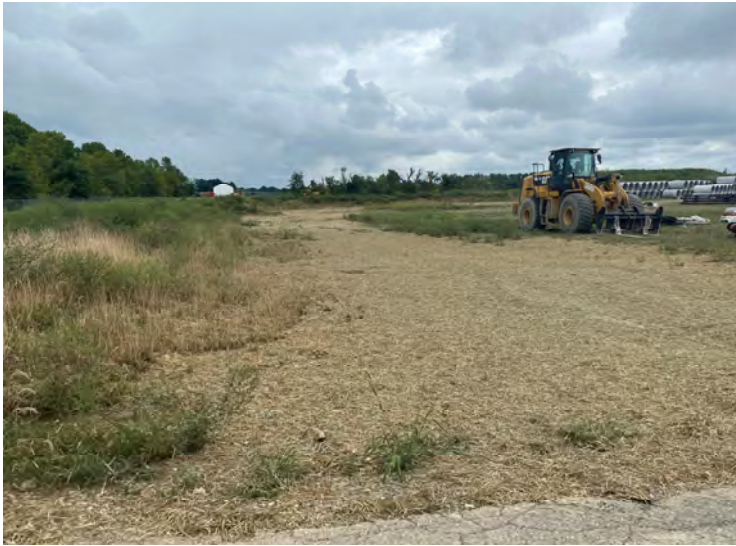
Photo 213: Former construction access road located adjacently west of Basin DA-2 following seed/fertilizer mixture and straw application. (August 29, 2023)
