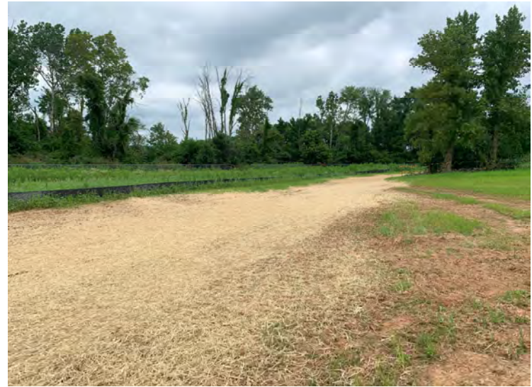
Photo 54: Straw spread across haul road in the LOD leading to Stockpile 7. (July 24, 2023)
