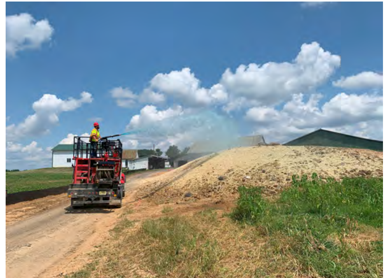
Photo 56: Hydroseeding Stockpile B. (July 24, 2023)
