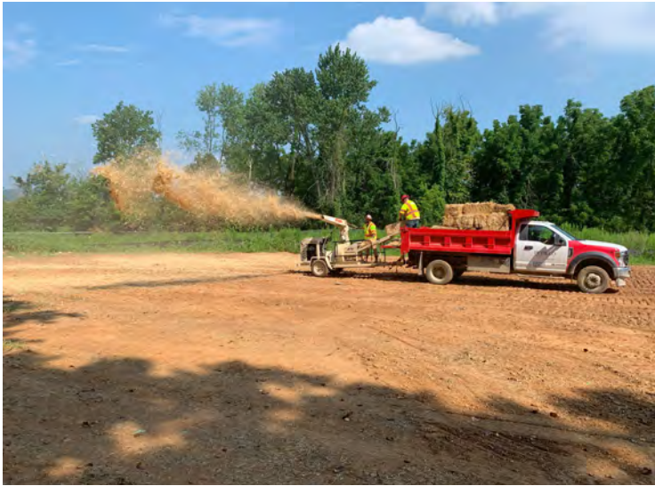
Photo 81: Covering disturbed surface area from Stockpile 7 relocation activities with straw. (July 28, 2023)
