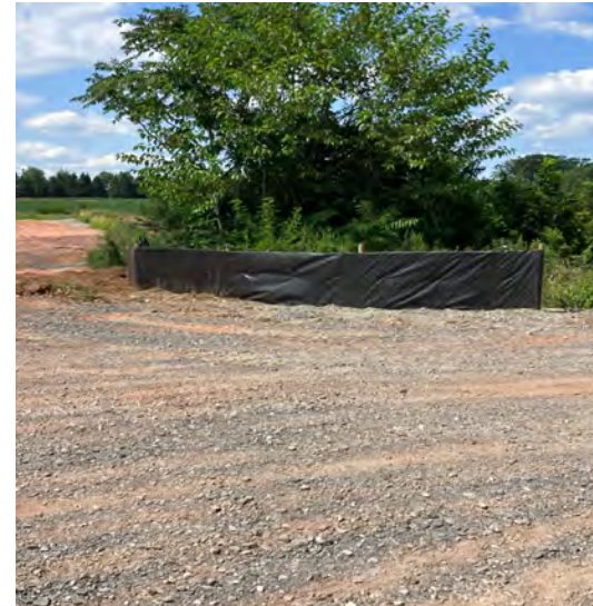
Photo 92: Installation of new silt fence near borrow pit entrance. (July 31, 2023)
