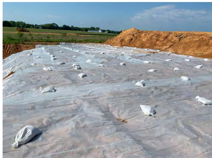
Photo 1444: Plastic sheeting completely covering Stockpile C. (August 8, 2023)
