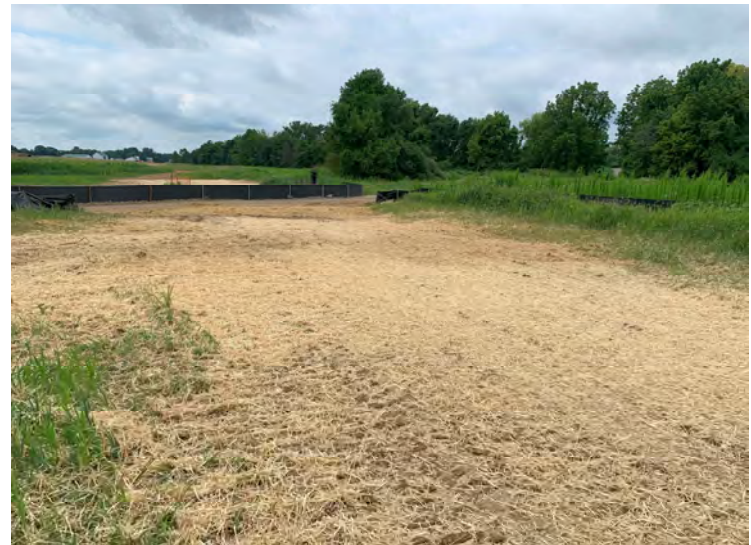
Photo 52: Straw covering disturbed area from the relocation of Stockpile 11. (July 24, 2023)
