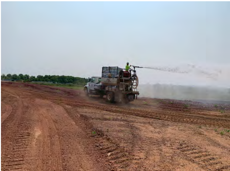
Photo 107: Spraying seed-fertilizer mixture across the edges of Quantum Place South. (August 2, 2023)
