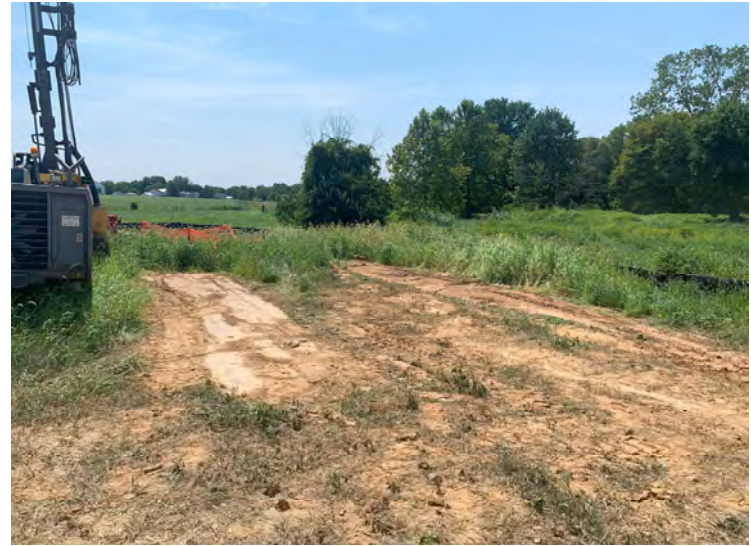
Photo 194: Disturbed sub-grade associated with footprint of Tanks 1 and 2. (August 22, 2023)
