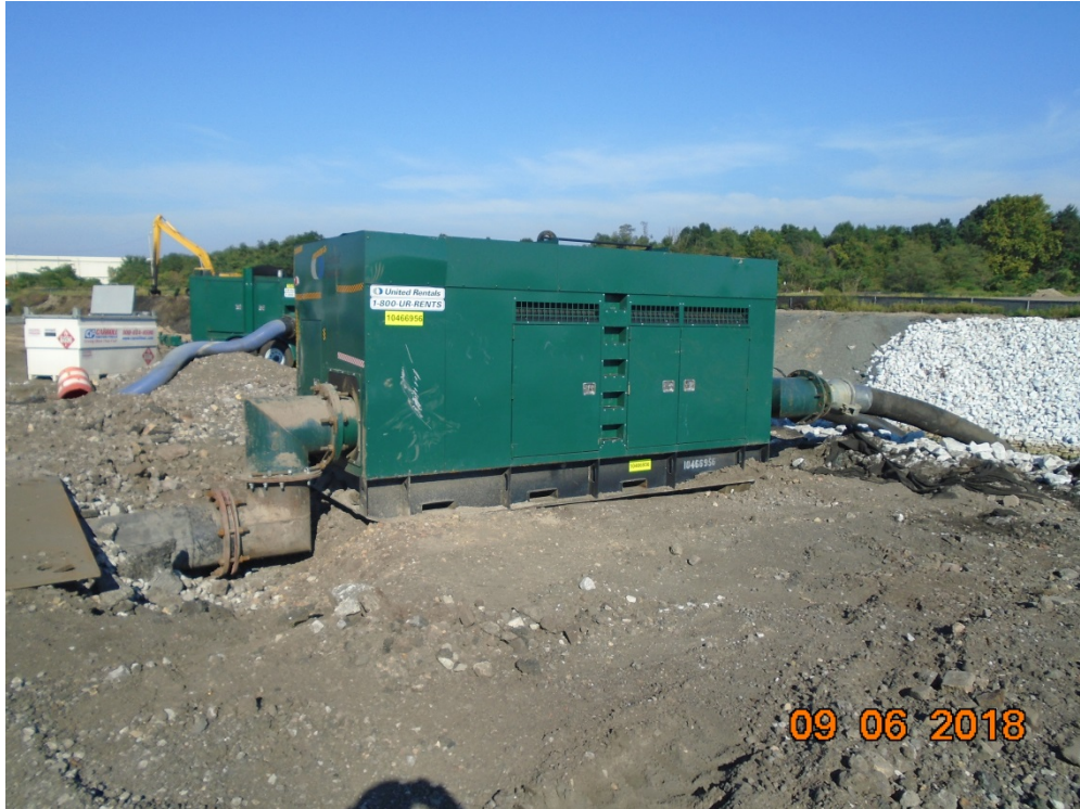
Photo 13: View of pumps used to remove water from the Tin Mill Canal, water pumped to Waste Water Treatment Plant.
