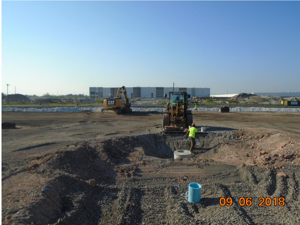
Photo 11: View of water main manway installation on the northern portion of the Property, looking south.
