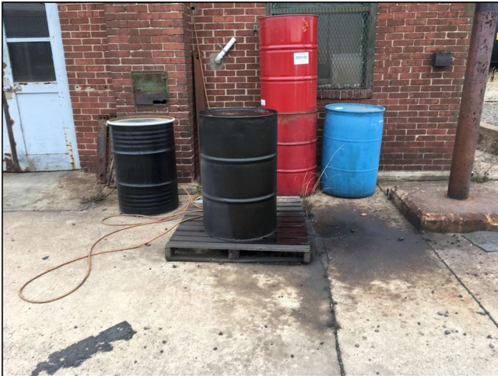
020118-2: Petroleum staining observed on the concrete surface along the exterior of the small Oil House.
