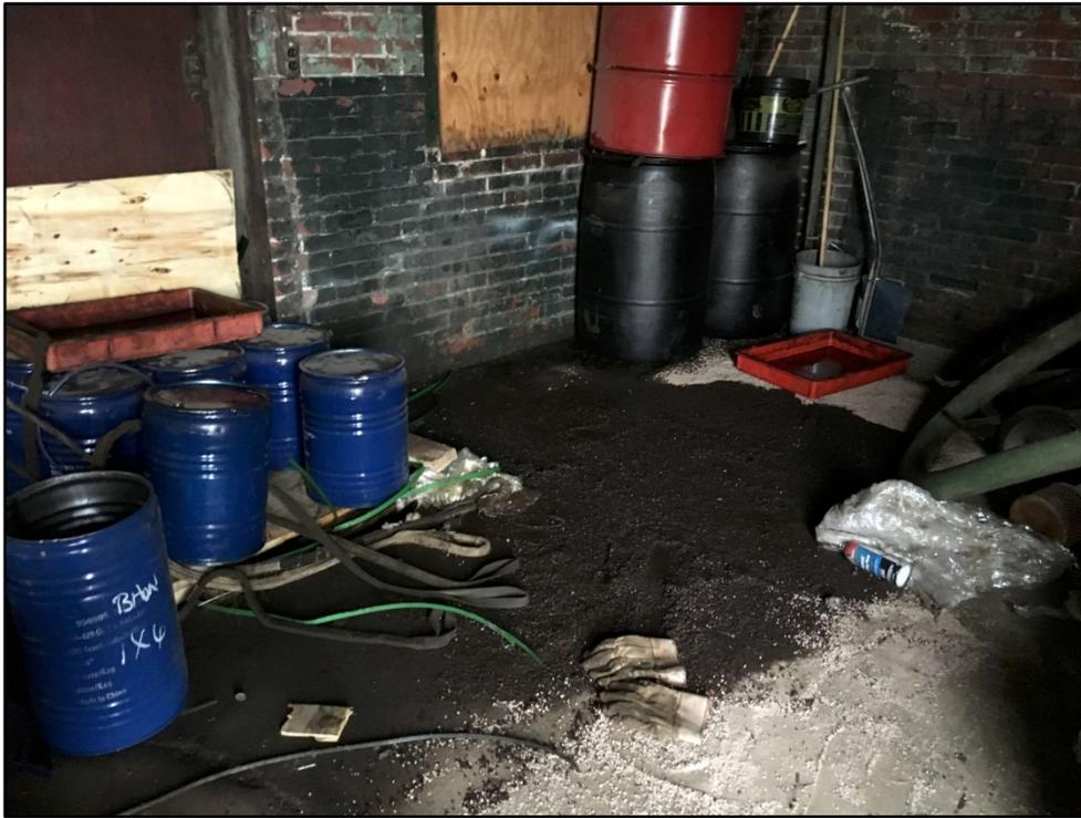
020118-3: Petroleum staining observed on the concrete surface within the small Oil House.
