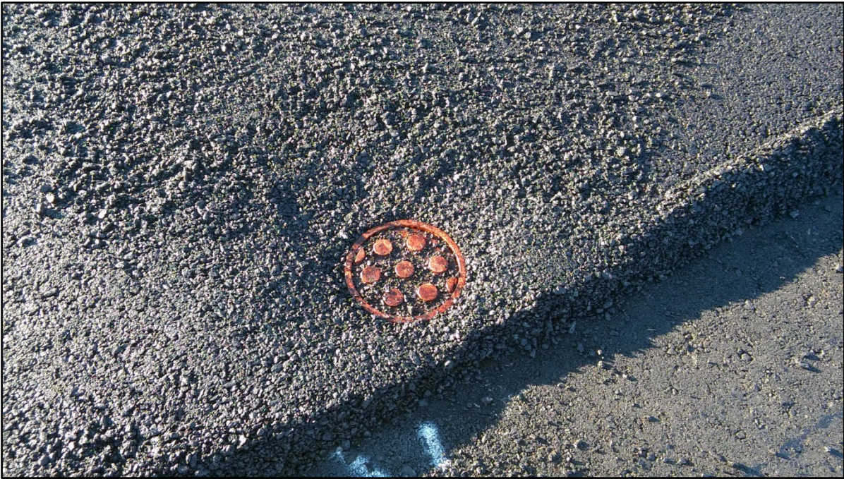
110716-44: View of paved-over and re-exposed piezometer cap.
