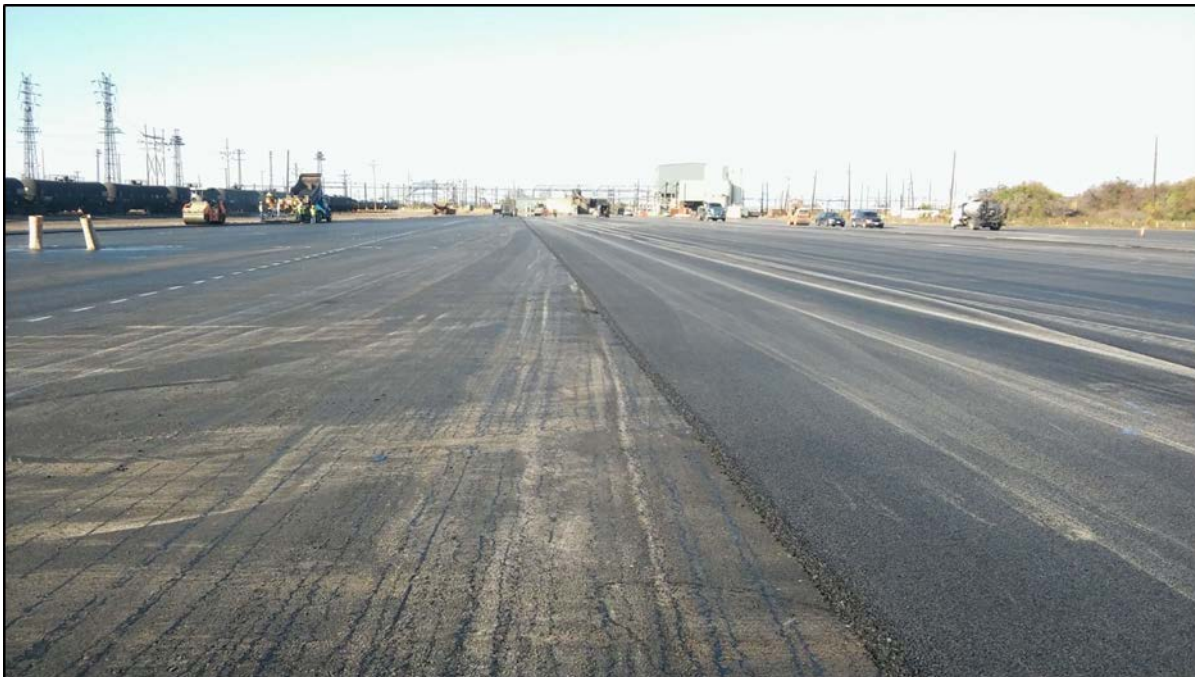
110416-1: View to the west of the start of second layer paving activities on western portion of the site. Visible are the two monitoring wells and tacked areas of the first layer of pavement.
