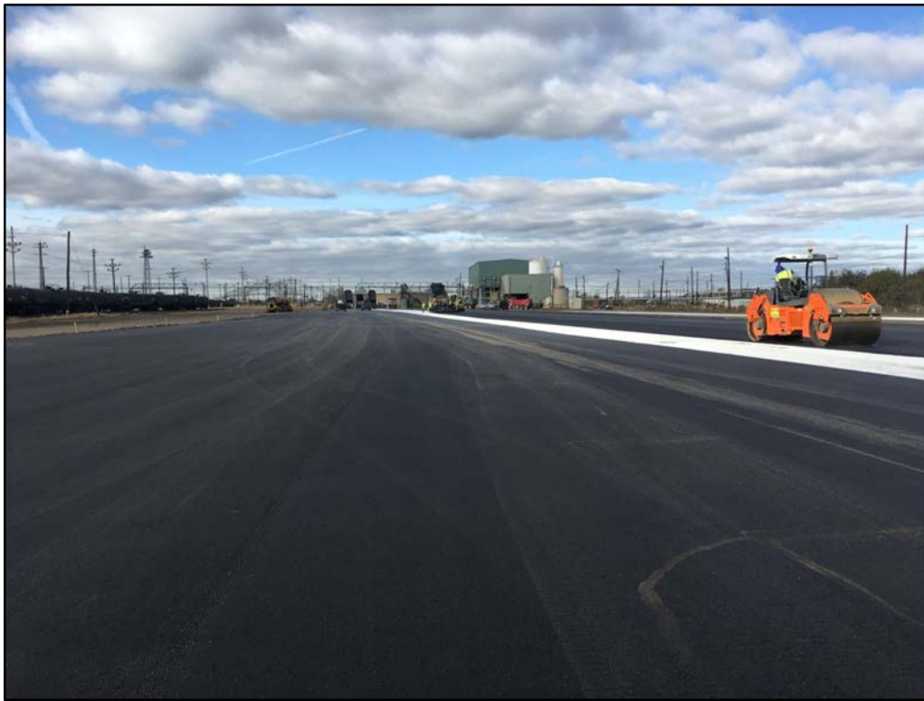
103116-1: View to west from center of site. Visible are first layer light-duty paving activities on western side of site.
