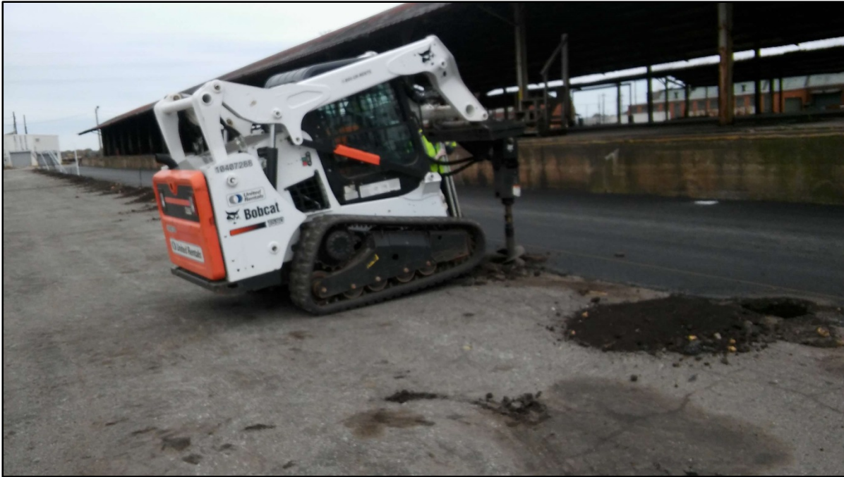
110116-1: Fence post drilling and digging activities along northern edge of building.
