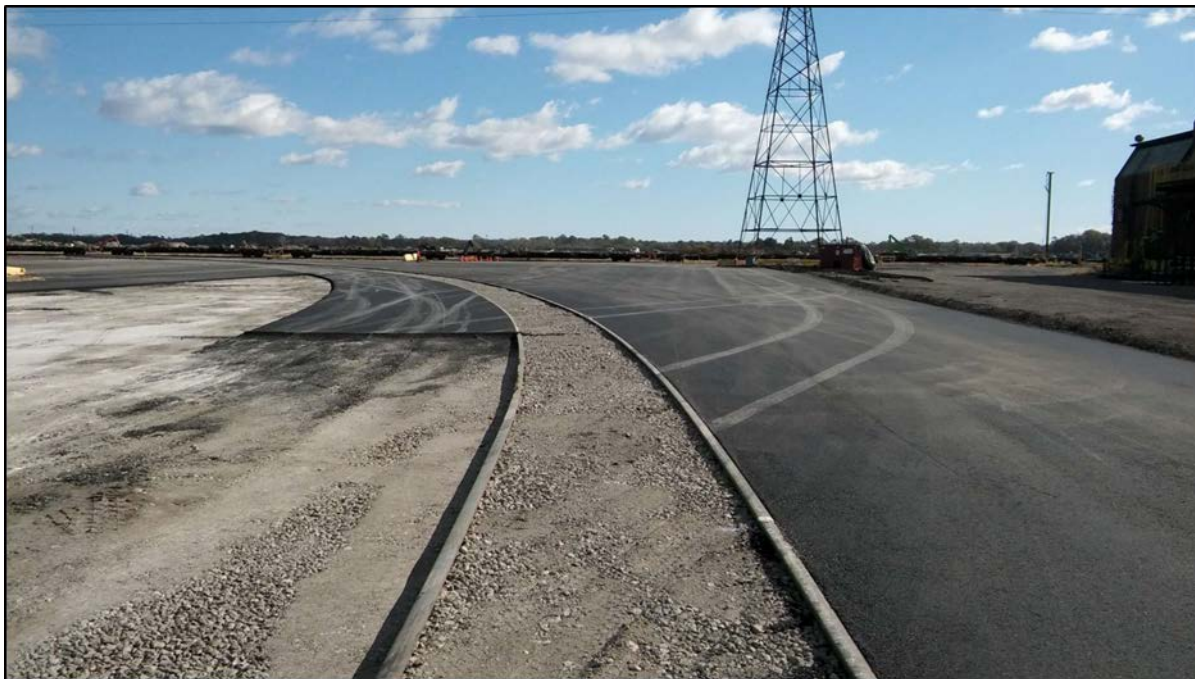
102816-2: Edge of first layer of paving on southeast corner of site.
