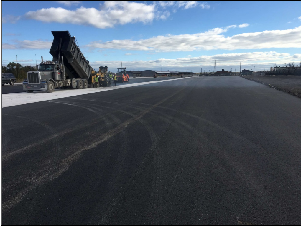
103116-2: View to the east of first light-duty layer paving activities.
