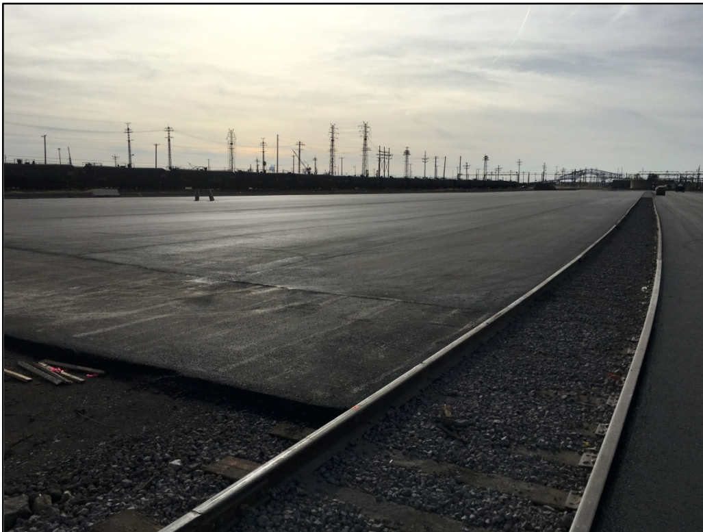
103116-3: View to the west of second layer heavy duty paving on each side of railroad tracks.
