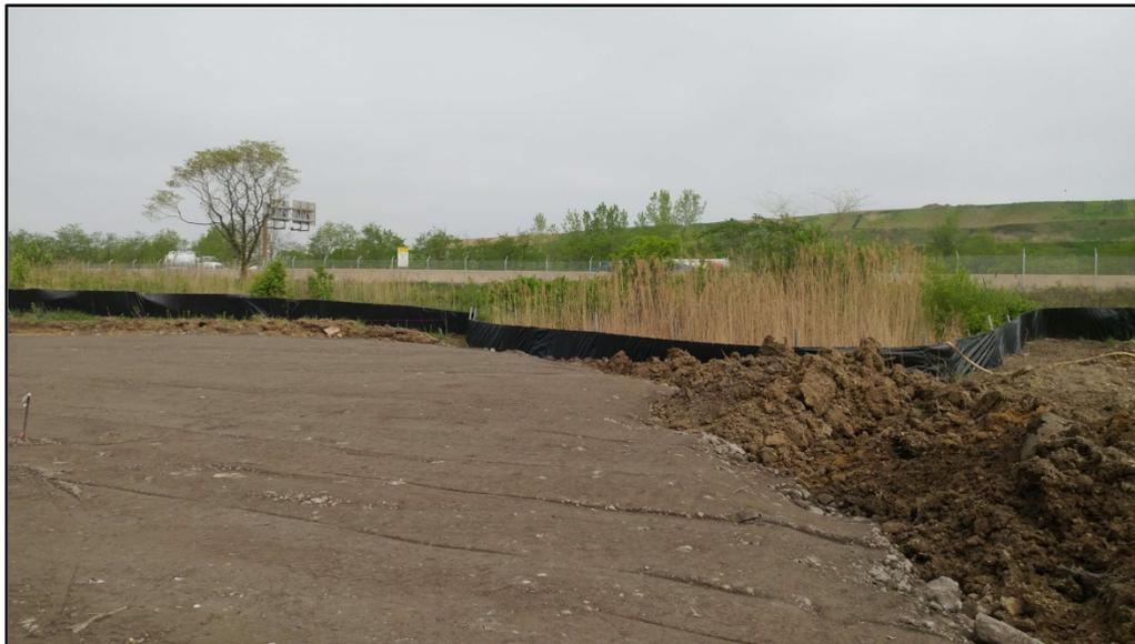
042717-2: Silt fence and parking area subgrade preparation north of NCMC building.
