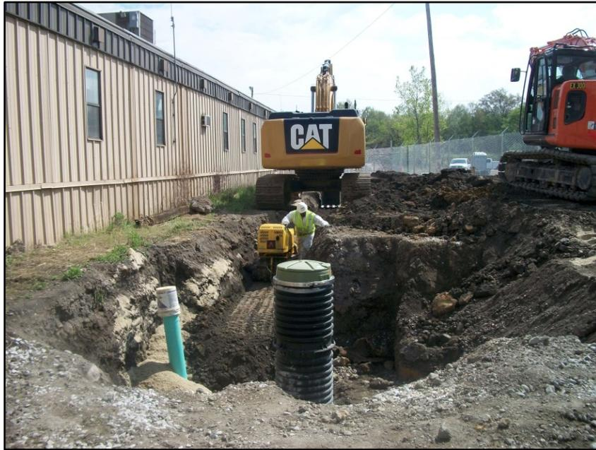
042017-3: Utility work and backfilling for truck well construction on east side of NCMC building.
