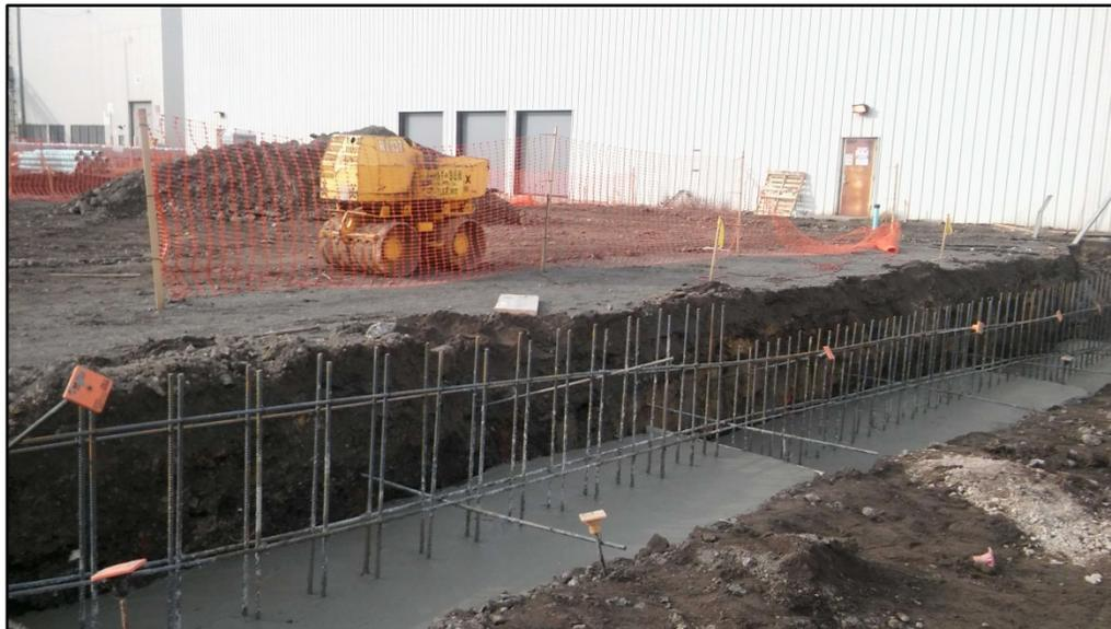
011917-1: Concrete foundation for truck well construction on south side of NCMC building.
