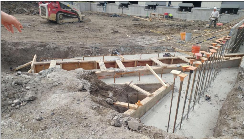
042717-4: Foundation work to avoid existing utility pipe for truck well on north side of NCMC building.
