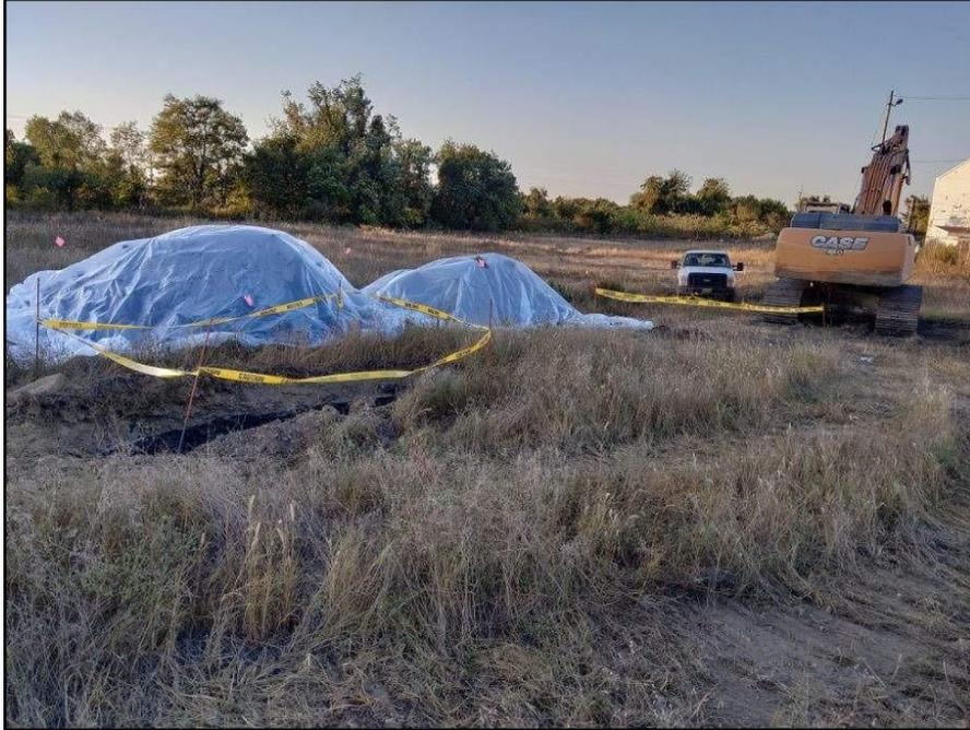
100419-5: View to the south of the completed A4 cadmium excavations and stockpiled soil.
