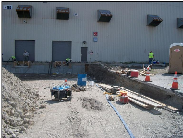
041317-1: Truck well construction on east side of NCMC building.
