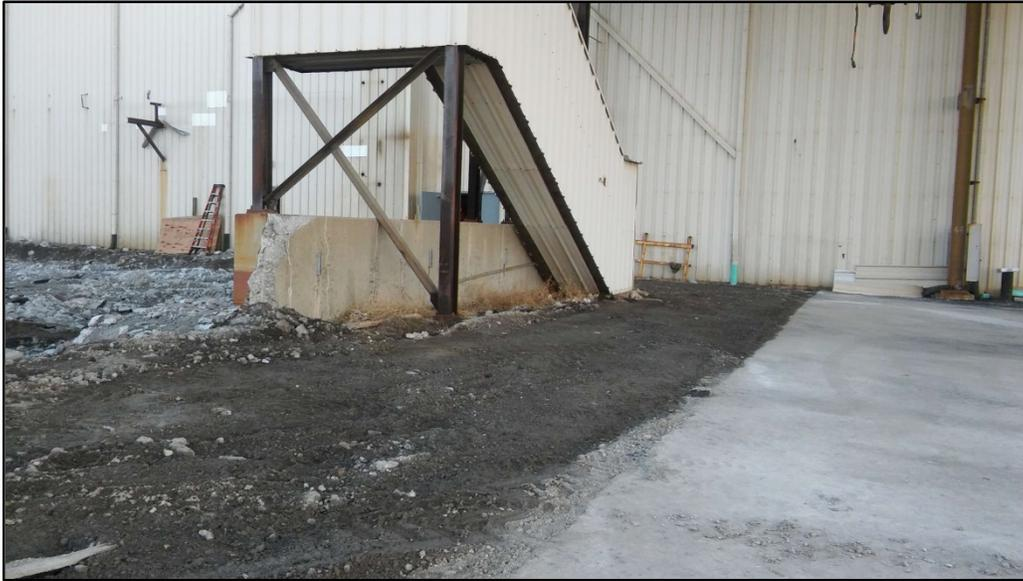
011317-1: Backfilled utility trenches on western side of NCMC building.
