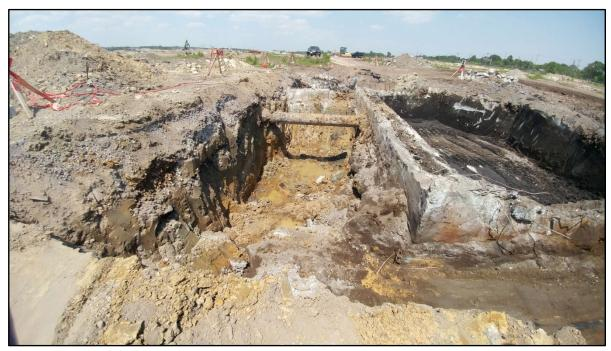
061217-1: View to the north of the western exterior trench of the excavation. A trench was dug around the concrete box to confirm if vertical and horizontal impacts from the concrete box were evident.
