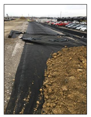
Photo 2: Placement of clean fill and marker fabric
