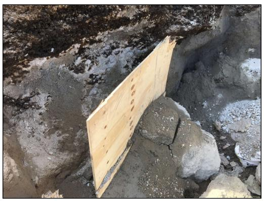
070517-1: Concrete capping, per the MDE request, of a NAPL bearing pipe encountered during excavation.
