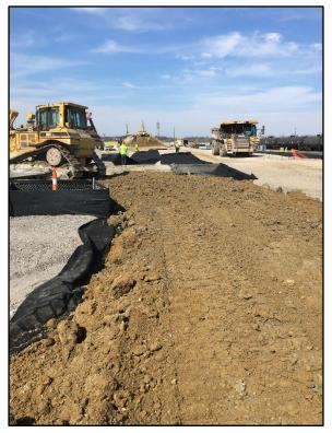
Photo 1: Placement of clean fill and marker fabric
