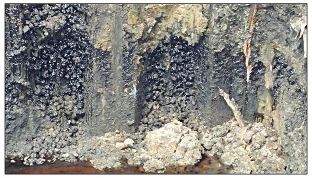
061917-1: View of NAPL encountered on excavation sidewall.
