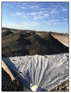
Photo 3: Impacted soils segregated and placed on plastic
