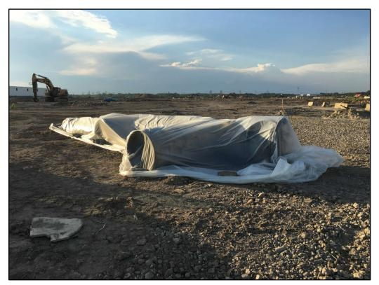
063017-1: Asbestos-wrapped pipe, wrapped in polyethylene.
