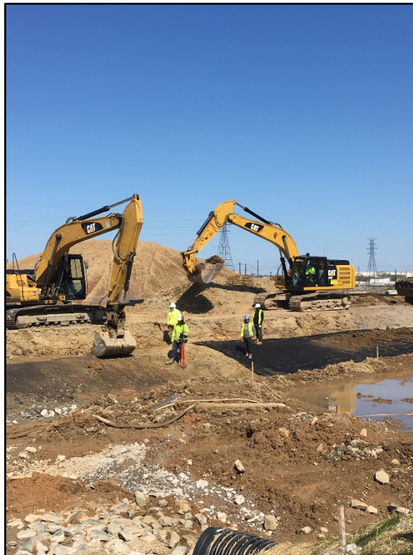
Photo 14: Sediment basin construction in progress
