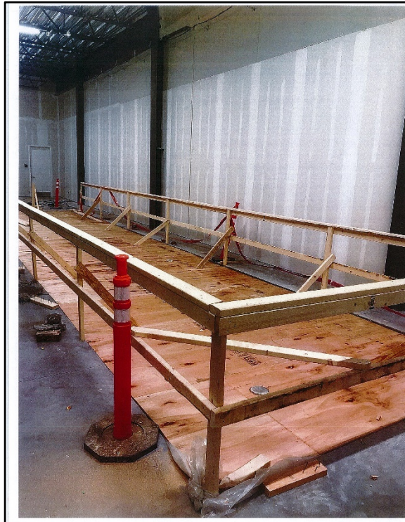
Photo 16: Implementation of agency approved interim remedy in kitchen area inside constructed building. Plastic and plywood were placed to cover the exposed surface soils. Railings prevent access to workers.
