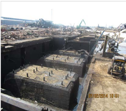
SGS #12 Machine Based Pads
