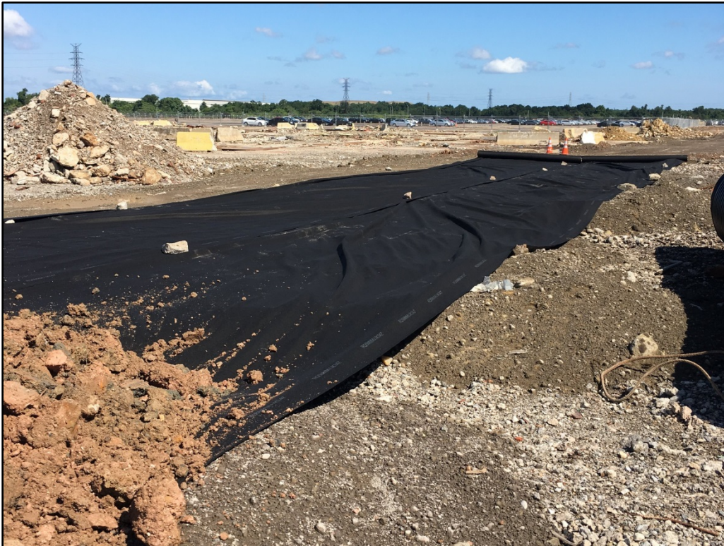
Photo 12: Placing marker fabric and clean fill in landscaped areas
