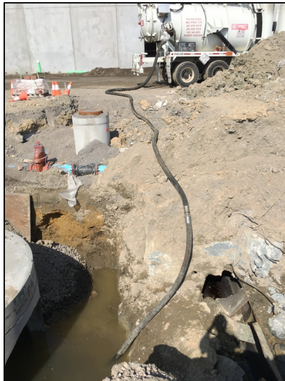
Photo 10: Pumping water from excavation during 5/16/17 event
