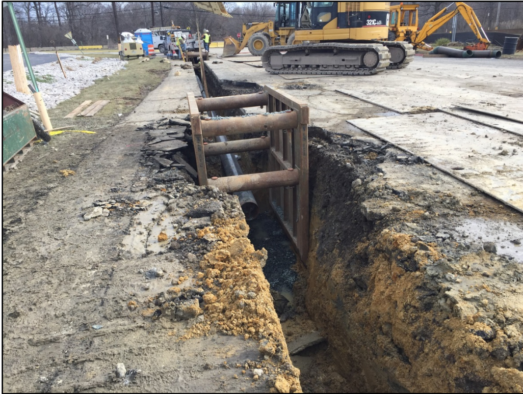
Photo 9: Typical utility installation along Tradepoint Avenue (Road and Utility work)
