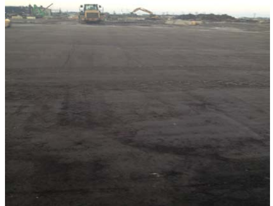
SGS#1 – Structural Backfill Complete
