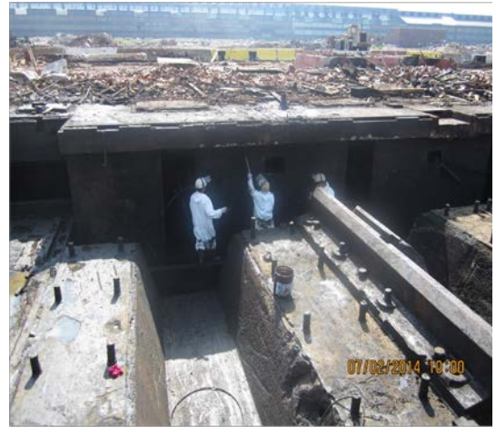
SGS #12 C&W Construction Pit Decon
