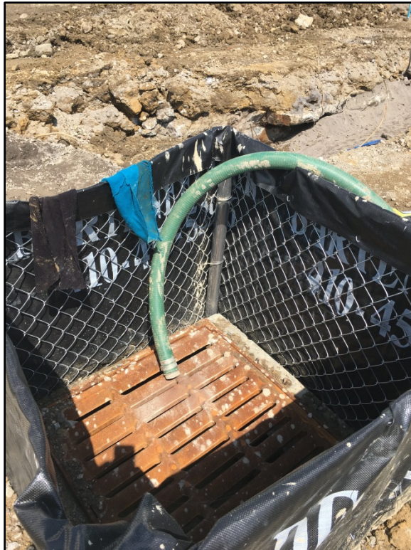
Photo 8: Dewatering that conveyed water to treatment facility
