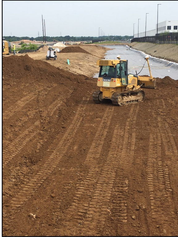
Photo 15: Sediment basin construction in progress
