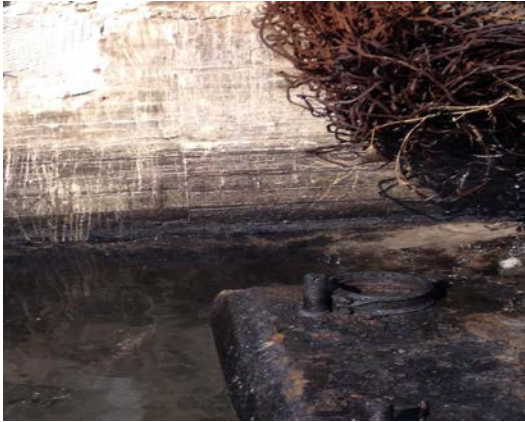
SGS#6 & 7– Concrete Scouring
