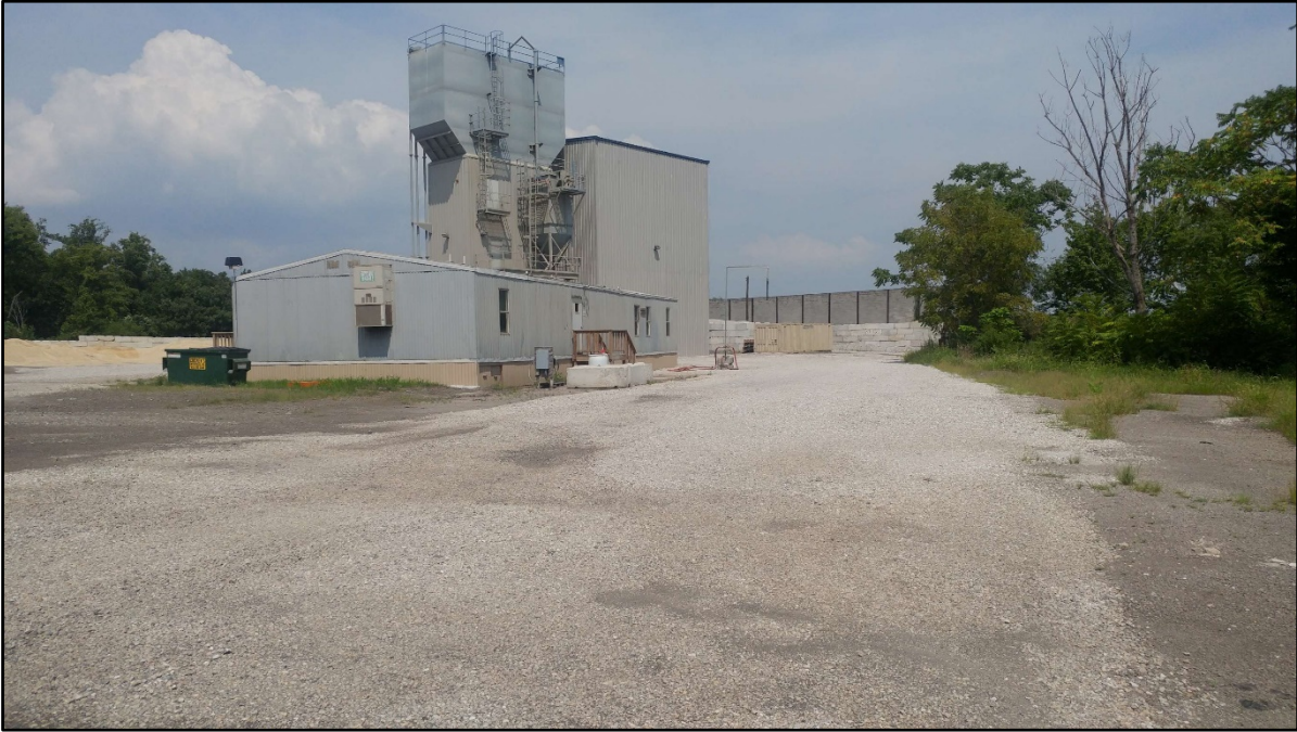
081618-1: Concrete plant in center of site.
