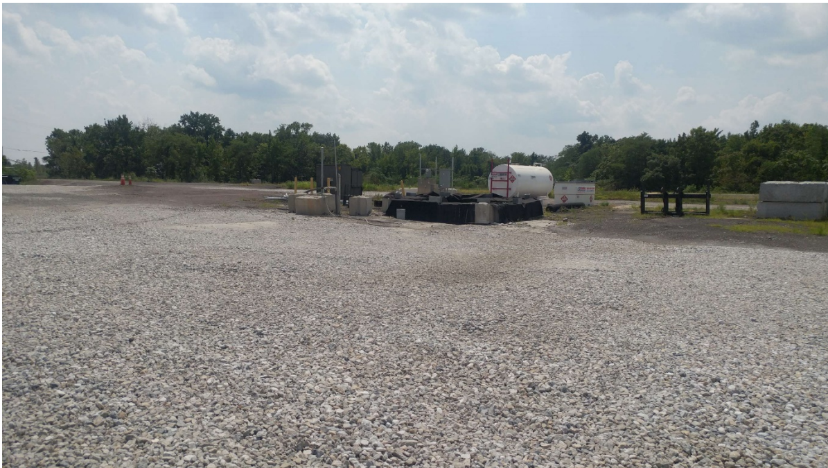
081618-4 : Electrical transformer on concrete pad.
