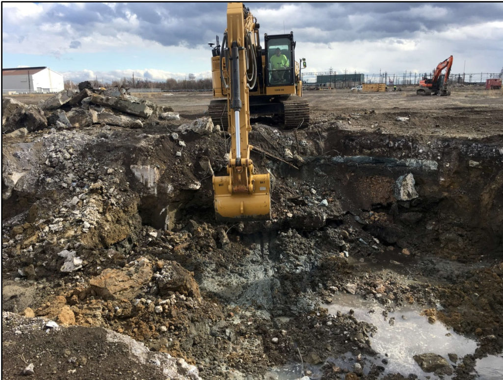
031017-1: View of removal of impacted material from excavation extension.
