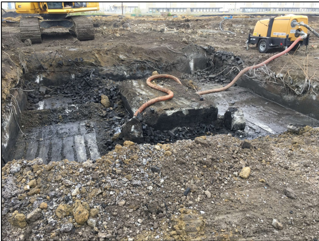
042117-2: Excavation in progress. Take note of the NAPL stained concrete box.
