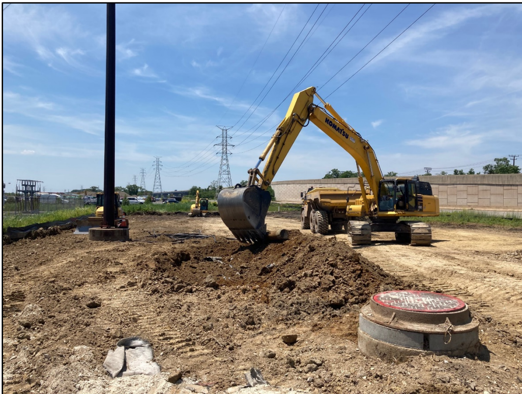
060920-2: Cutting around the electrical manhole and a monopole electrical tower north of the substation.
