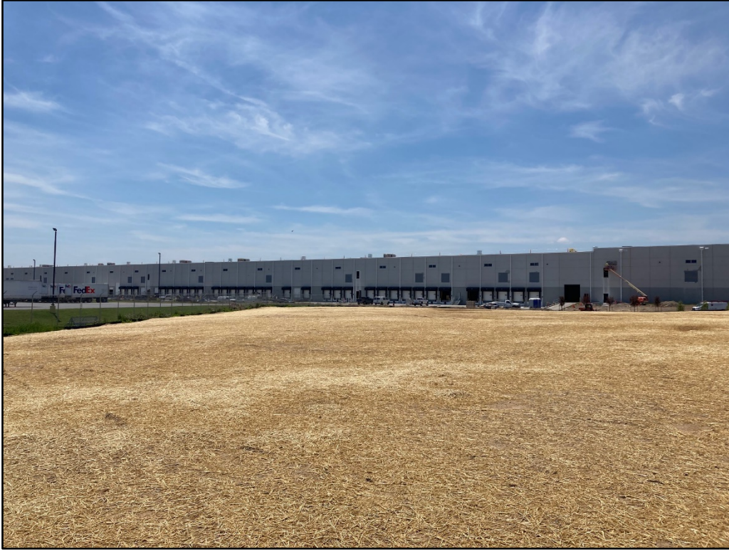
060920-1: Seeding and stabilization in place following the completion of filling and grading in the south of the substation.
