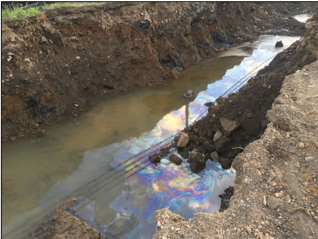
050217-1: View to the north of the RW-003 Response Area with oily sheen on accumulated groundwater.
