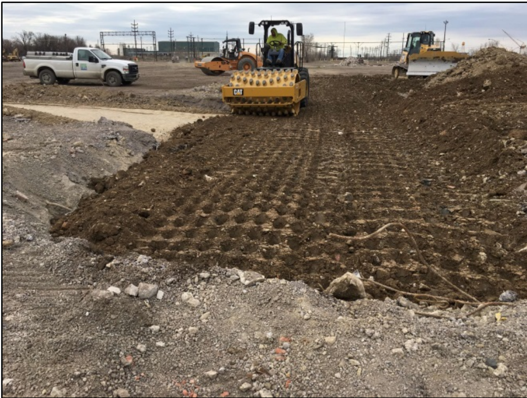
023017-1: View to the south of backfilling in progress.
