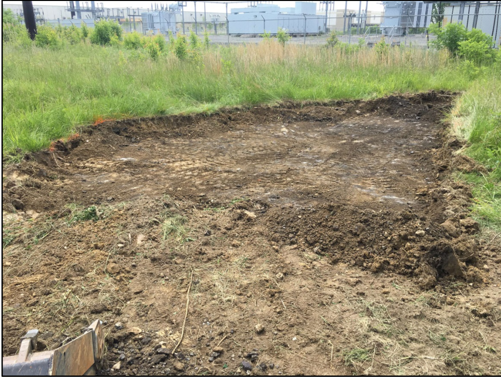
051817-3: RW-004 Excavation – facing south. Excavation to 1 foot below ground surface (bgs).
