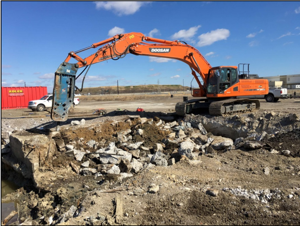
030217-1: Excavator with hammer attachment used to break up and remove NAPL stained concrete floors, walls, footers, and boxes.
