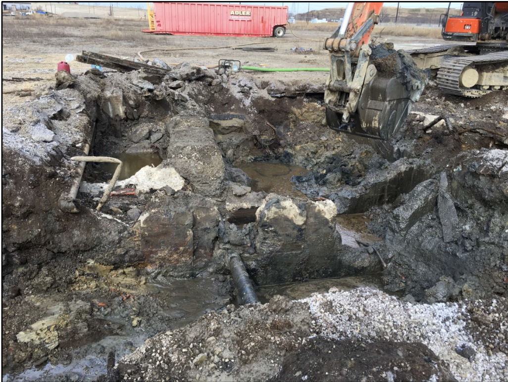
022117-1: Excavation in progress. Visible in background is an Adler tank used as a temporary storage unit to dewater the excavation.
