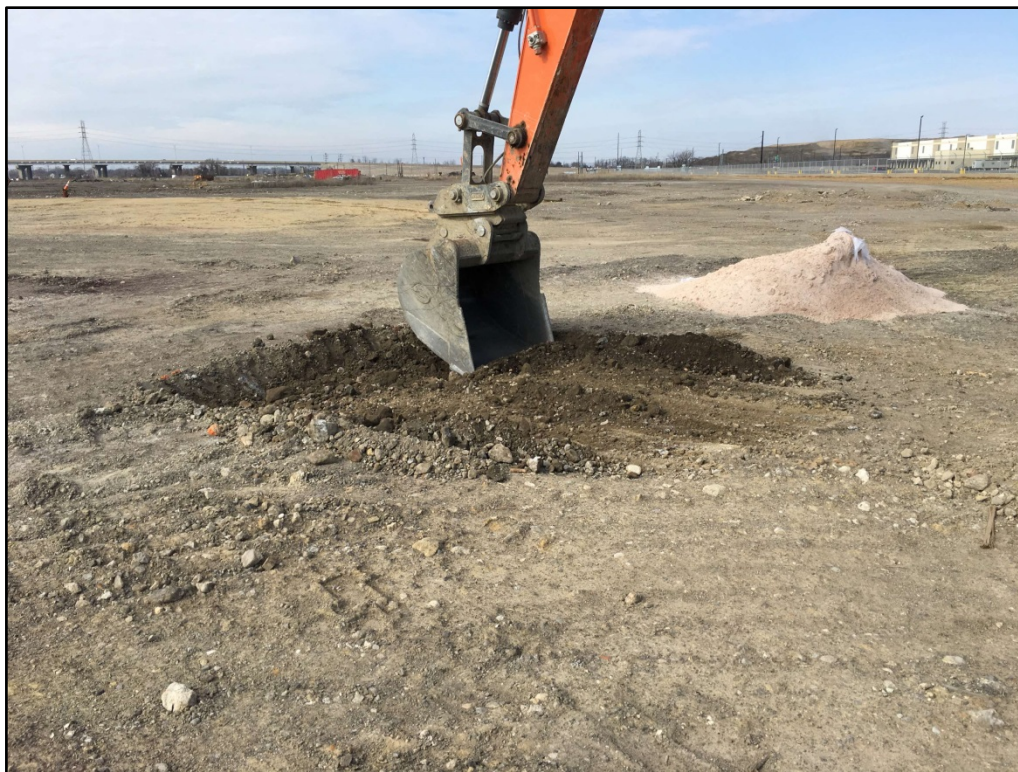
030617-1: RW-021 Excavation – View to the north of initial excavation activities. Visible to the northeast of the excavator bucket is Terrabond material for mixing with excavated soils.
