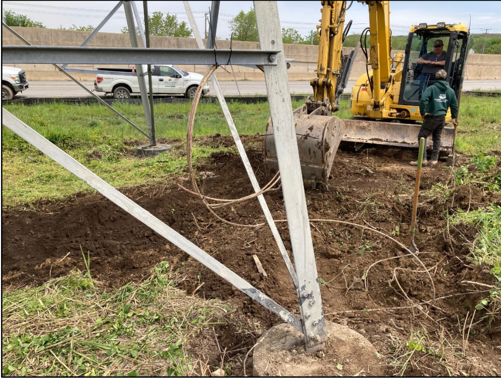
050520-1: Grounding cables exposed just below the surface while cutting around the electrical tower in the northern capping area. Cables were replaced by BGE contractors prior to filling in the area.
