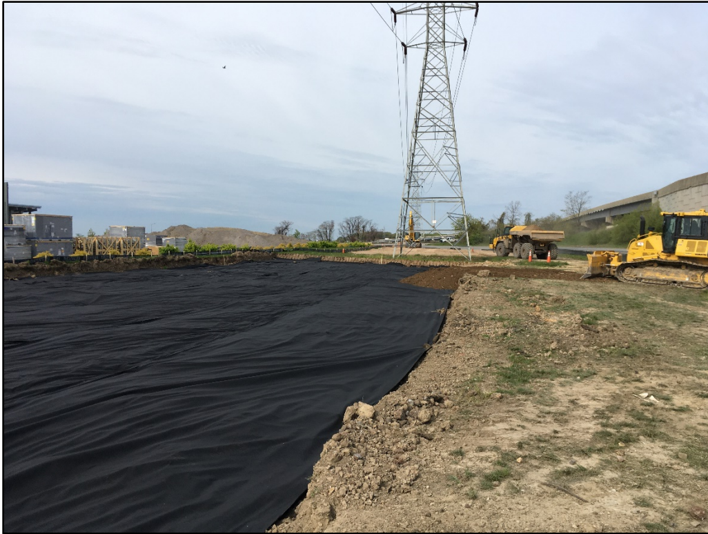
042320-1: Placing clean fill material in the northwestern capping area.
