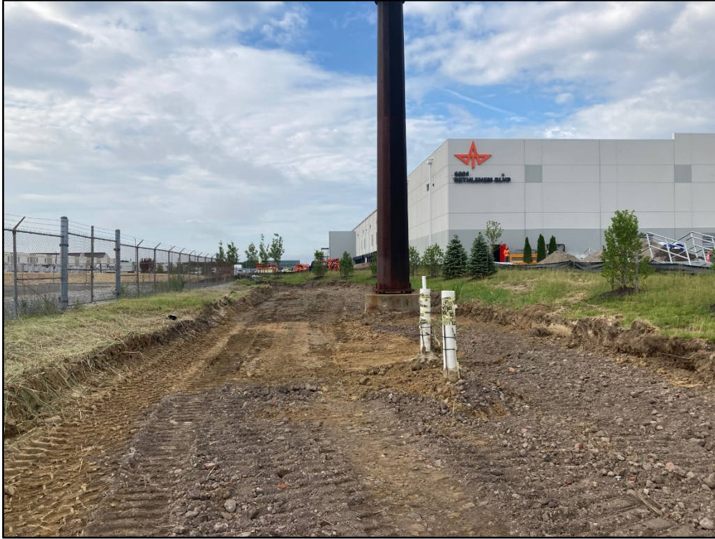
061920-1: Area west of the substation excavated around a monopole electrical tower and a monitoring well pair.
