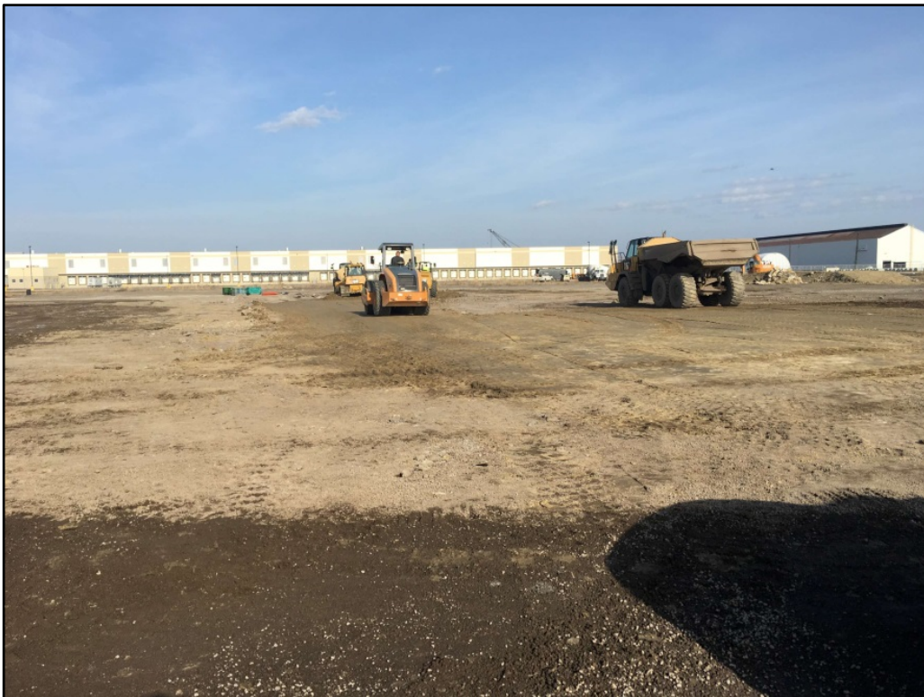
032717-1: View to the east of the RW-029 Response Area backfilled to grade.
