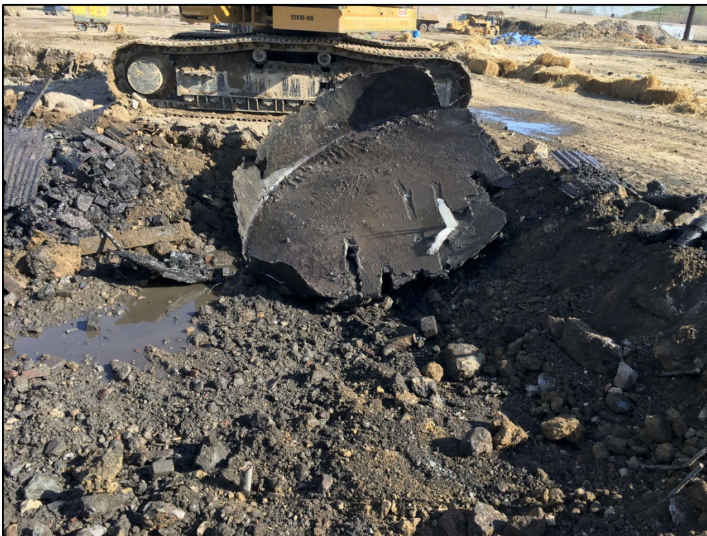
041917-1: View of bottom fragments of a fiberglass tank. Soil impacts were observed around the location of this along with four other tanks of similar size in the same vicinity. Tanks were located on the concrete pad.
