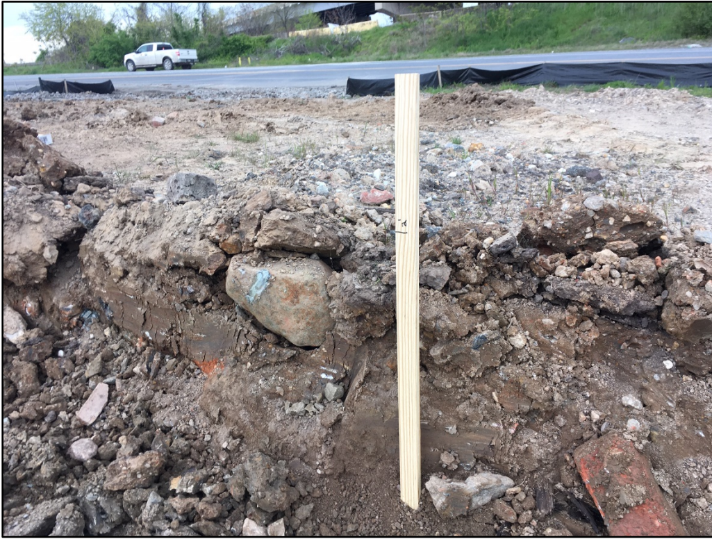
042020-1: Grading stakes used to measure clean fill depth.
