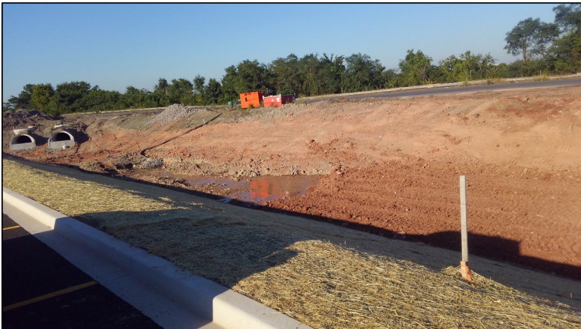
Photo 2: Placement of clay in basin
