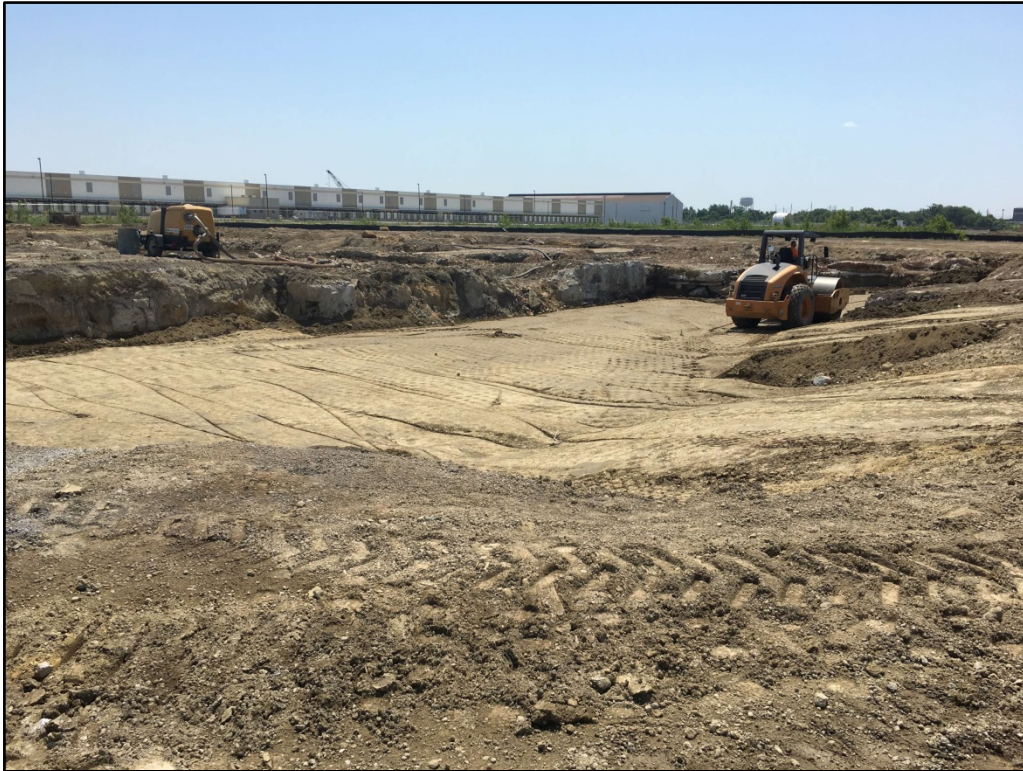
051917-1: View to the southeast of backfilling in progress
