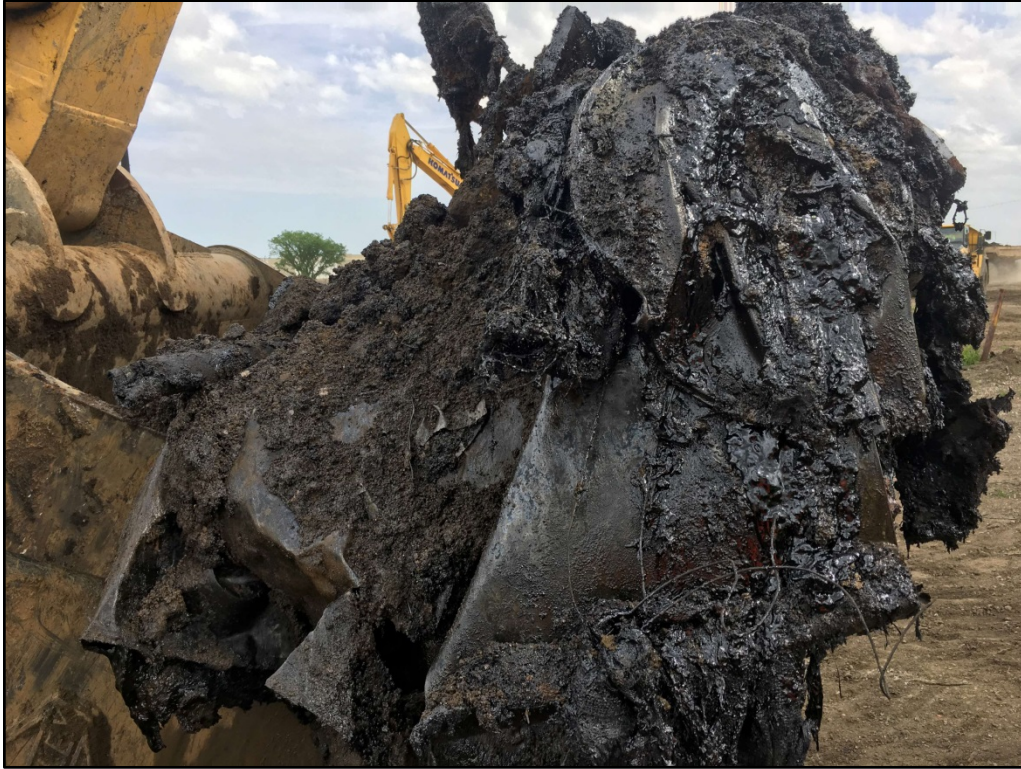
050117-3: Fragments of steel drums saturated in NAPL from the RW-003 Response Area.
