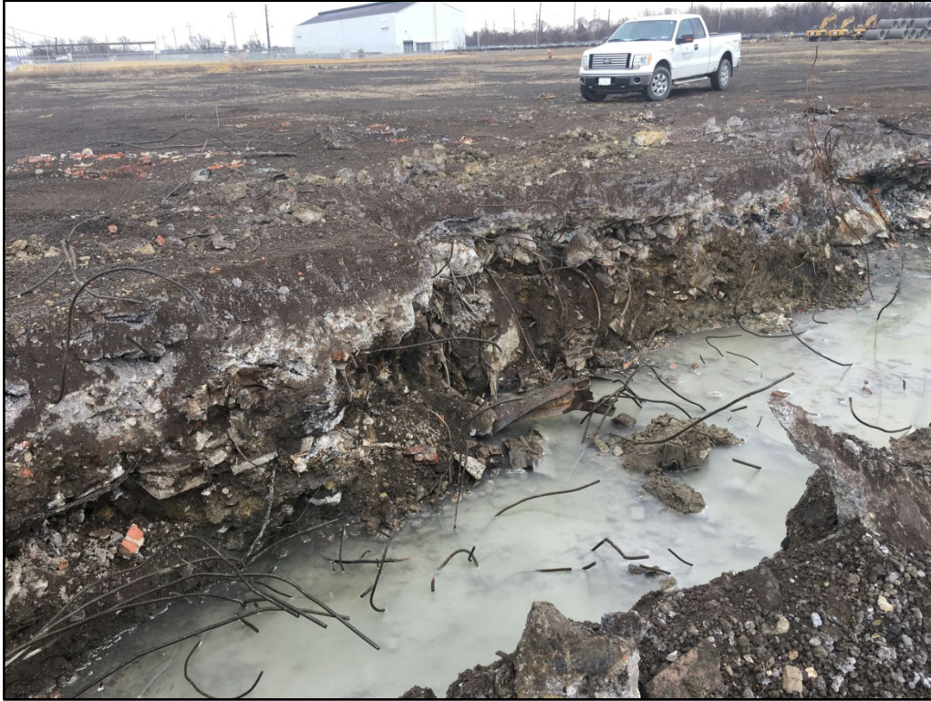
030717-1: View to the southeast of the RW-041 Response Area. Take note of the backfill debris along the east sidewall; this backfill material was common throughout the entire excavation.
