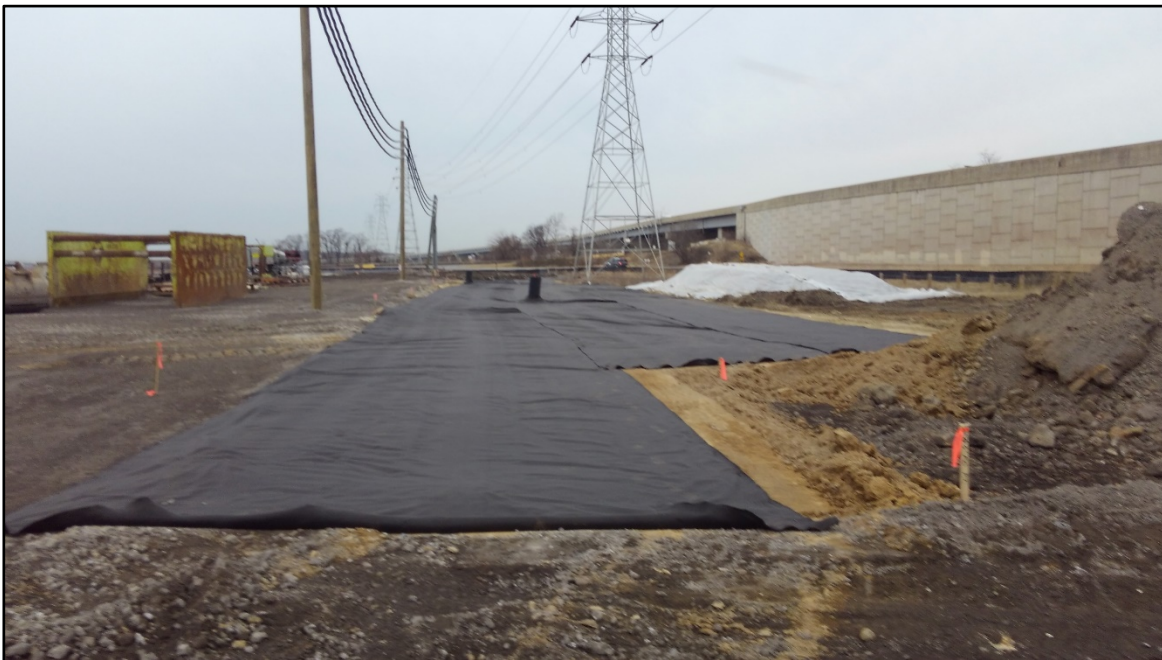
Photo 8: Placement of fabric in northern portion of Site
