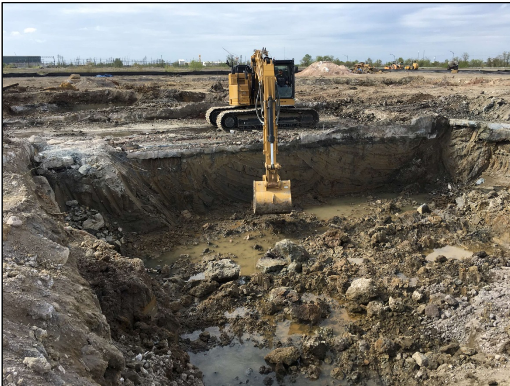
042017-1: View to the south of concrete pad encountered during excavation activities. This concrete pad was not removed due to no impacts beneath.
