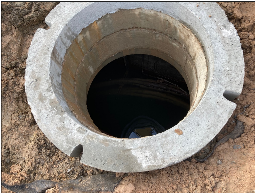
042320-2: 6" concrete collar placed around an electrical manhole in the northwestern capping area.
