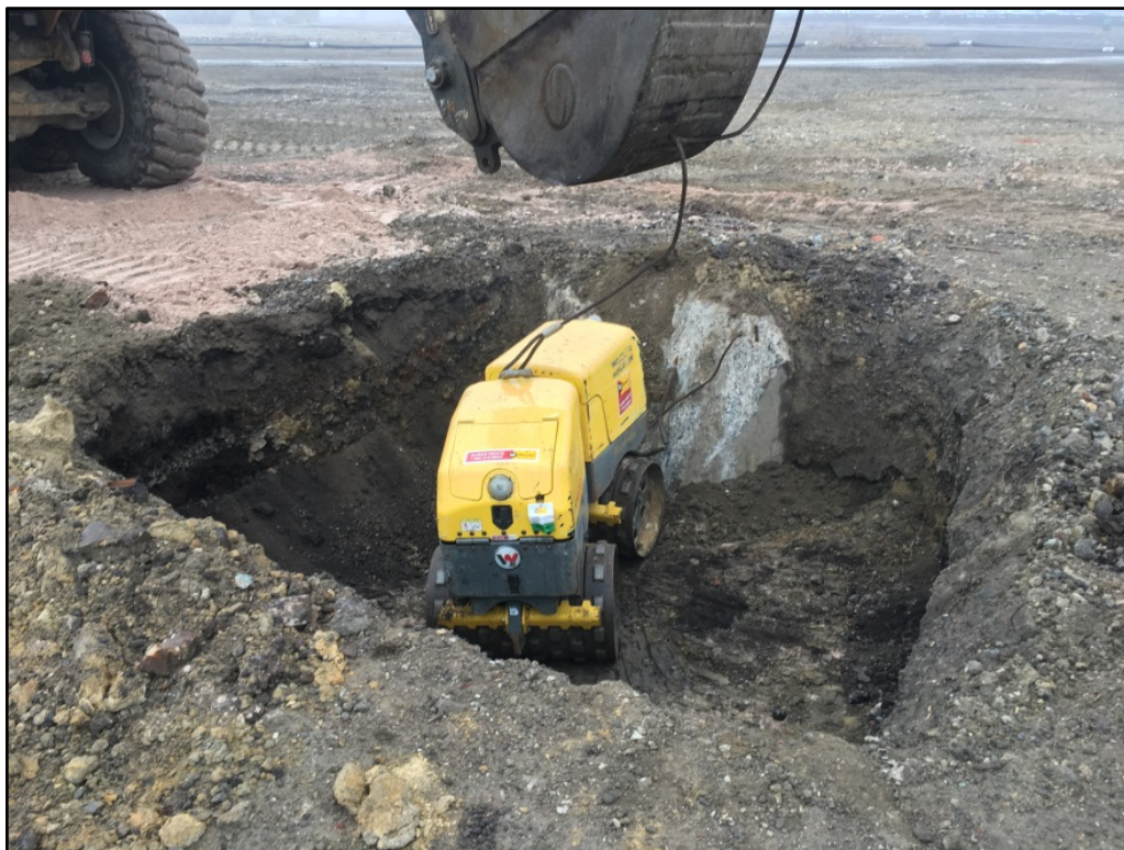
032717-1: RW-021 Excavation – Backfilling and compaction in progress
