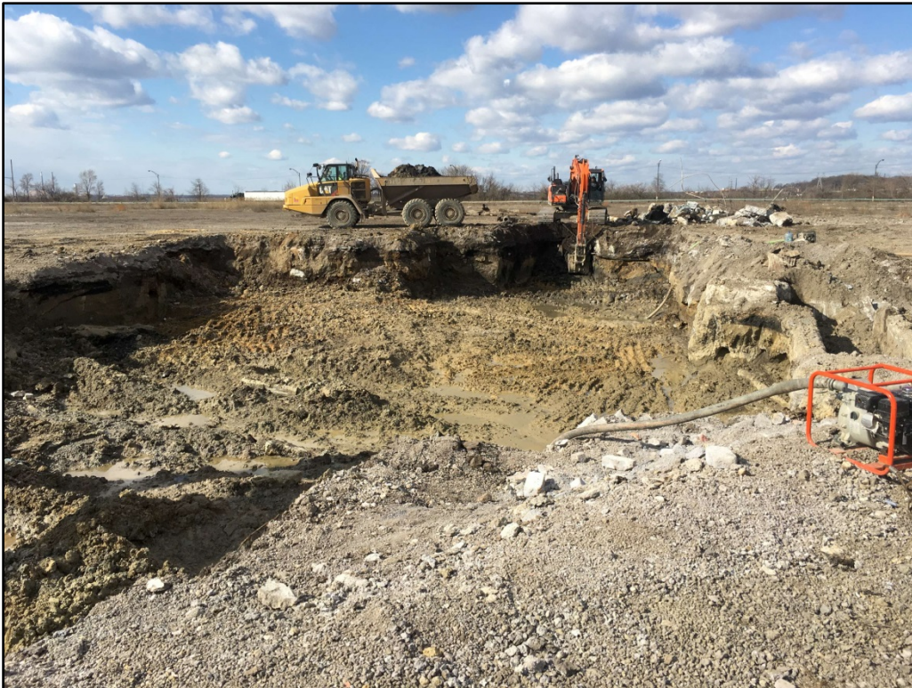
030317-1: An Oil & Grease exceedance was identified along the west wall where the excavator is located; this area was extended.
