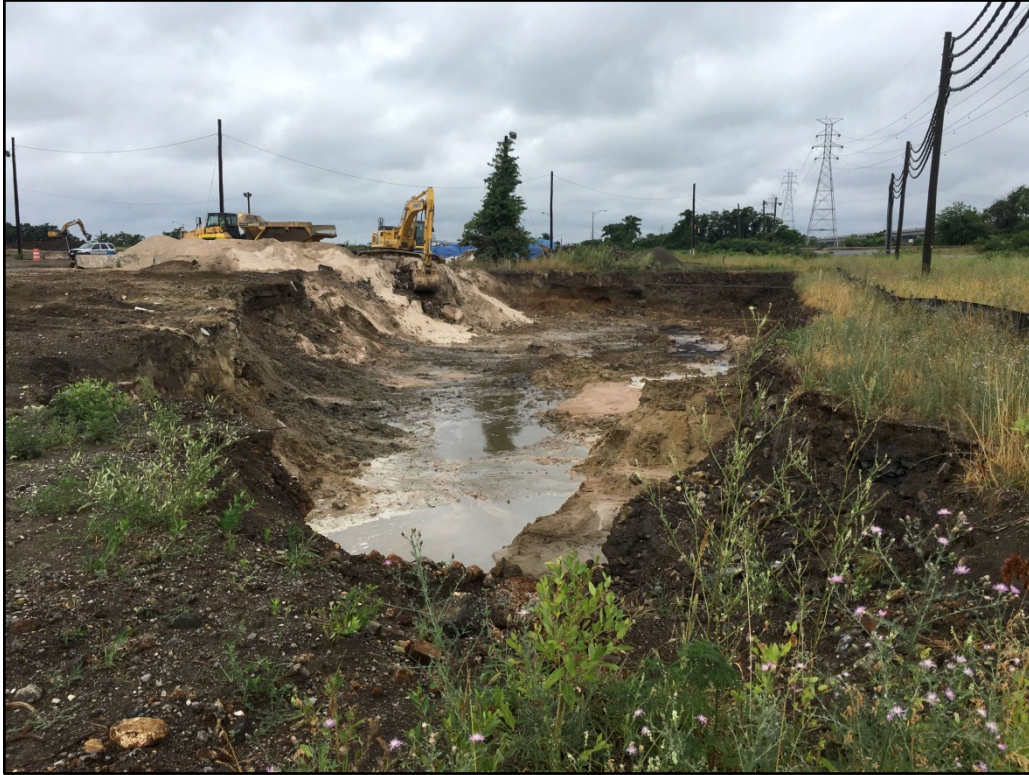
070617-1: View to the west of excavation and mixing with Terrabond in progress.
