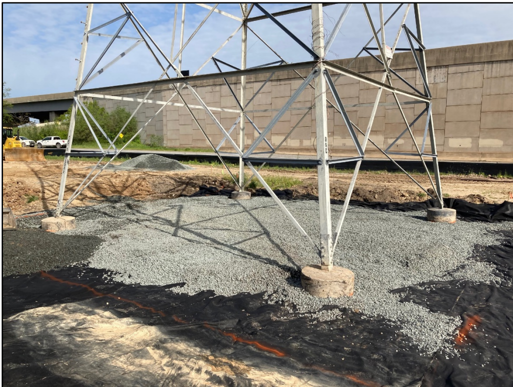
Photo 12: Geotextile marker fabric and #57 stone placed around the footprint of the electrical tower.
