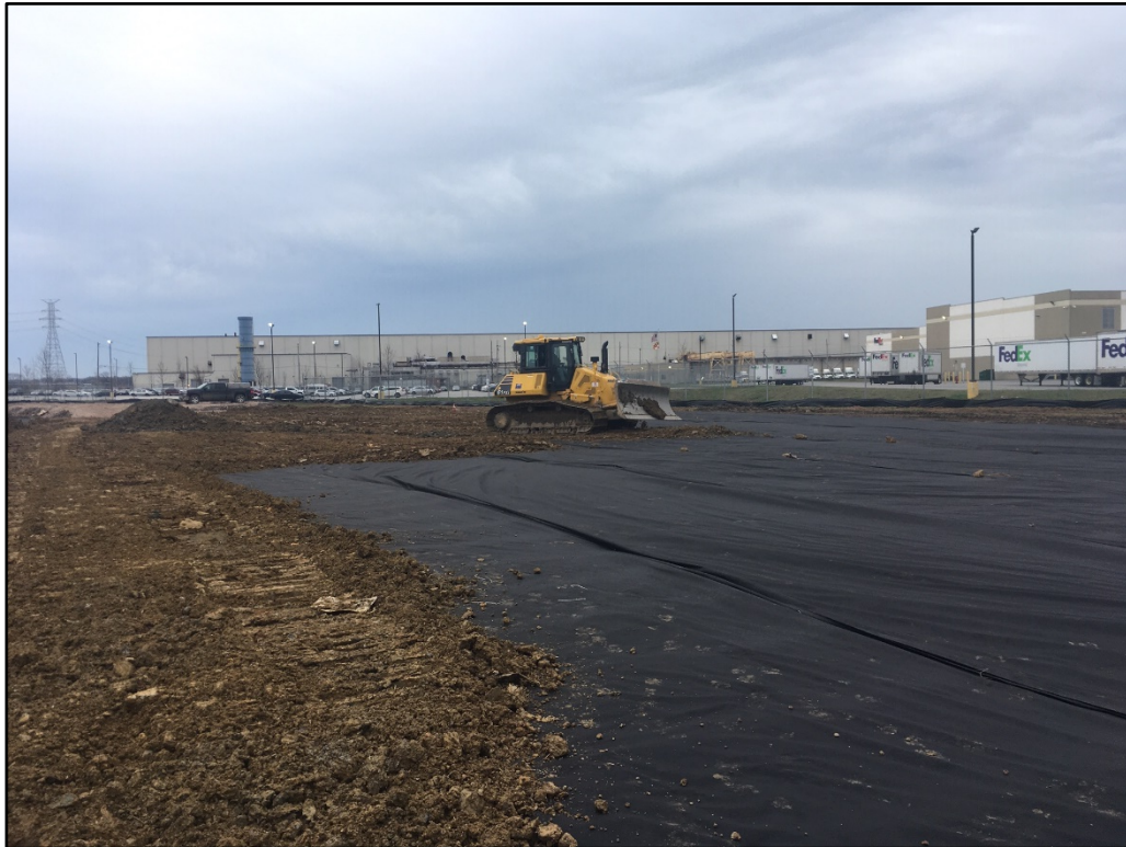
032320-1: Placing and grading clean fill material.
