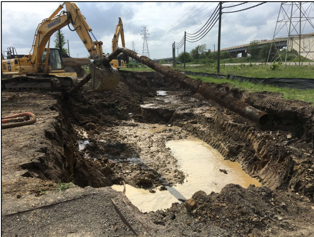
050117-2: View to the west of excavation in progress. An empty corroded utility pipe was found and removed.
