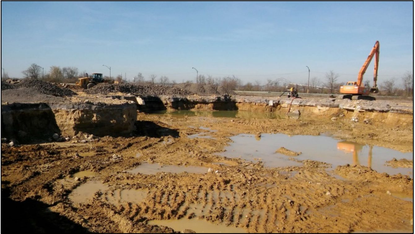
041017-3: View to the west of dewatering the excavation prior to backfilling.
