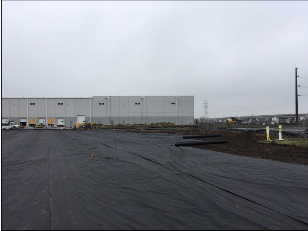
032020-1: Placing geotextile marker fabric over the portion of the site south of the substation following the completion of rough grading.
