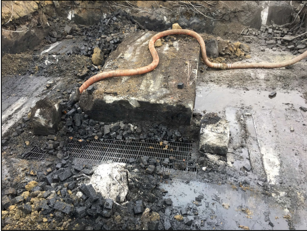
042217-1: Trench drains located around the raised concrete box.
