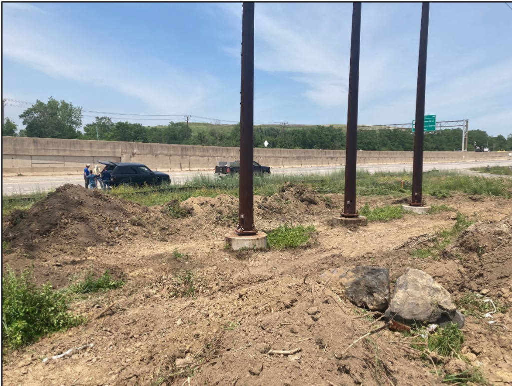
060420-1: Cutting around the three monopole towers in the northern capping area.
