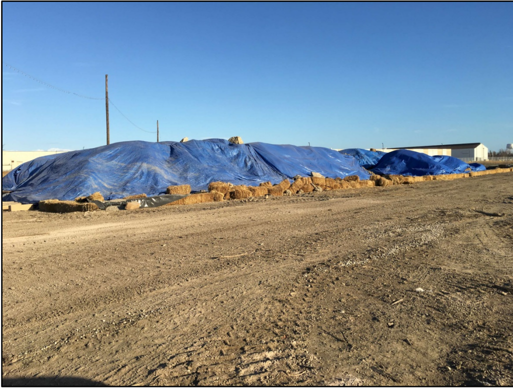
022417-1: Soil waste stockpile contained and covered with plastic.
