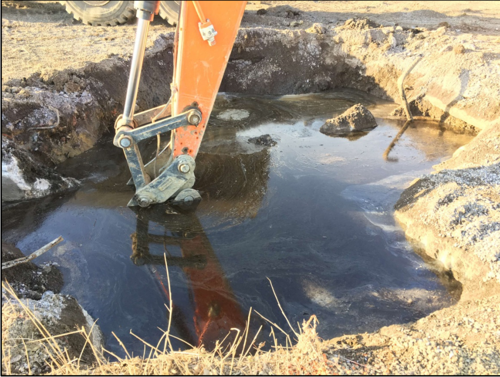
022017-1: NAPL observed in the groundwater during excavation activities.
