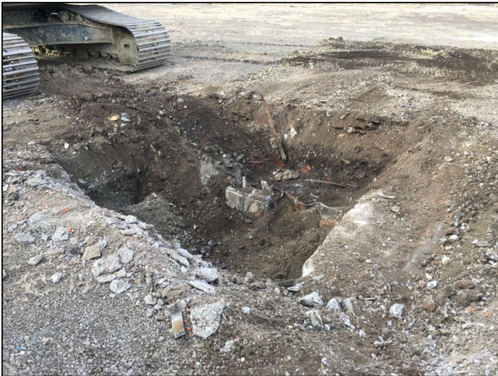
021617-4: Completed excavation. Little to none impacts were observed.
