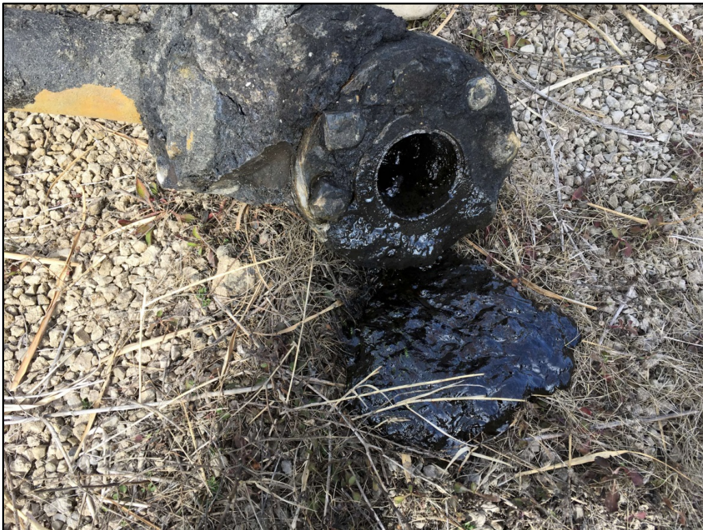
021717-2: A NAPL bearing pipe was observed and removed from the excavation.
