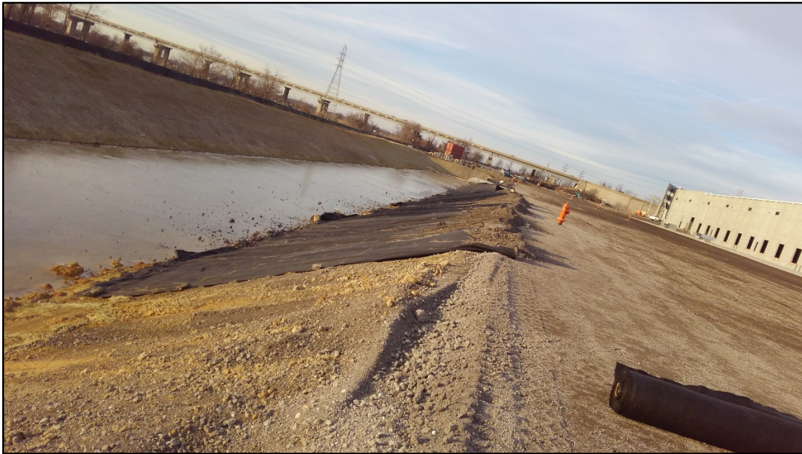
Photo 3: Placement of fabric in basin
