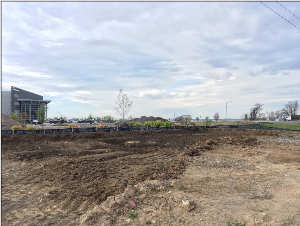
042020-2: Cutting in the northwestern section of the capping area to approximately 18" below the initial grade.
