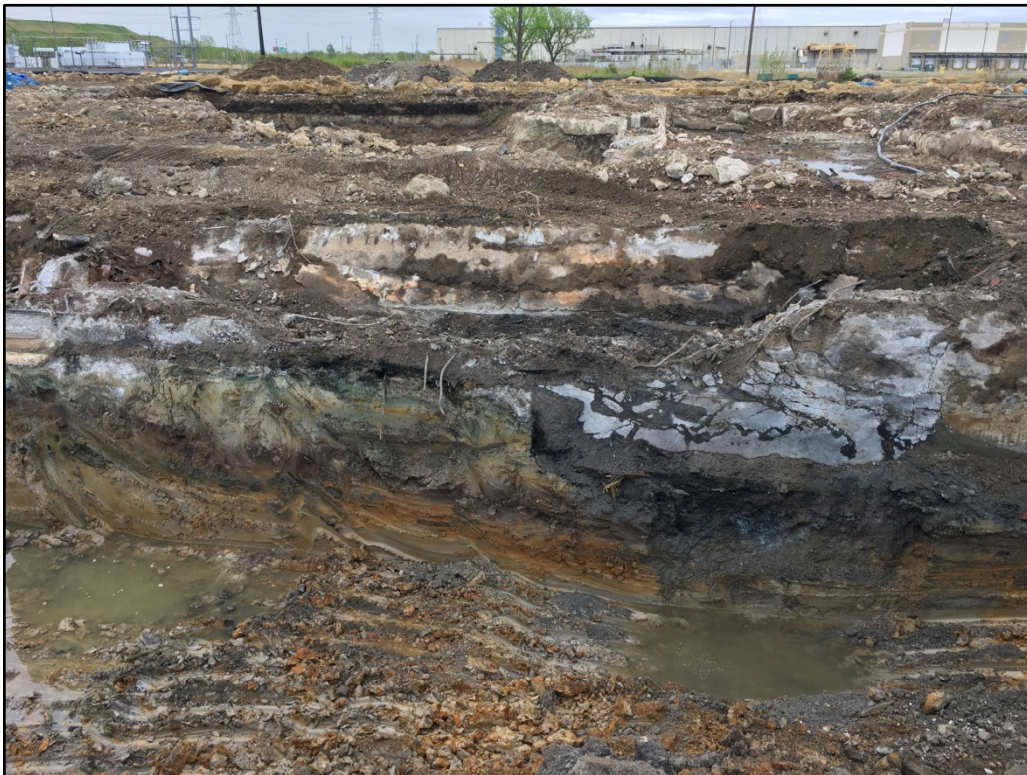
042417-1: View to the east of open face concrete structure with impacted soil underneath.
