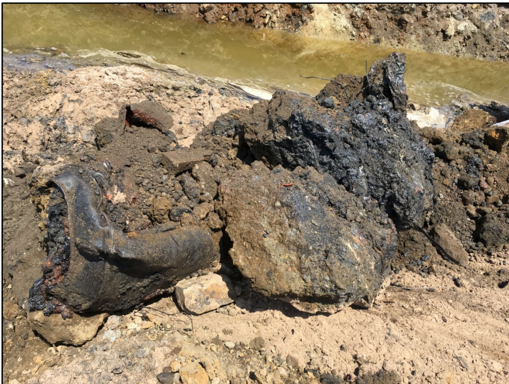
051817-1: Fragments of steel drums and large sections of slag material that were excavated from the RW-003 Response Area.
