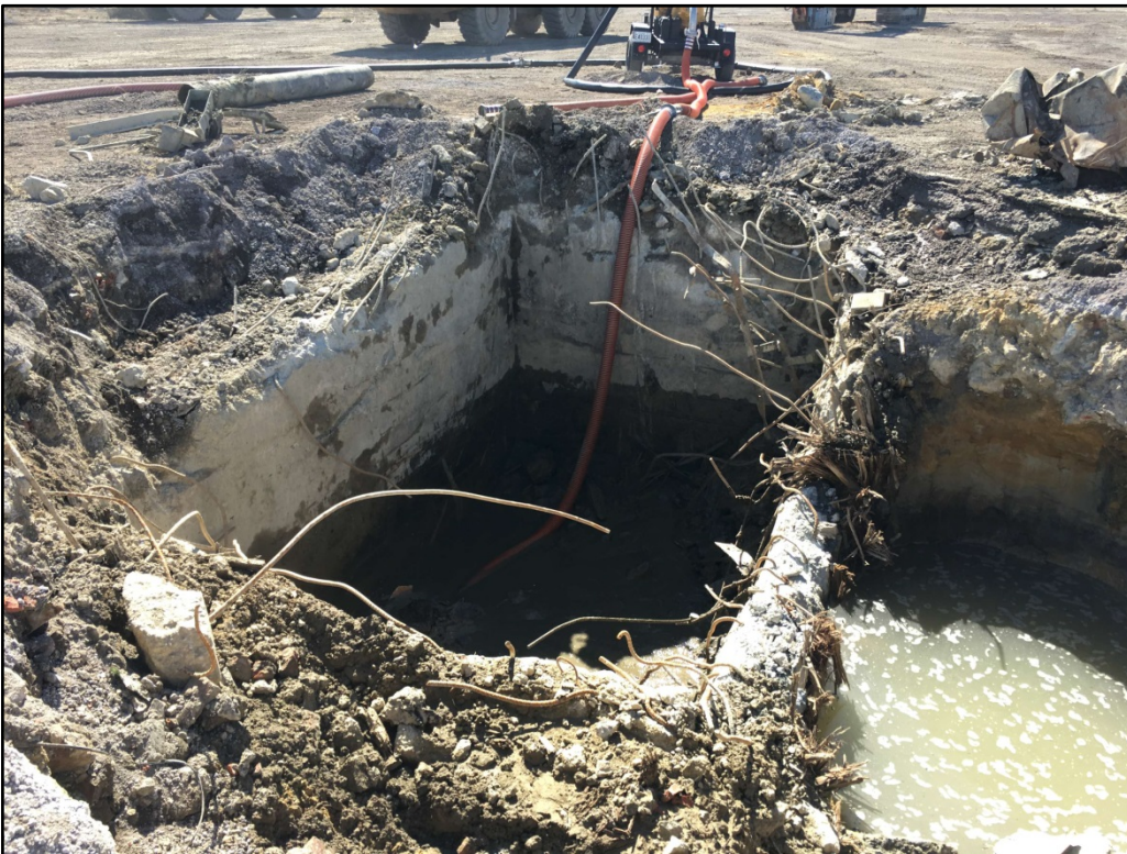
032917-1: View of dewatering completed excavation for backfilling. Concrete boxes were not NAPL stained.
