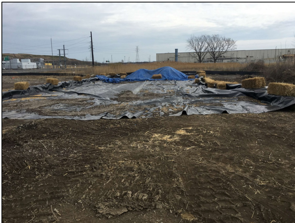
030617-2: RW-021 Excavation – Excavated soils stockpile staging area
