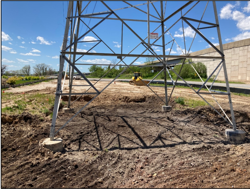
050420-1: Cutting material around the footprint of the large electrical tower in the northwestern capping area.
