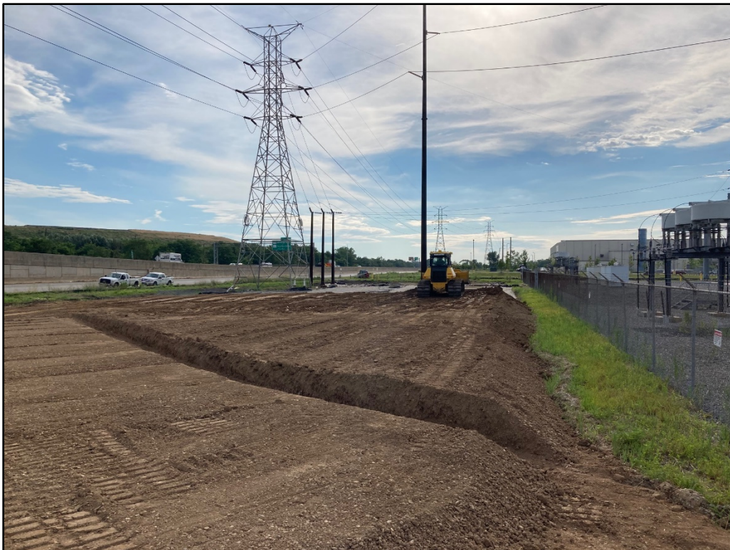
071320-1: New drainage swale stretching from the northwest corner of the substation to a stormwater inlet adjacent to Bethlehem Boulevard.
