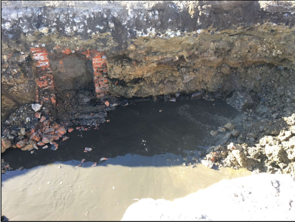
030917-1: Extension of excavation in progress. NAPL saturated soil removed in and around brick box.
