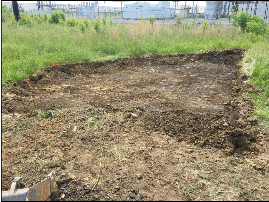
051817-3: View to the south. of excavation to 1 foot below ground surface (bgs).
