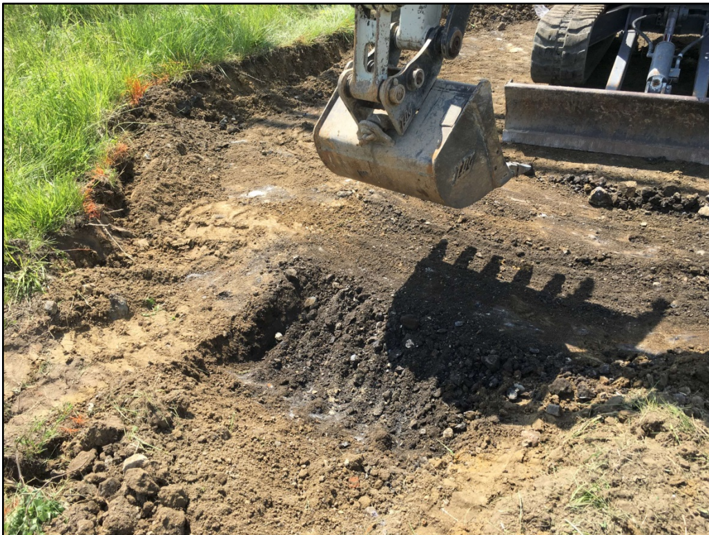
051817-4: Close-up view of excavation attempt below 1 foot bgs.
