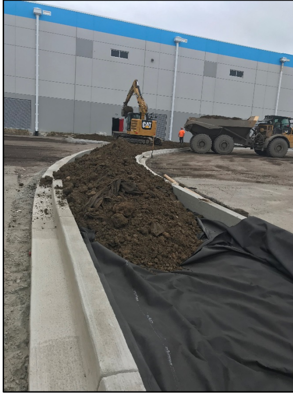
Photo 9: Placement of fabric and clean fill
