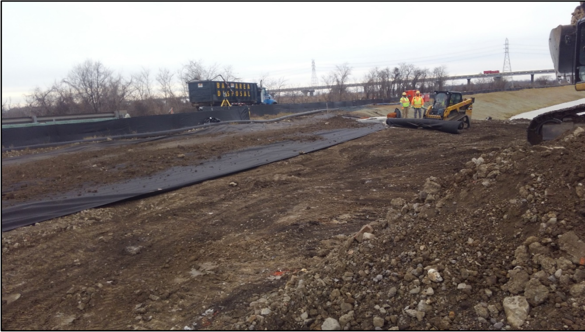
Photo 7: Placement of fabric in western portion of Site
