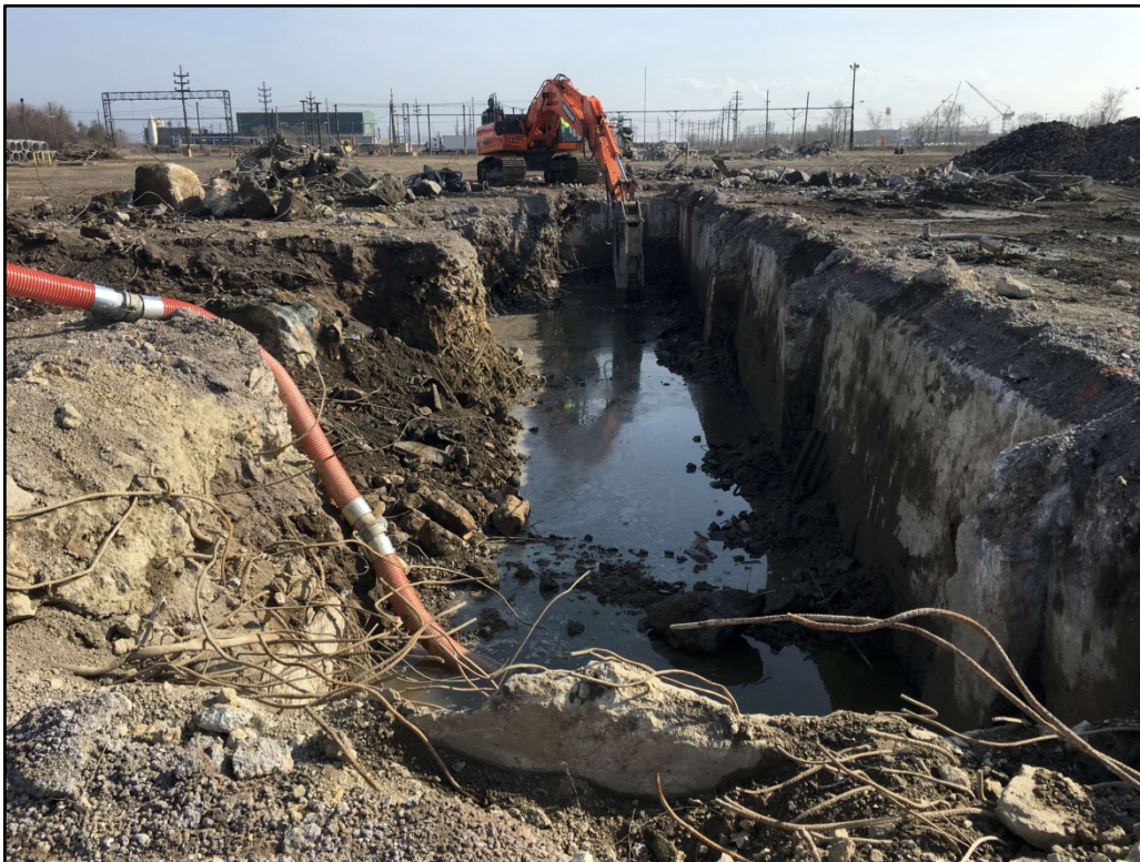
032717-1: View to the south of excavation in progress. The excavator with a hammer attachment can be observed making holes along the concrete bottom of this excavation. Take note that the west sidewall is concrete.
