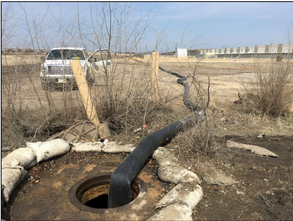
032417-2: Dewatering discharge to existing manhole. Water was conveyed to Tradepoint Atlantic's on-site wastewater treatment plant.
