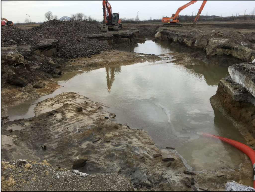
032417-1: Backfilling excavation in progress. Visible in bottom-right corner is dewatering hose.
