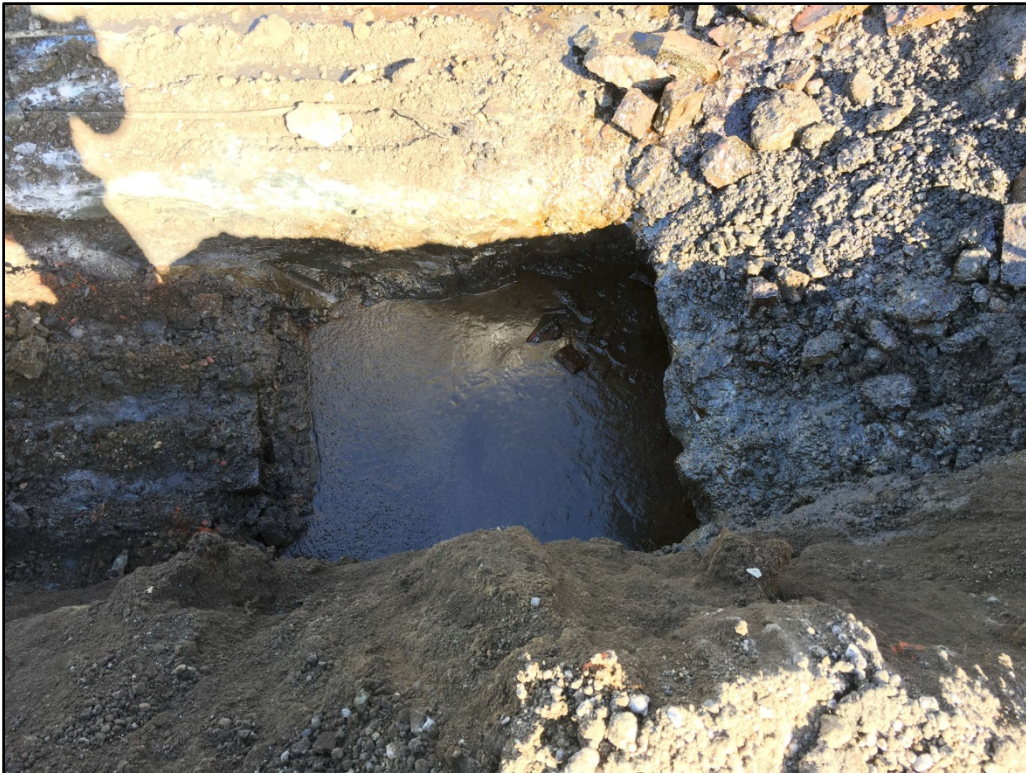
022417-2: View of concrete box filled with black NAPL located along the southeast corner of the excavation.
