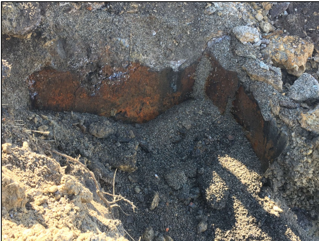
031617-1: View of a metallic tank located along the southeast corner of the excavation. Black NAPL impacted soil was observed in and around the tank.
