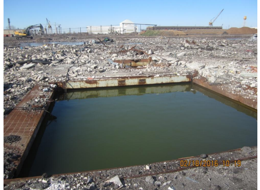
SGS-54 Freight & Passenger Elevator Pits
