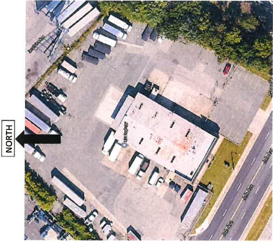
Google Earth view shows building after the fire and before renovations. Note holes in roof that has since been repaired. The temporary office trailer on the front lawn is no longer on the premises.
