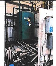
Photo H6: Tank #642 used for the storage of PCB wastes 50-499 ppm.
