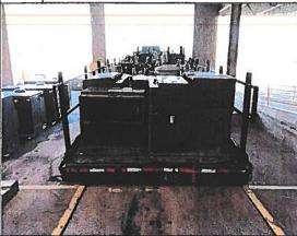
Photo Transformers drained and loaded onto #17: transport for disposal.
