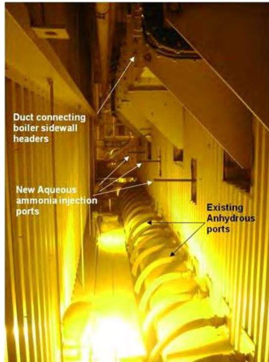
**Figure 3. Tertiary Air Front Wall Duct**
