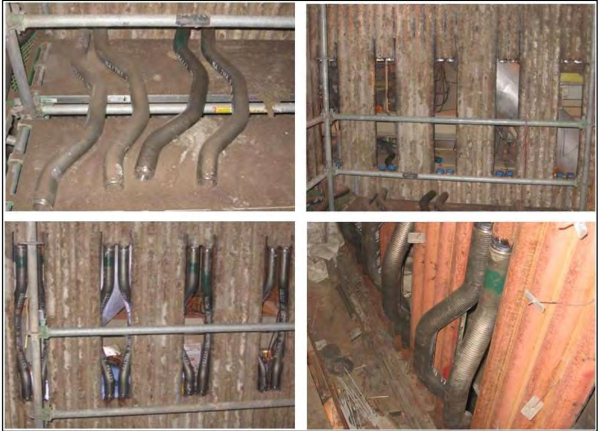
**Figure 4. Waterwall Tube Modifications for Tertiary Air Nozzles**
