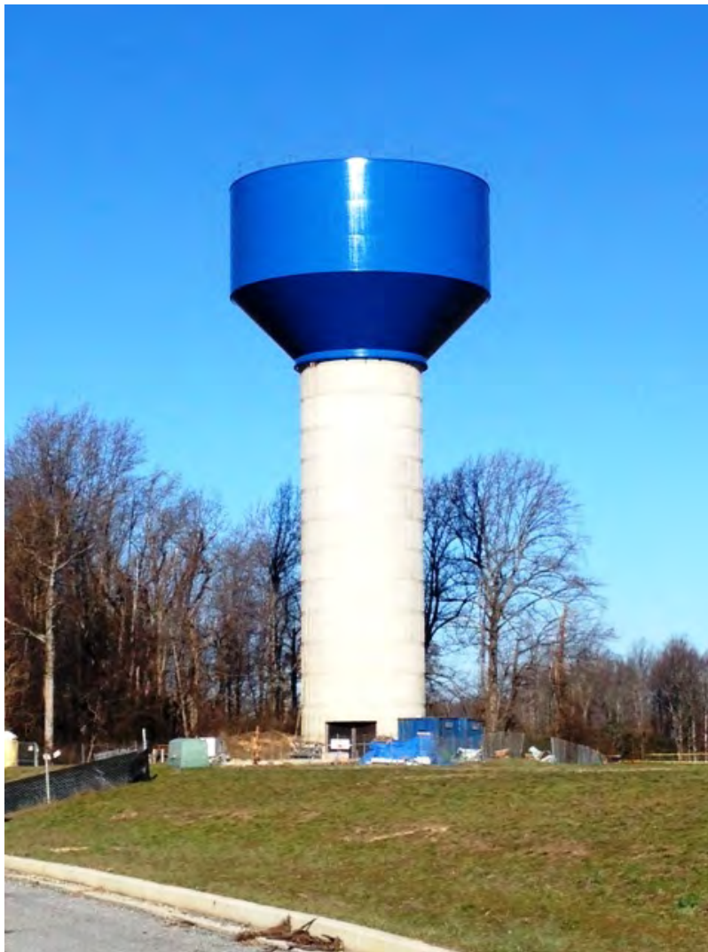
East Prince Frederick Elevated Storage Tank
