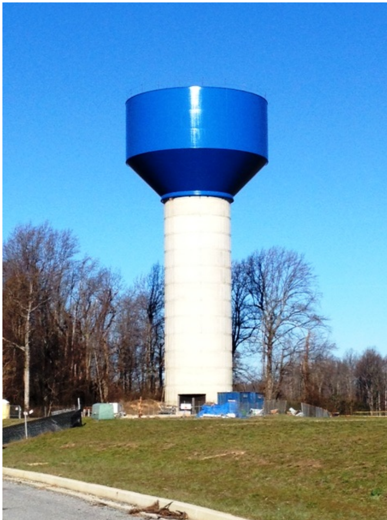
East Prince Frederick Elevated Storage Tank
