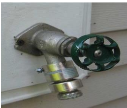
Hose bib with BFP; water supply is protected from contamination when a hose is connected.
