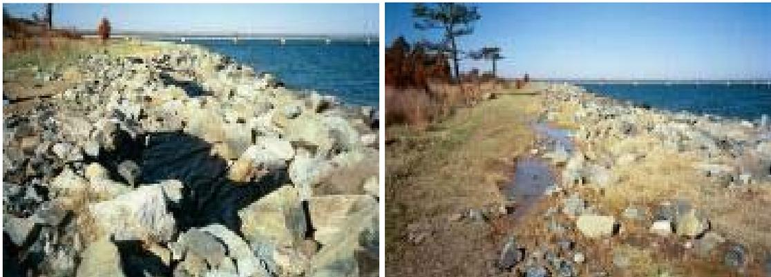
**Figs 26 and 27.** Failed revetments showing open area where rocks have shifted. (Photos: Maryland Department of Natural Resources)
