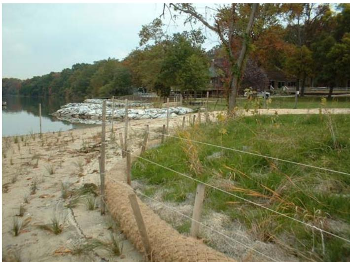
**Fig. 8. Fiber logs provide temporary stabilization for a newly created marsh. A fence prevents waterfowl from eating young plants.** (photo: Department of Natural Resources)
