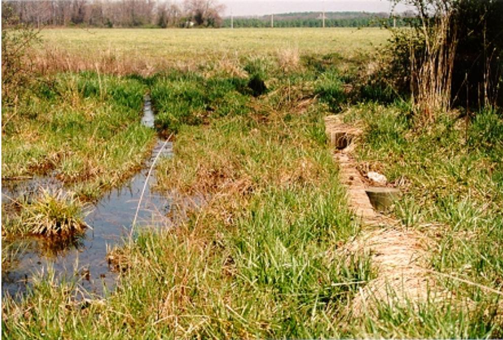
Figure G.26: Timber weir along hedgerow to control drainage (photo Noble 1/98)
