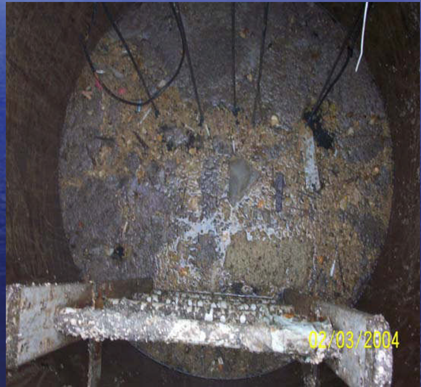
Grease accumulation in a Sewer Pump Station.
