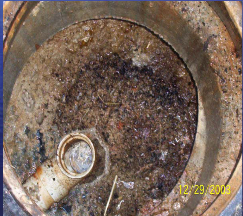
Buildup in a grease interceptor.
