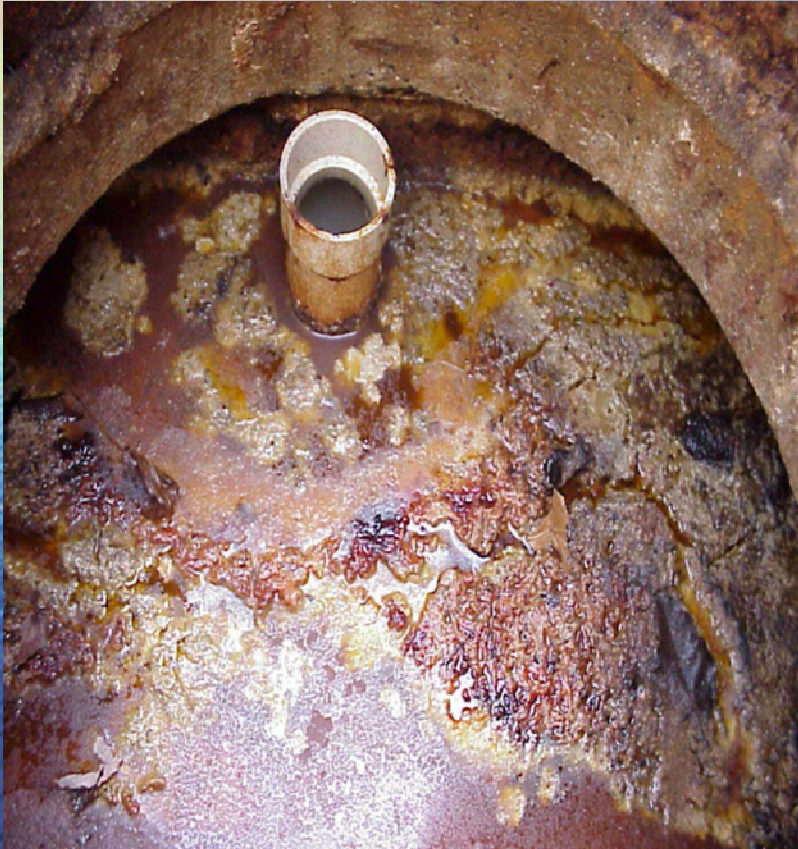
Grease needs enough time to separate from soapy water.
