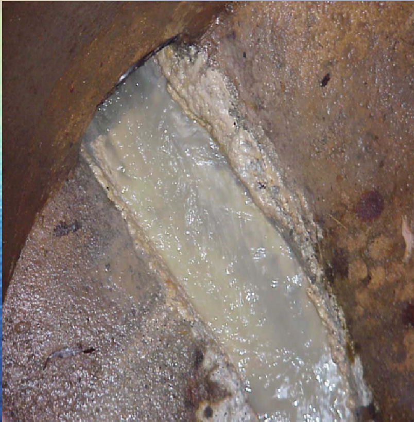
Fog deposits in manhole invert.
