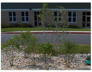
Stone prevents weed growth and erosion in this bioretention Figure 8. Examples where stone was placed as an alternative to mulch.
