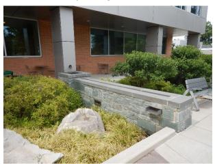
Bioretention and rooftop disconnect are designed to complement the architecture
