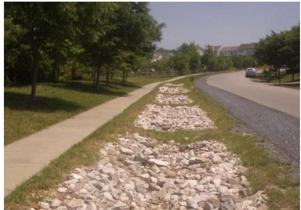
*Infiltration trench, Stormwater LLC*
