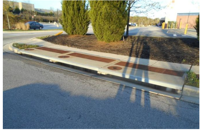
Perimeter Sand Filter
