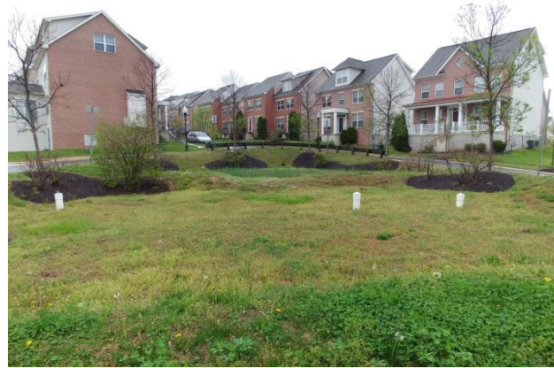
Surface sand filter with grass turf cover
