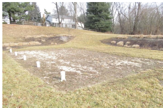
Surface sand filter
