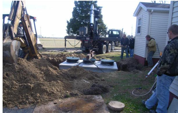
*Connection of the waste stream to a wastewater treatment plant*
