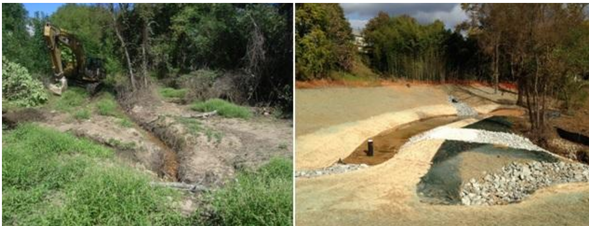
Figure 10: Harford County Water Quality Improvement Project - Before and After (Harford County Watershed Protection and Restoration Office)
