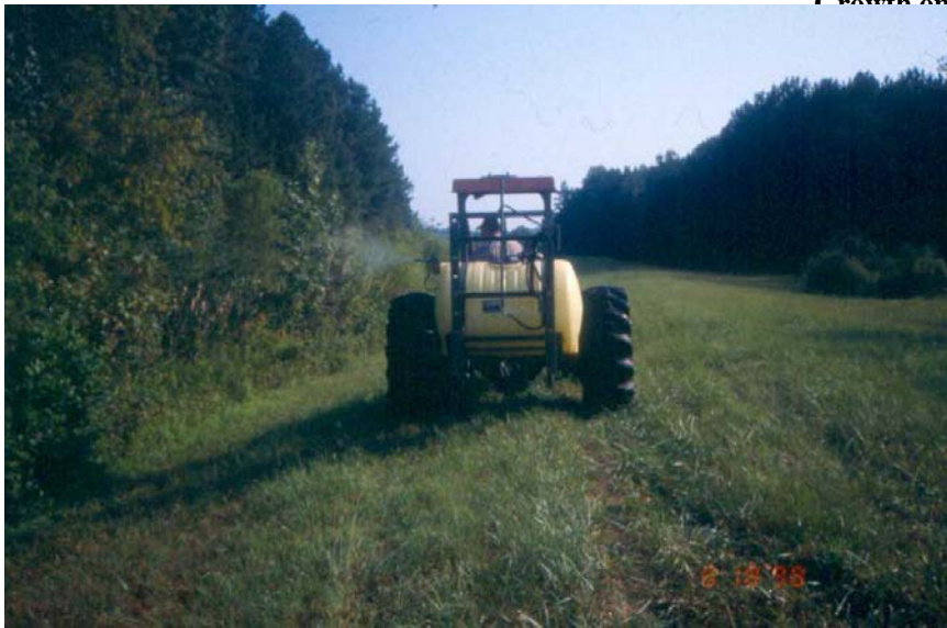
Figure 5f. Tractor spraying application on dam.
