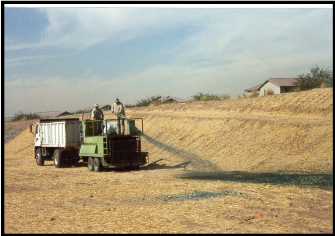
Figure 8. Hydro-seeding operations on a floodway dam in Maricopa County, Arizona (Renckly & Drake, 1999).
