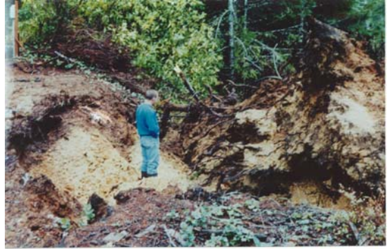
Figure 5. Serious damage by uprooted tree to embankment stability at a dam in Oregon.
