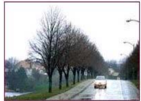
Figure 2. Example dam with problematic trees in Nebraska.
