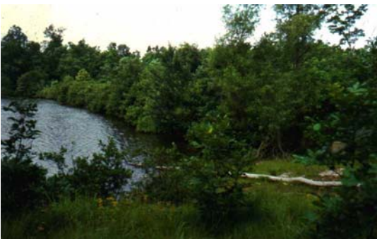
Figure 3. Example dam with inspection-hindering trees in Tennessee.
