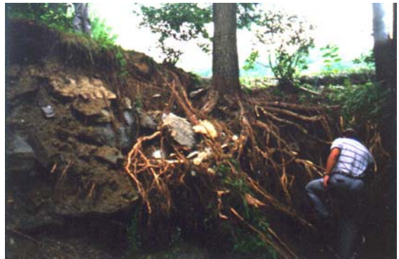
Figure 6. Tree root induced scouring on crest and downstream face of Coffey dam in Kansas.
