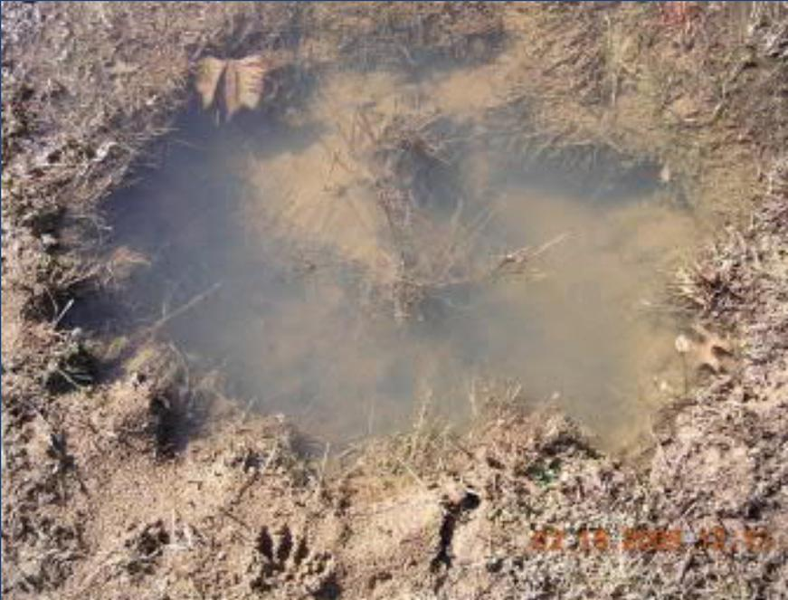
4-ft-diameter sand boil at downstream toe of dam
