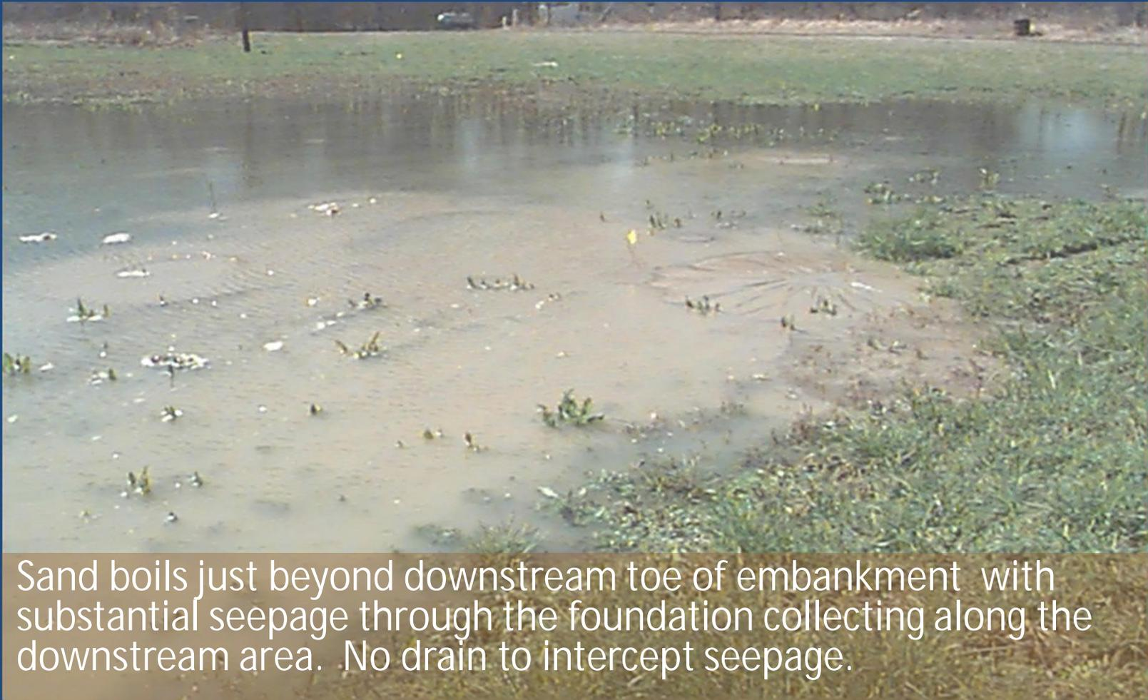
Sand boils just beyond downstream toe of embankment with substantial seepage through the foundation collecting along the downstream area. No drain to intercept seepage.
