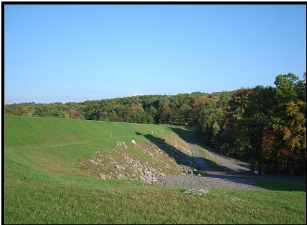
Deep Creek Lake Dam (Earthen)
