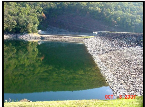
Savage River Dam (Rockfill)
