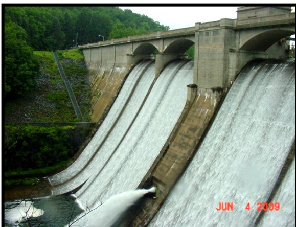
Prettyboy Dam (Concrete Gravity)
