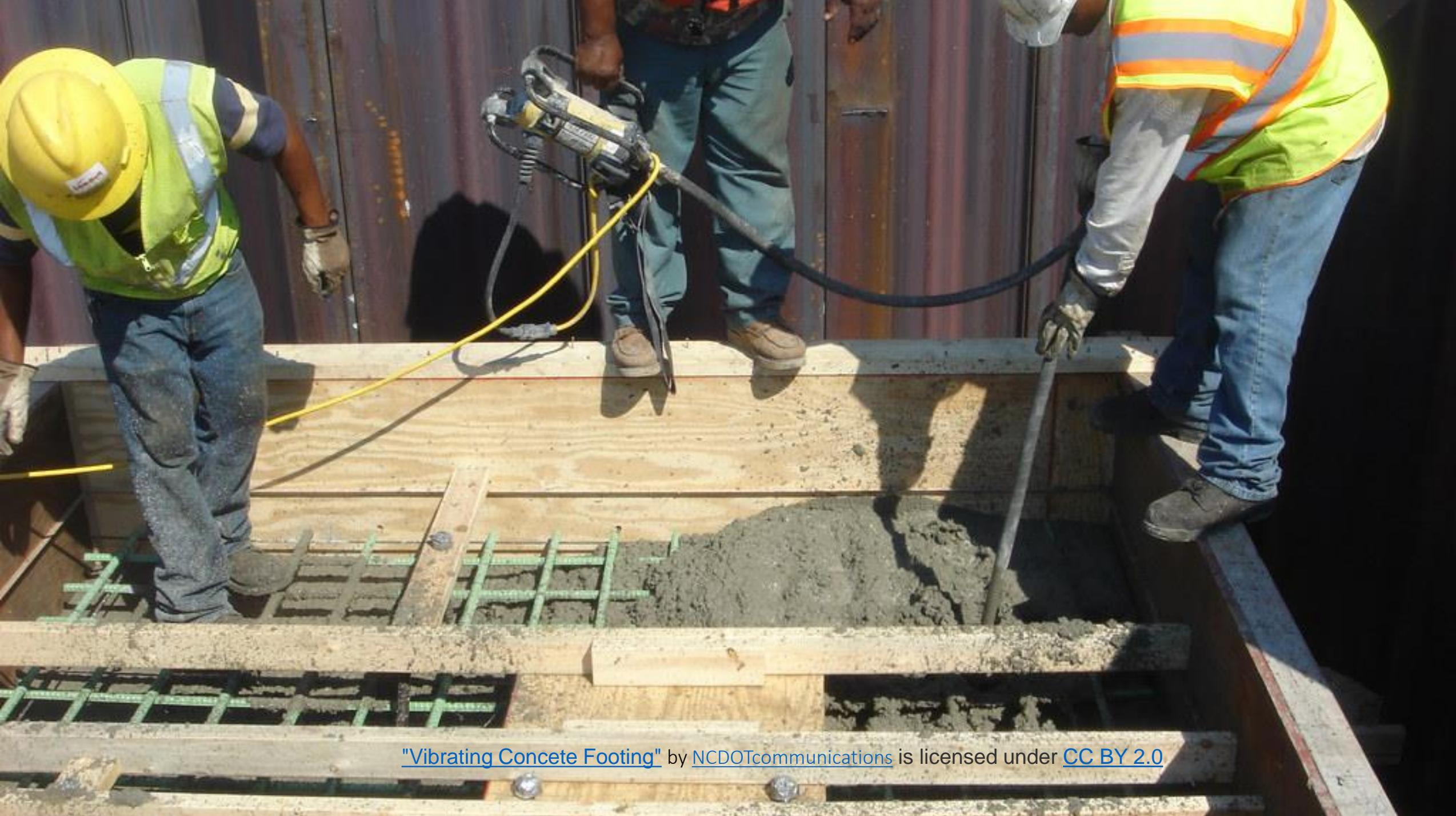
"Vibrating Concrete Footing" by [NCDOTcommunications](#) is licensed under [CC BY 2.0](#)
