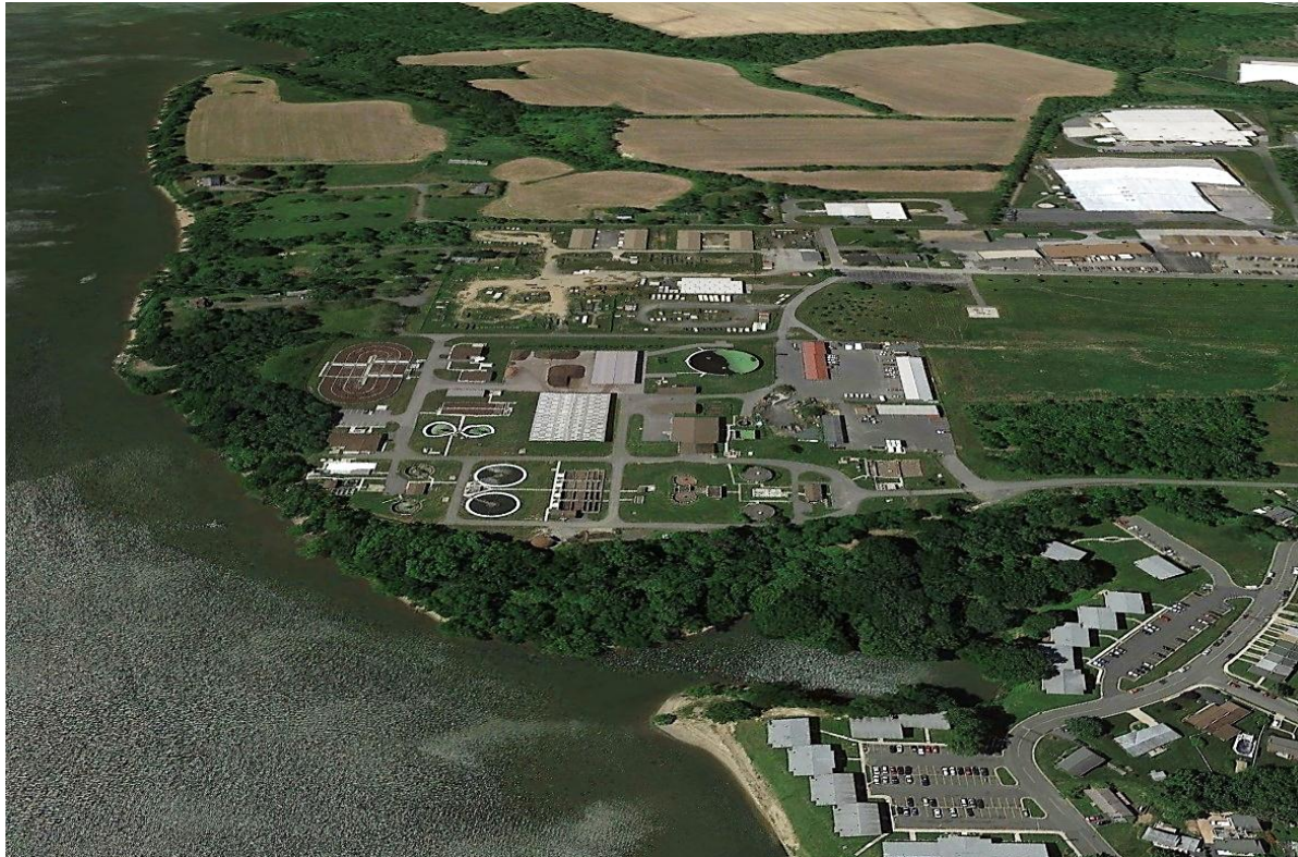
Figure 1 - Havre de Grace WWTP Source: Google Maps
