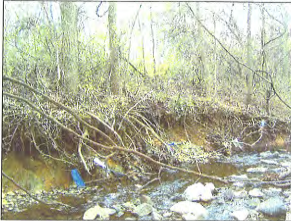
Bank erosion (Dec 2003)
