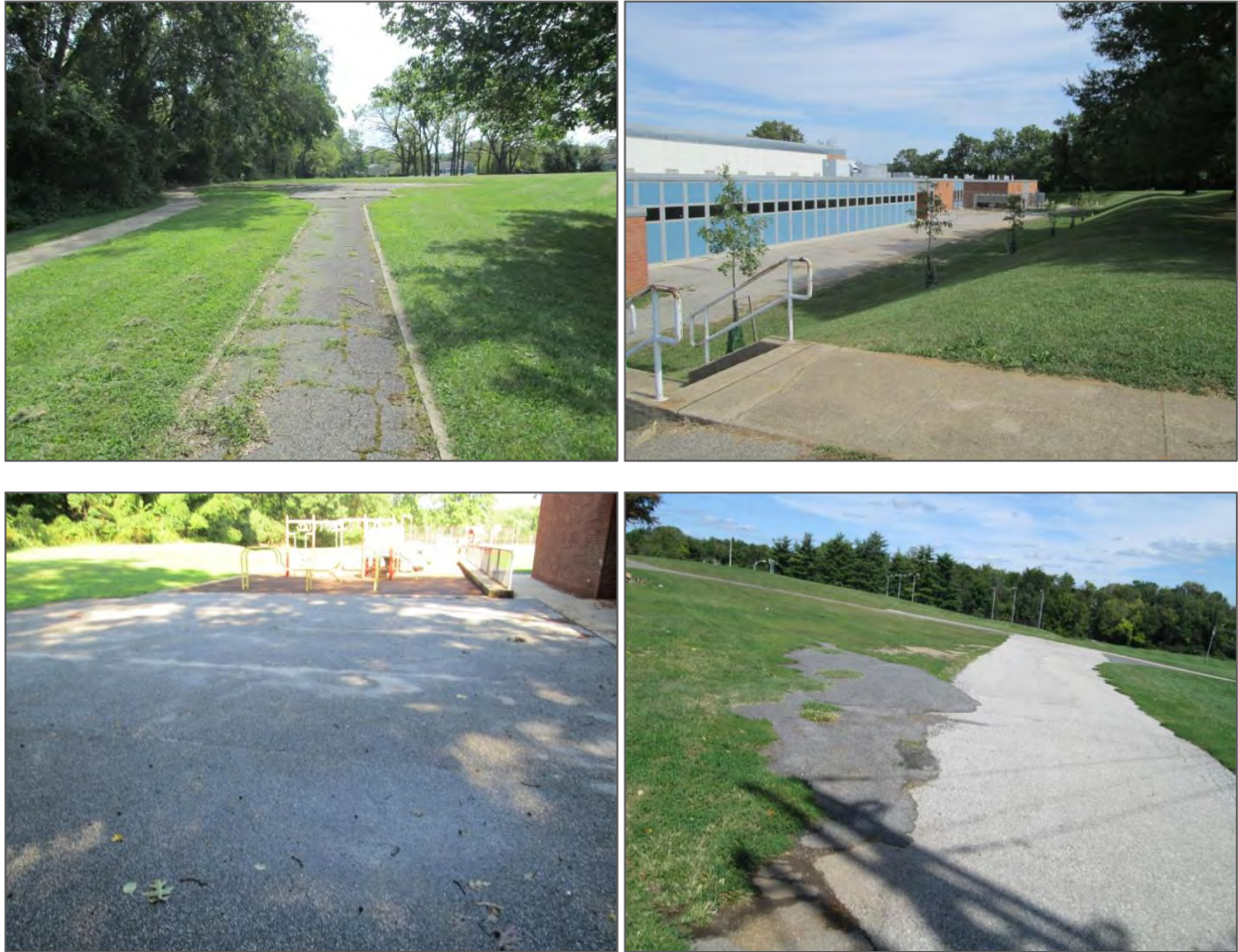
Figure 4-27: Extraneous Asphalt Cover Removal Opportunities at ISI_C_117 (top left and top right), ISI_C_202 (bottom left), and ISI_C_304 (bottom right)
