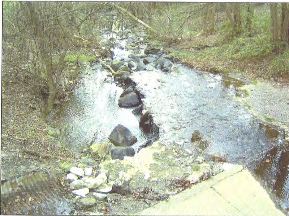
Looking downstream from the Patterson Ave. culvert (Dec. 2004)
