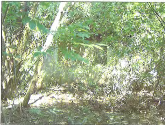
Looking downstream at headwall/riser (Summer 2003)
