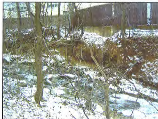
Erosion near parking lot
