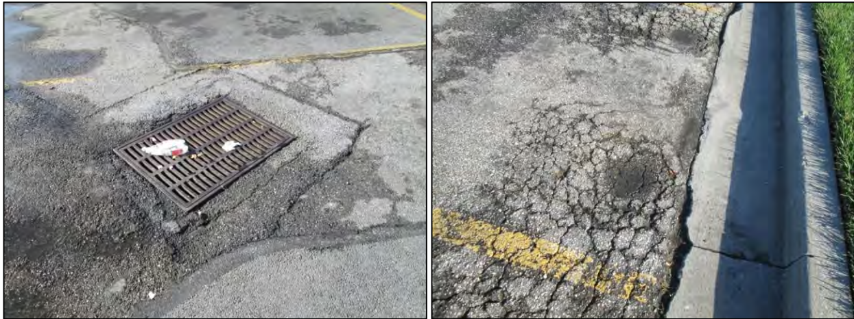
Figure 4-18: Degraded Impervious Surfaces at Commercial Hotspots
