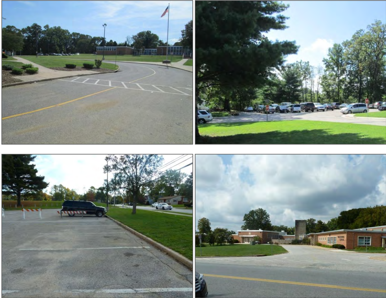
Figure 4-25: Parking Lot Retrofit Opportunities at ISI_C_117 (top left), ISI_C_202 (top right), ISI_C_306 (bottom left) and ISI_C_401 (bottom right)
