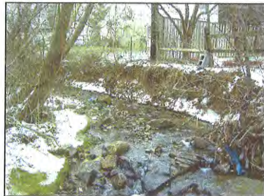
Bank erosion encroaching on a private fence
