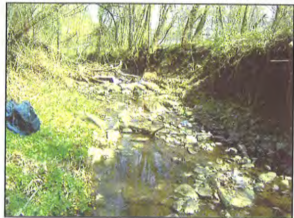
Typical bank erosion
