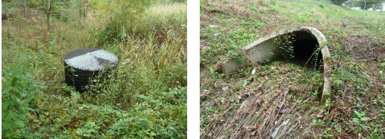
Figure -3-20: Outlet Structure (left) and Sediment at Inflow (right) at SWM_C_651
