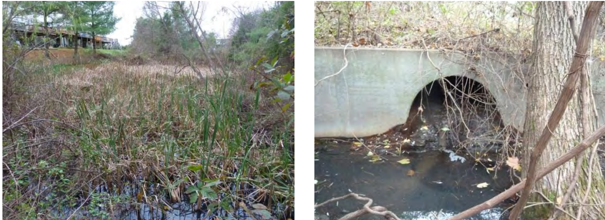
Figure-3-17: Invasive Species, Ponding (left) and Sediment Blocking the Downstream Outfall (right) at SWM_C_432
