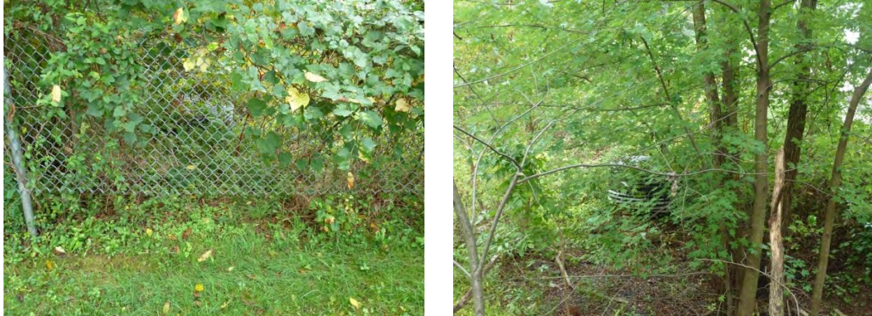
Figure-3-22: Fence Not Extended to Ground (left) and Vegetation Around Riser (right) at SWM_C_738
