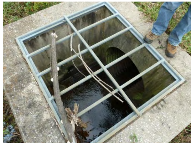
Figure-3-26: Undercutting and Erosion at Inflow Endsection (left) and Control Structure with Flowing Underdrains (right) at SWM_C_961
