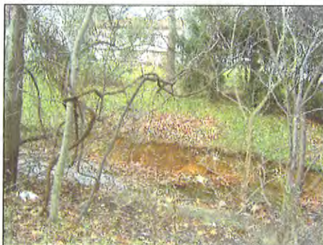
Bank erosion (December 2003)
