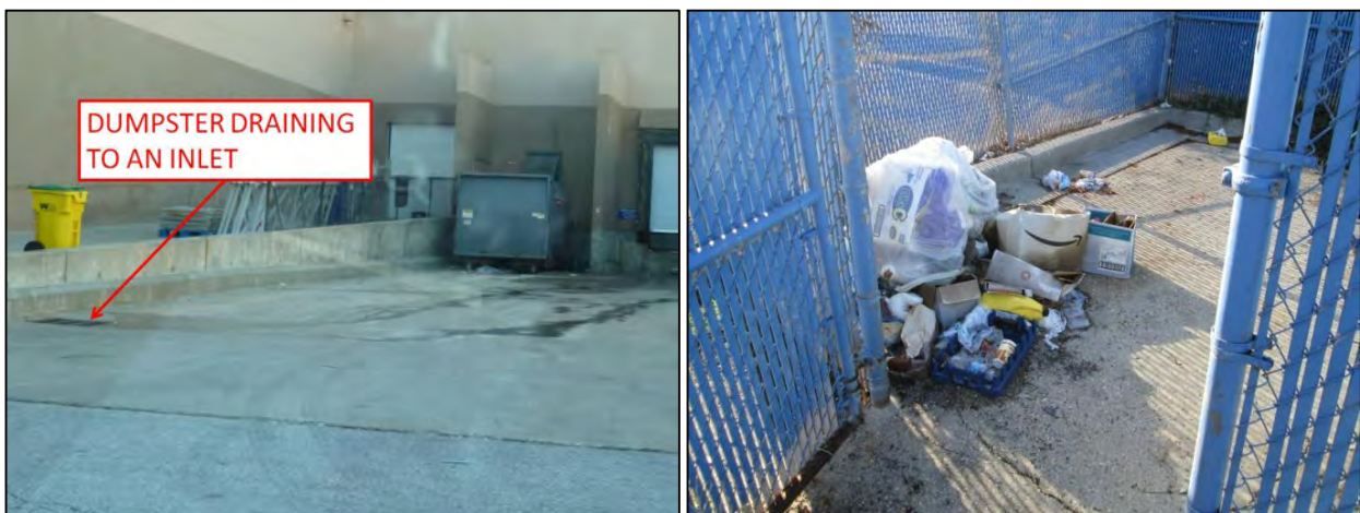
Figure 4-15: Leaking (left) and Overflowing Dumpsters (right) from Waste Management Operations at Commercial Hotspots
