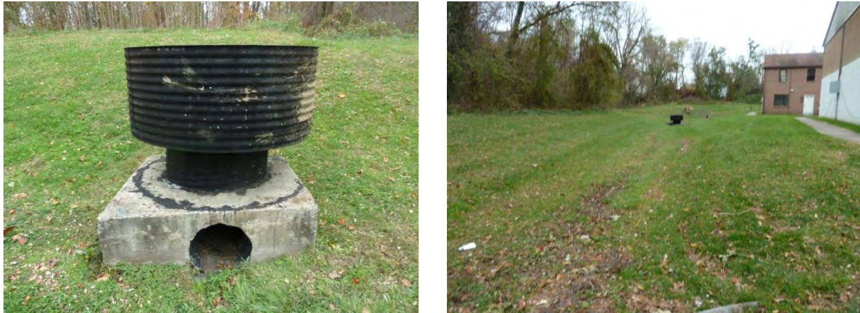
Figure-3-21: Riser with 18" Low Flow Pipe (left) and Grass Swale Leading to Riser (right) at SWM_C_715
