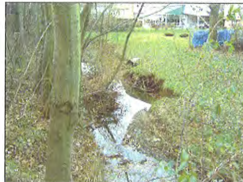
Bank erosion (December 2003)
