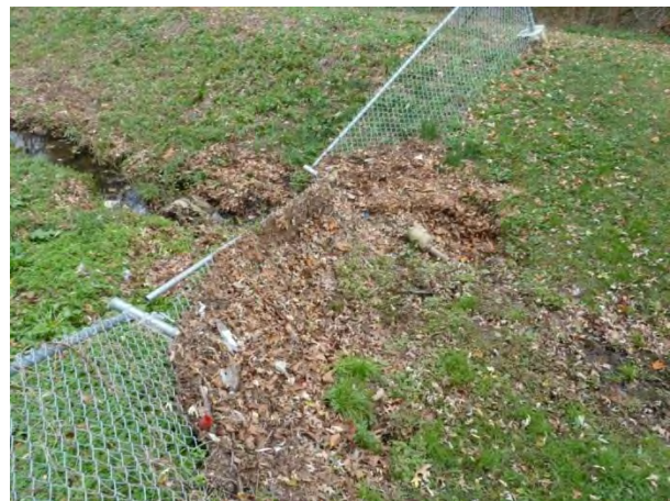
Figure 3-16: Channelized Grass Inflow (left) and Damaged Fence (right) at SWM_C_334
