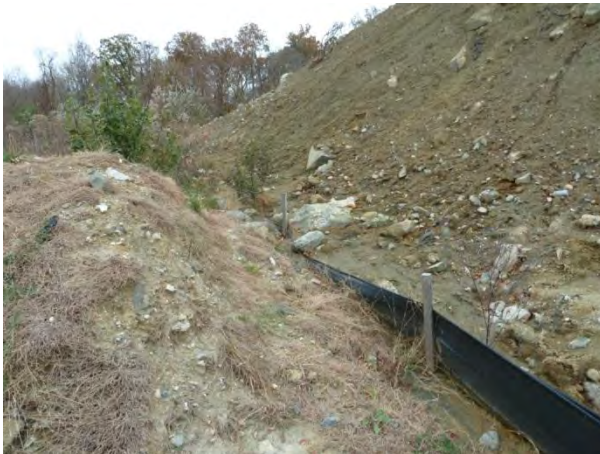
Figure-3-23: Sediment from Adjacent Stockpile Overtopping Silt Fence (left) and Dense Vegetation around Riser (right) at SWM_C_817
