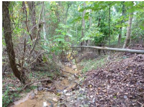
Figure-3-28: Down Tree Branches at Pond Outfall (left) and Low Flow Channel (right) at SWM_C_984
