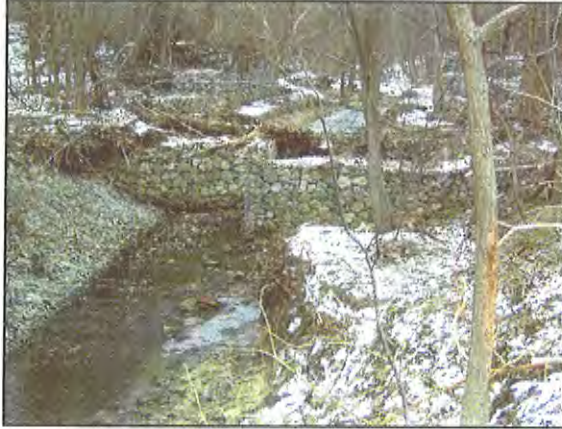
Energy dissipater dividing GFM-15-00-07 & -03
