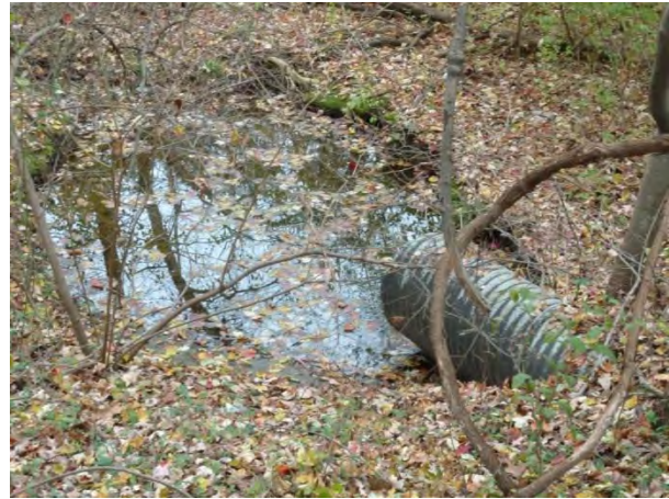
Figure-3-19: Side Slope Failure (left) and Erosion & Undercutting at Outfall (right) at SWM_C_450
