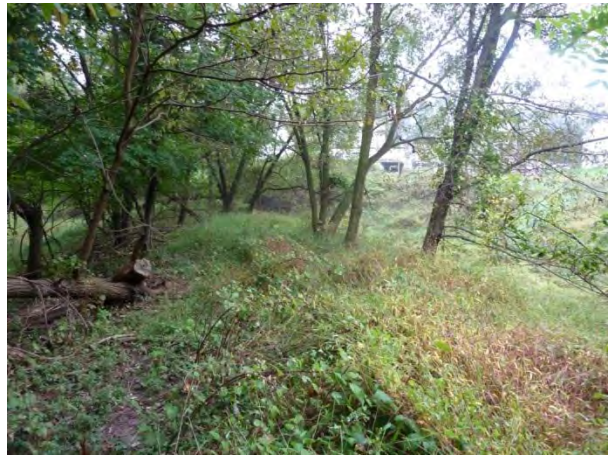
Figure-3-30: Animal Burrow (left) and Trees (right) on the Embankment at SWM_C_1652
