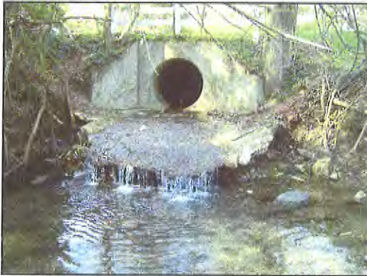
Outfall needing energy dissipater
