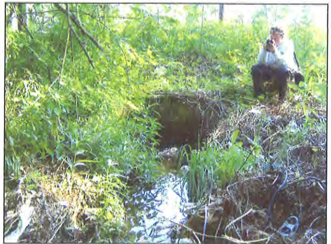
Looking U/S at headwall
