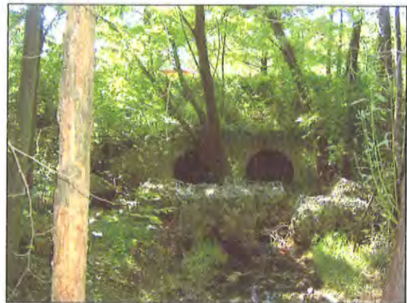
Looking upstream at outfall and failed dissipators (Summer 2003)
