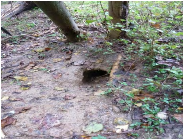
Figure-3-30: Animal Burrow (left) and Trees (right) on the Embankment at SWM_C_1652
