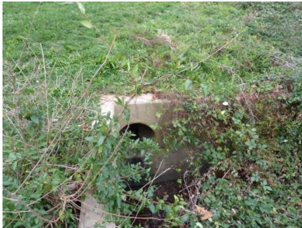
Figure-3-29: Pipe Invert at Inflow Endwall above Grade (left) and Wide Grass Swale Draining to Pond (right) at SWM_C_1188
