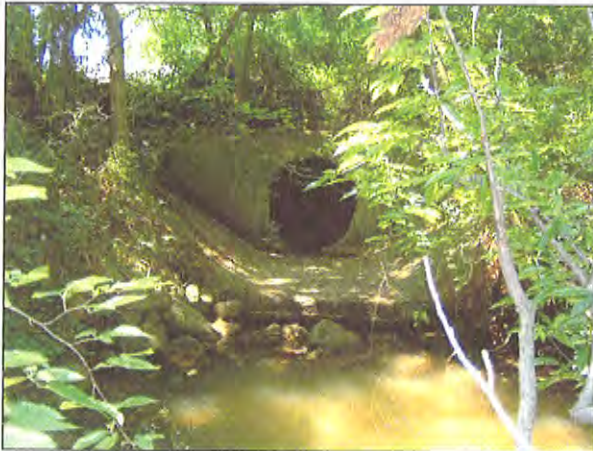
Looking upstream at outfall
