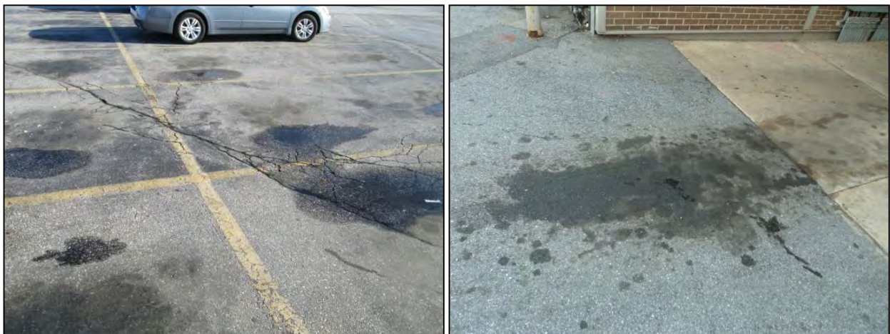
Figure 4-13: Asphalt staining from Outdoor Vehicle Operations at Auto-related Hotspots.
