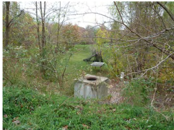
Figure-3-25: Pond Embankment (left) and Control Structure with Missing Lid (right) at Detention Pond SWM_C_859
