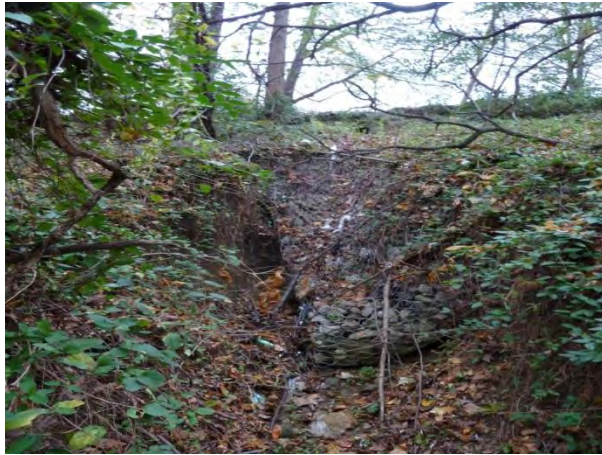
Figure-3-19: Side Slope Failure (left) and Erosion & Undercutting at Outfall (right) at SWM_C_450
