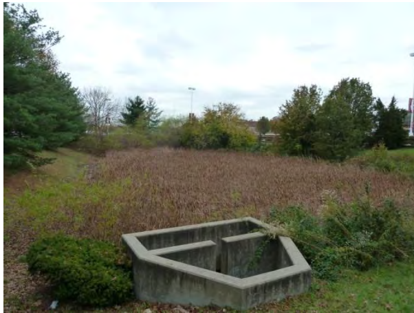
Figure-3-24: Dense Invasive Vegetation Around the Outlet Structure (left) and Curb Cut Inlet Configuration (right) Draining to SWM_C_857
