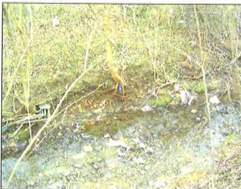
Bank erosion in December 2003.
