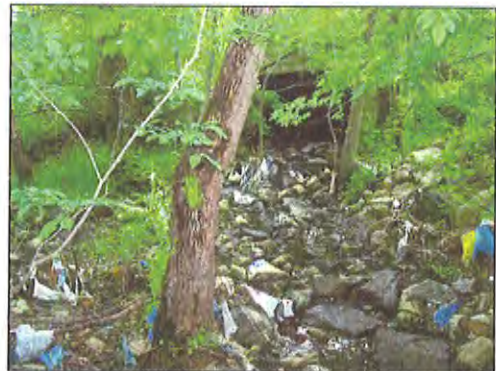
Looking upstream at outfall for project , May 2004
