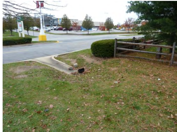
Figure-3-24: Dense Invasive Vegetation Around the Outlet Structure (left) and Curb Cut Inlet Configuration (right) Draining to SWM_C_857
