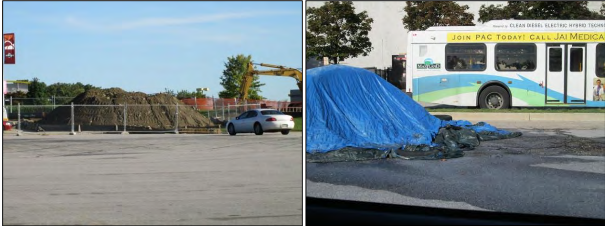
Figure 4-19: Soil Stockpile (left) and Leaking Stockpile Area (right) at Construction Hotspots
