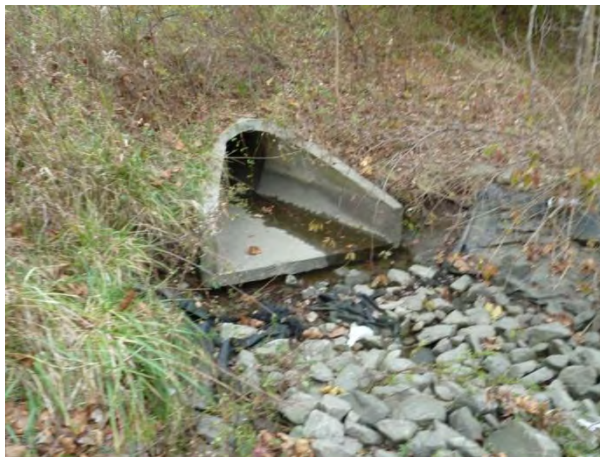
Figure-3-26: Undercutting and Erosion at Inflow Endsection (left) and Control Structure with Flowing Underdrains (right) at SWM_C_961
