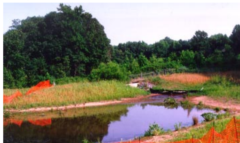
Stormwater management ponds are the standard answer for stormwater control. Yet, the outfall from this pond has helped to create large gulleys and other erosion problems in the area of Cuckold Creek.
