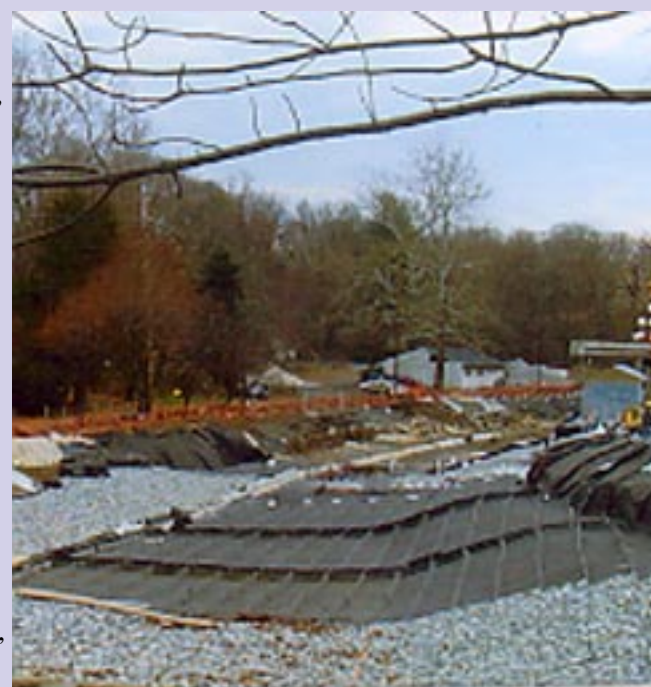
The site during the construction of the protective layer.
