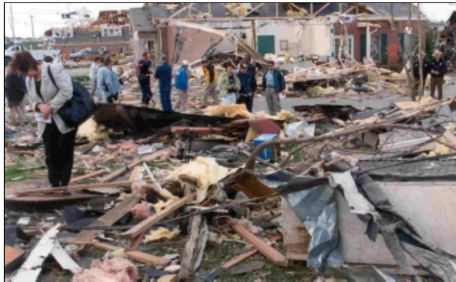
Above, state and local officials join residents in looking at the remains of La Plata's Main Street business and residential area after the town was hit by an F-5 tornado on April 28. At right, a wind-toppled water tower drained about 600,000 gallons from the county's water supply.
