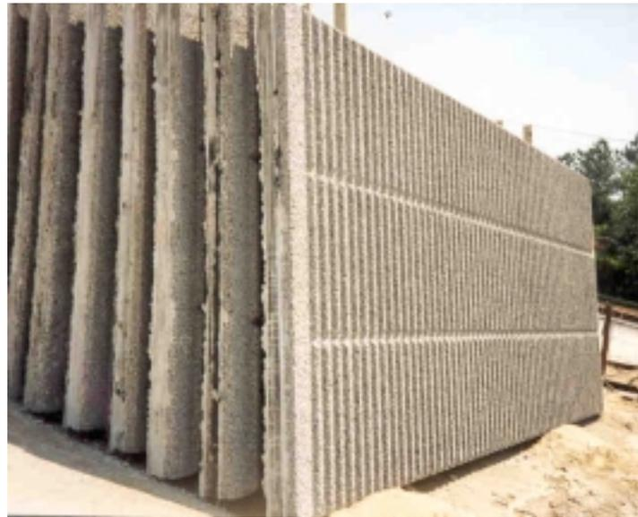
Individual concrete and scrap tire soundwall panels ready for installation.
