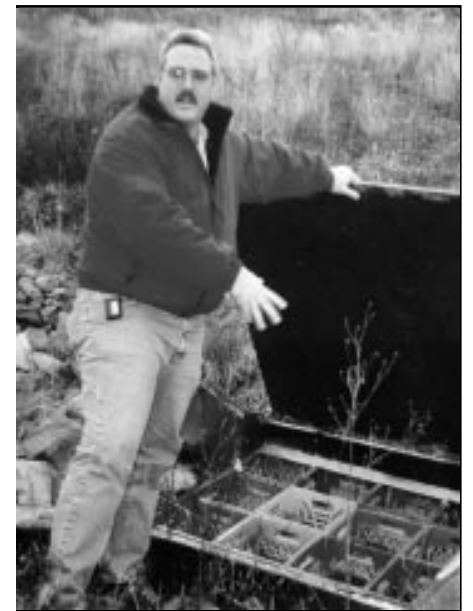
Hand-made innovations by Jim Keithley (pictured above), manager of the the Cecil County Central Landfill, and his staff, include using milk crates and photofloc gel logs to help filter sediment before it enters Northeast Creek.
