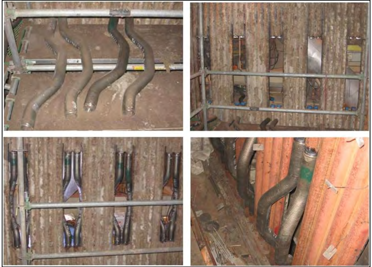
Figure 4. Waterwall Tube Modifications for Tertiary Air Nozzles
