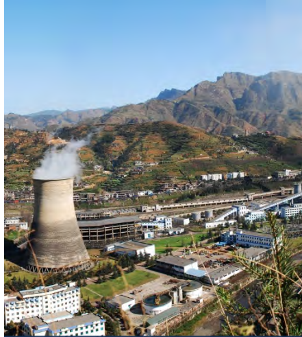
Yixing Power, Jiangsu
