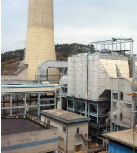
Shajiao Power Plant, Shenzhen
