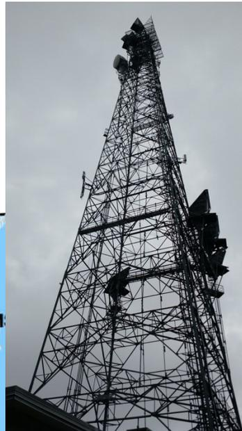
Towers clustered in the Baltimore/Washington area - measure methane and CO<sub>2</sub> continuously
